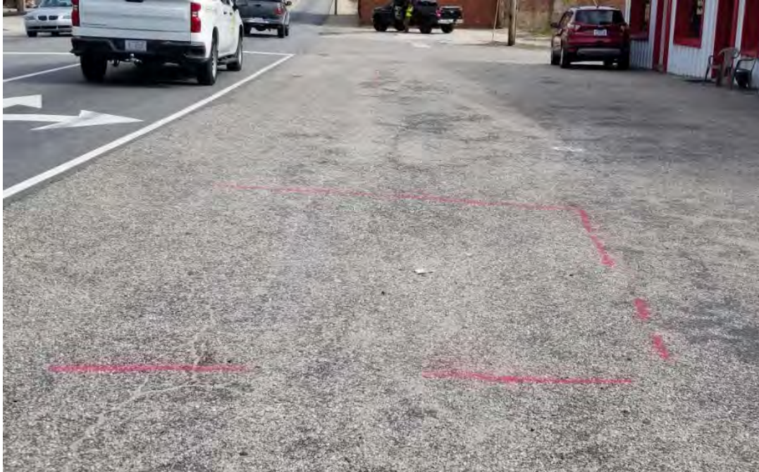
Photograph 1. Parcel 005 non-metallic GPR anomaly.
