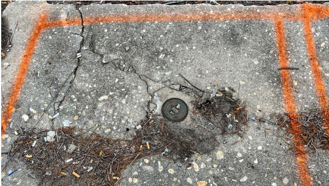
Photograph 2. Fill port visible at the surface.
