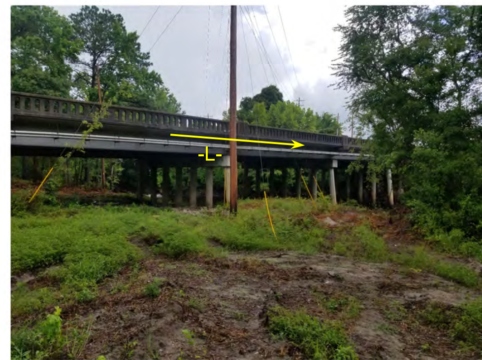
DOWNSTREAM (RIGHT) OF -L- FACING NORTH
