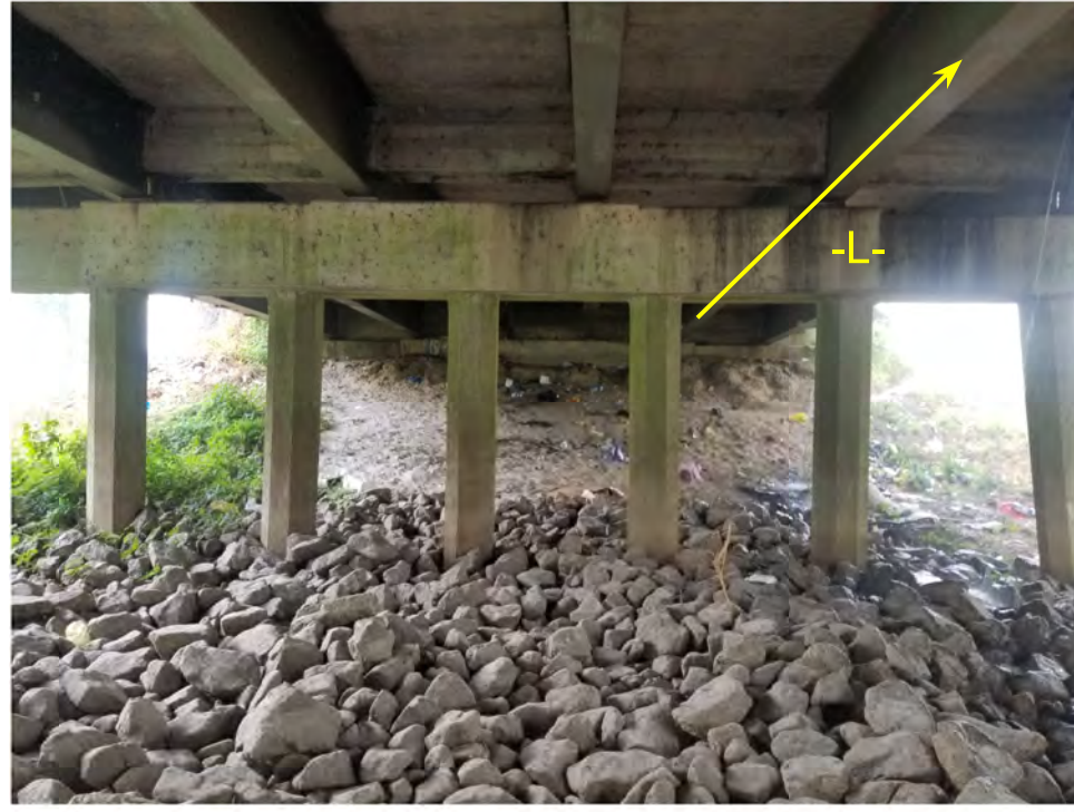
NEAR BENT 1 FACING WEST TO END BENT 1
