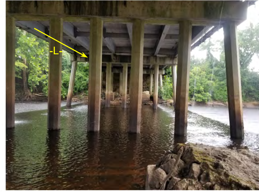
NEAR BENT 1 FACING EAST TO END BENT 2
