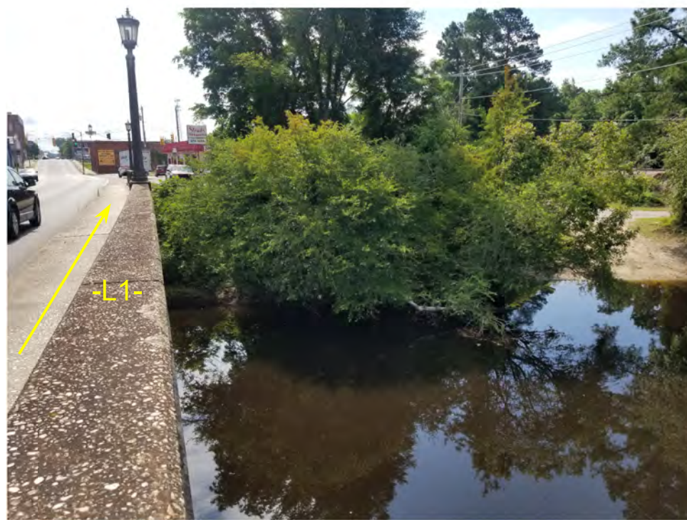
RIGHT OF -L1- NEAR BENT 2 FACING EAST TOWARDS END BENT 2
