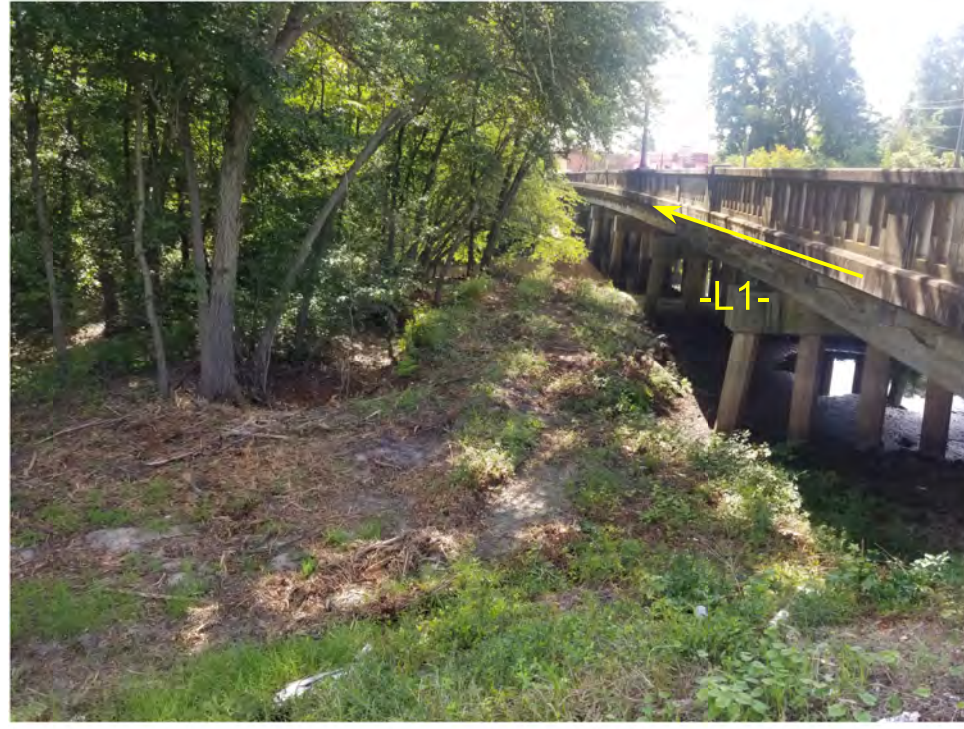
LEFT OF -L1- NEAR END BENT 1 FACING EAST
