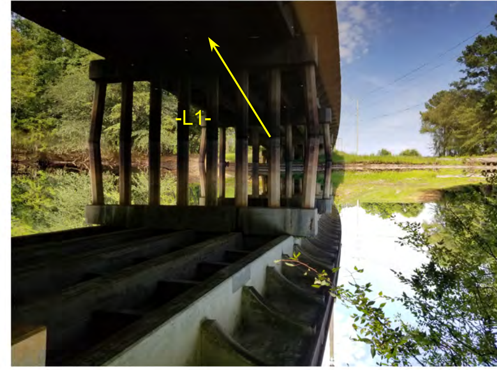
LEFT OF -L1- NEAR BENT 2 FACING WEST TOWARDS END BENT 1
