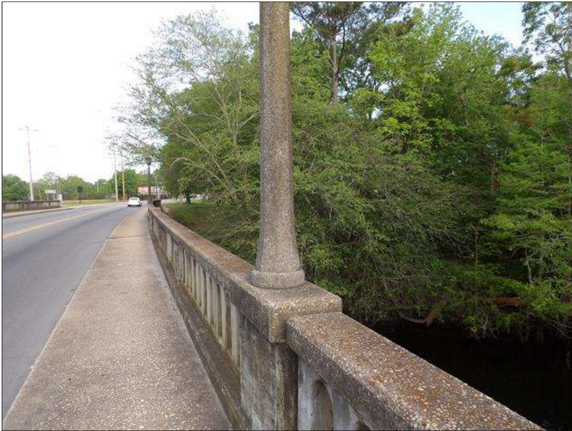
Typical light post attached to rails, left rail shown
