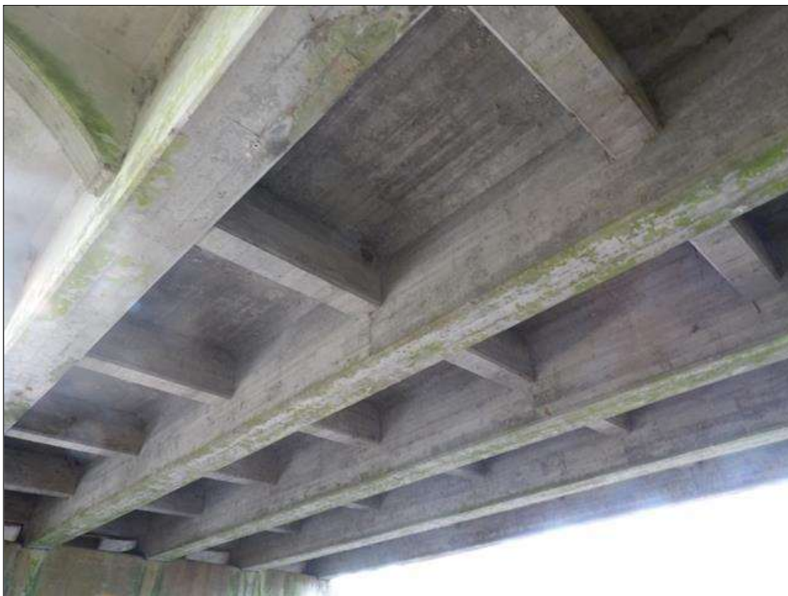
Superstructure underside, Span 3 shown, all others similar
