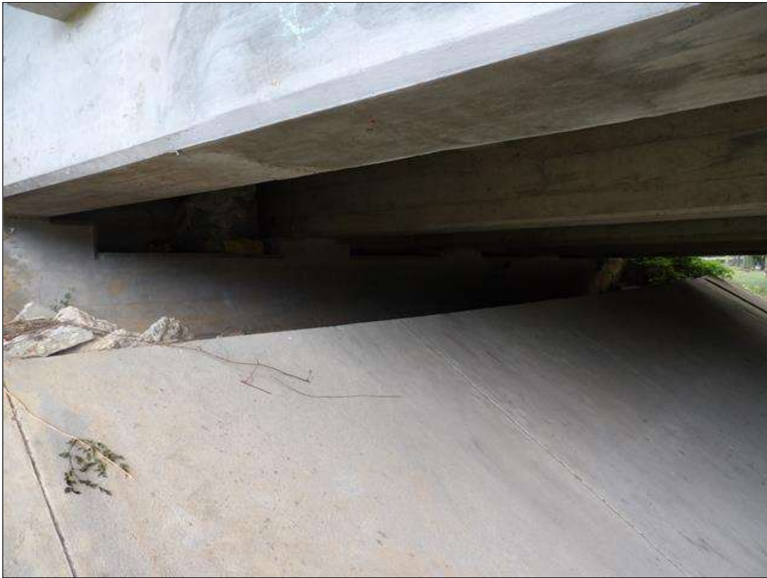
Abutment 1, Abutment 2 similar
