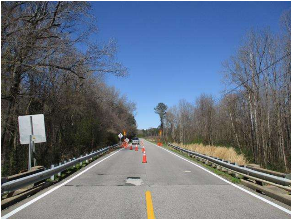
GUIDERAIL LOOKING NORTH
