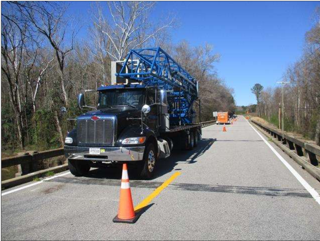
HYDRAPLATFORM AND TRAFFIC CONTROL USED DURING INSPECTION
