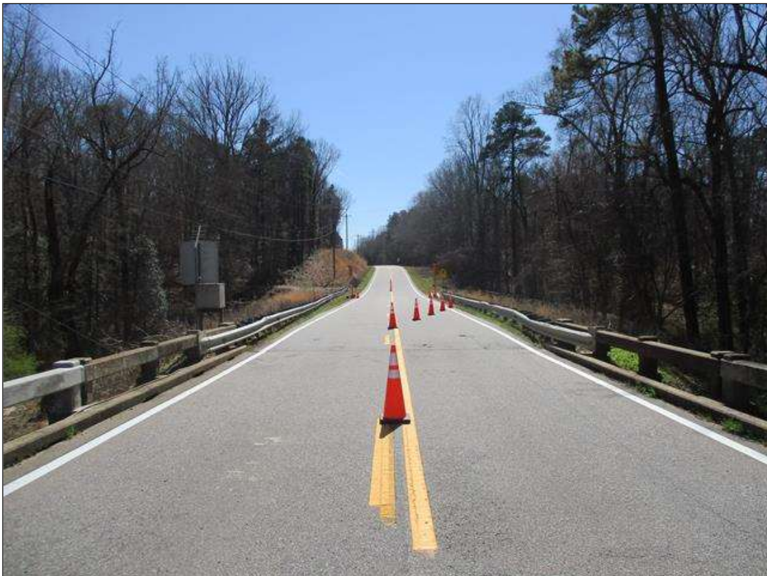
GUIDERAIL LOOKING SOUTH
