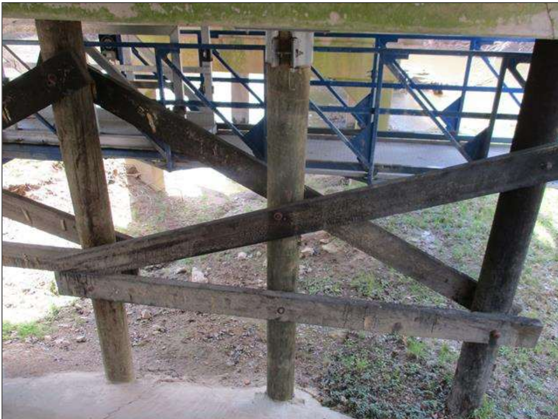
Bent 9 Pile 2: [NEW REPAIR] PILE SPLICED USING STEEL COLLARS [APPROXIMATELY 12' LONG]
