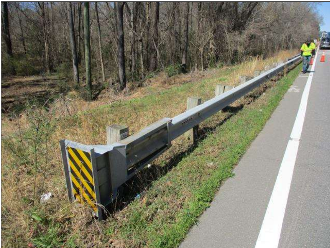
TYPICAL GUIDERAIL END
