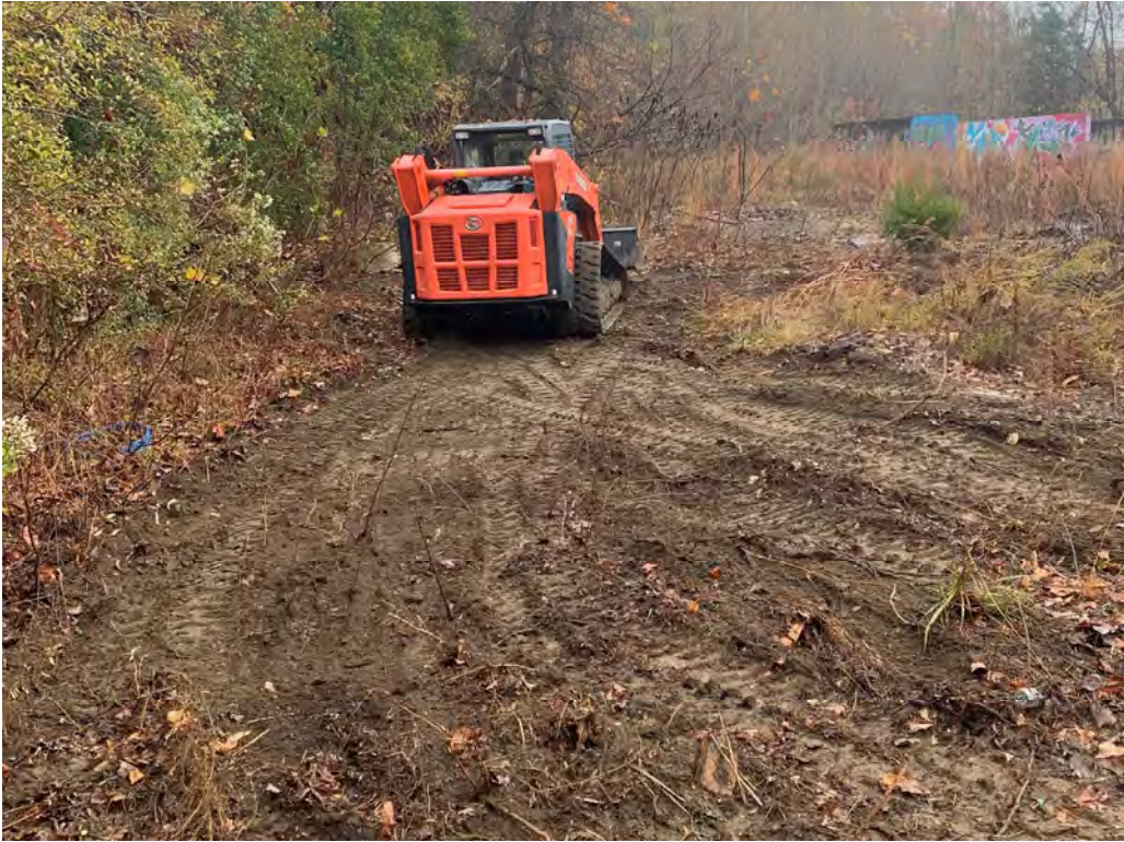
Photograph 3 – Photo of investigation area being cleared.
