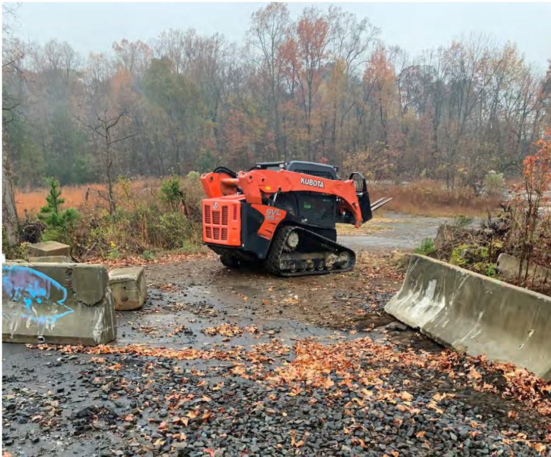
Photograph 2 – View of barricade being moved to gain access to site.
