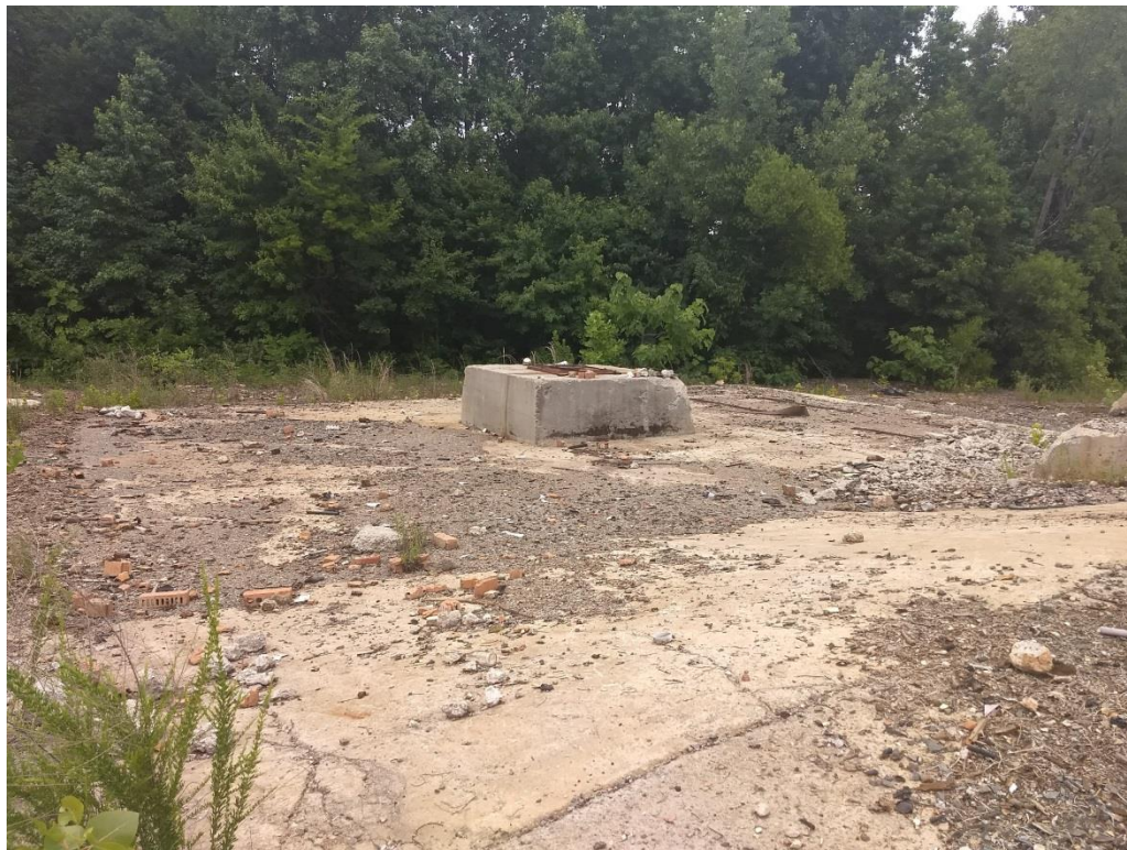
C. Photo from central portion of site showing typical building debris.
