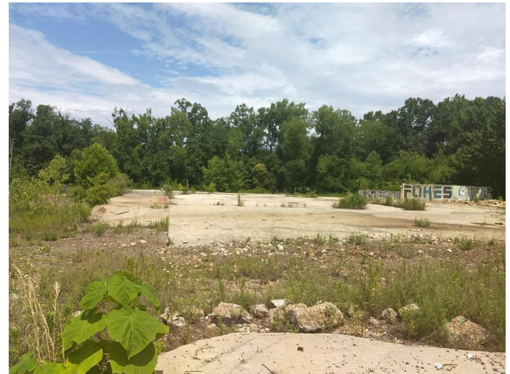
D. Photo from central portion of site showing typical building debris..
