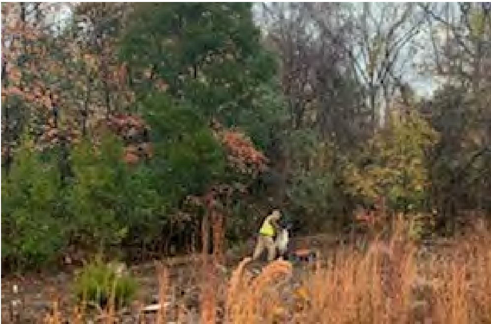
Photograph 4 – Photo of private utilities being located.
