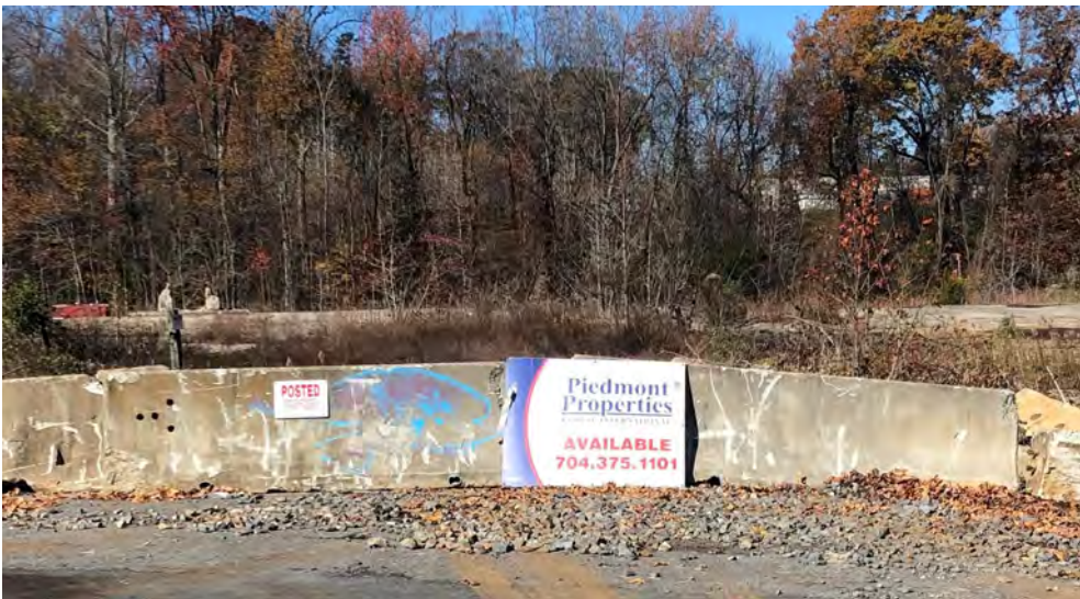
Photograph 6 – Photo of replaced barricade wall after investigation activities.
