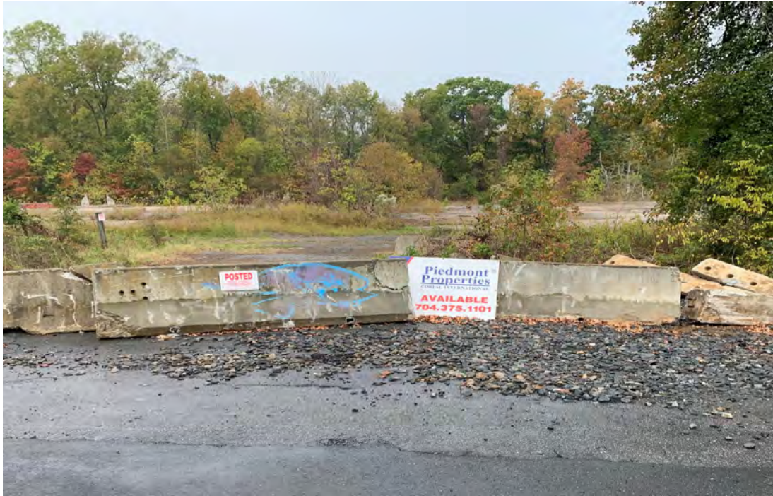
Photograph 1 – View of site entrance barricade prior to investigation activities.
