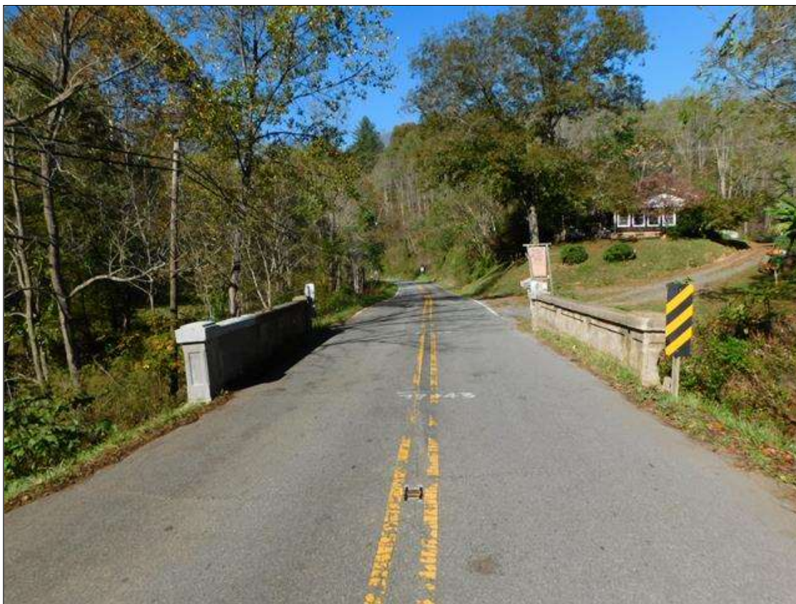
SOUTH APPROACH LOOKING NORTH
