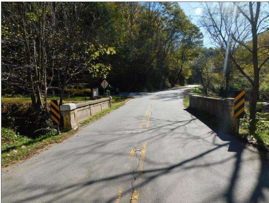
NORTH APPROACH LOOKING SOUTH
