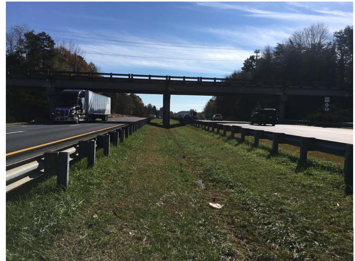
BENT 1, LOOKING FROM RT TO LT.
