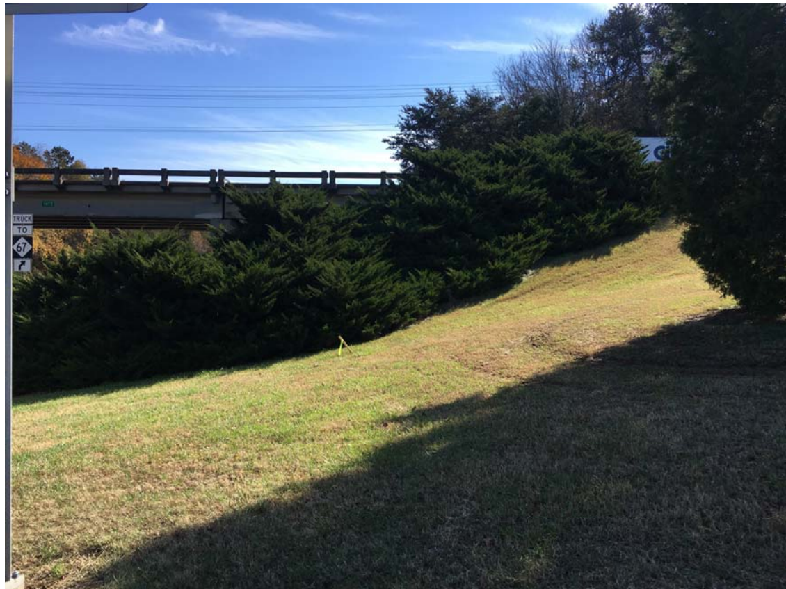
END BENT 1, LOOKING FROM LT TO RT.
