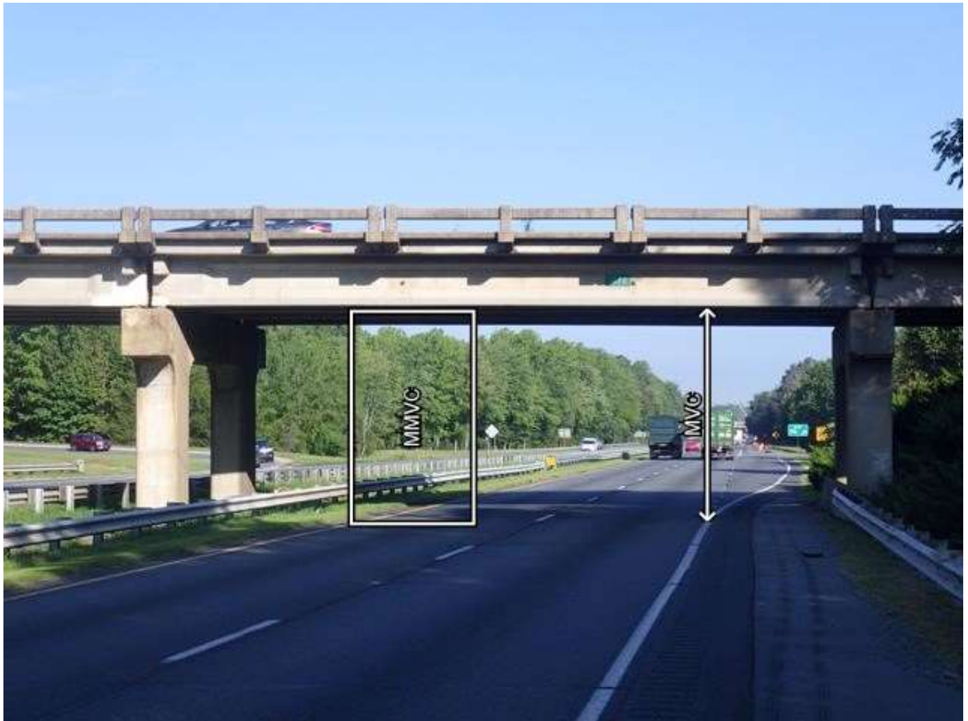
SPAN 3 SOUTH ELEVATION (LOOKING NORTH)
