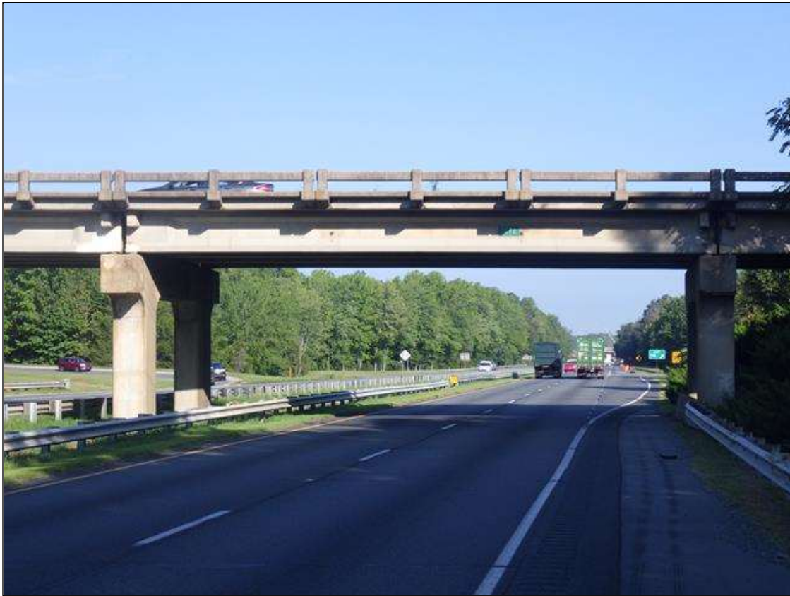
SPAN 3 SOUTH ELEVATION (LOOKING NORTH)
