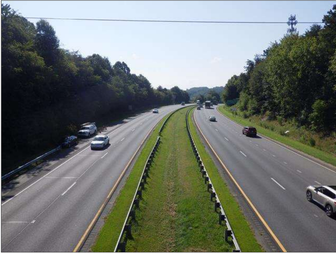
LOOKING SOUTH ALONG US52
