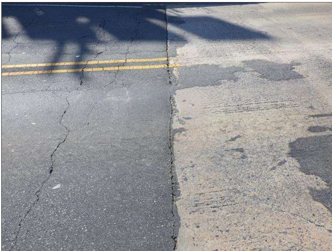
EAST APPROACH TRANSITION AT END BENT 2
