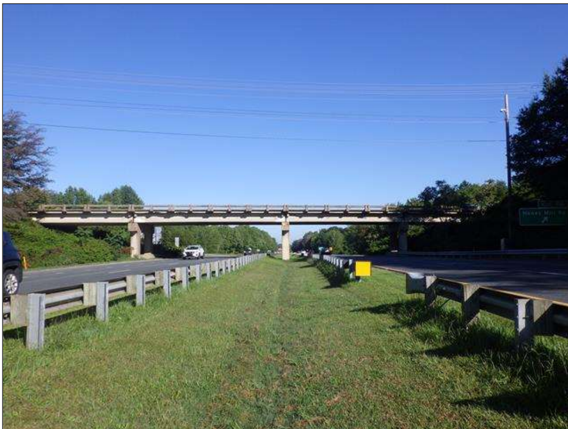
SOUTH ELEVATION LOOKING NORTH
