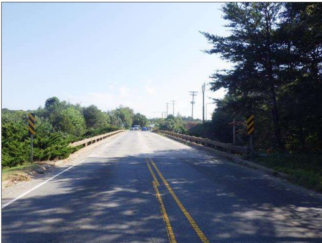
WEST APPROACH LOOKING EAST
