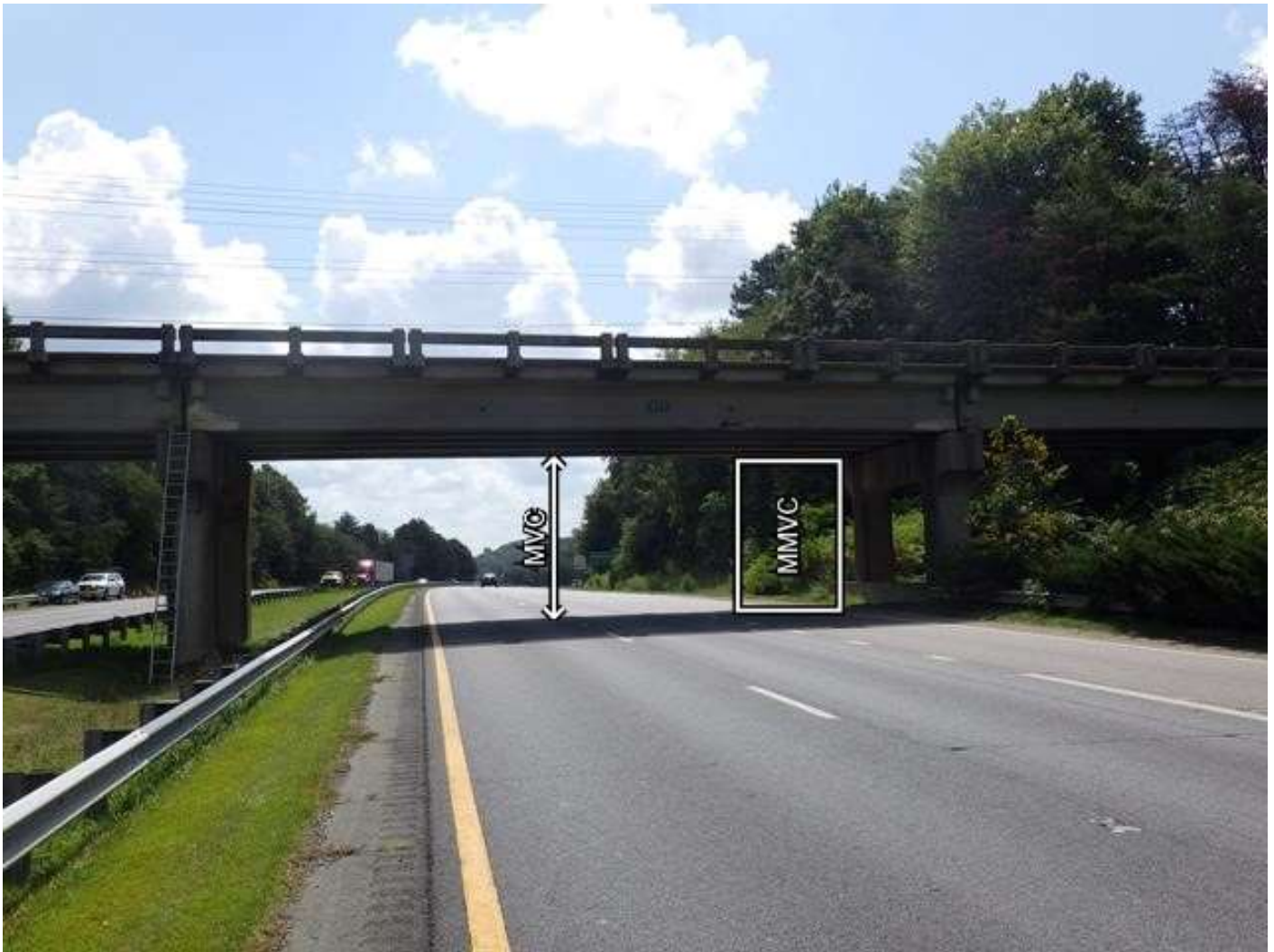
SPAN 2 NORTH ELEVATION (LOOKING SOUTH)
