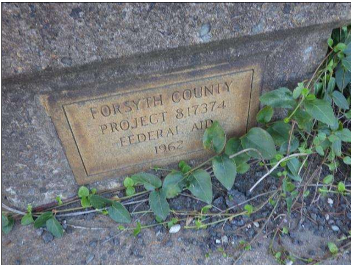
SOUTHWEST BRIDGE PLAQUE (NORTHEAST SIMILAR)
