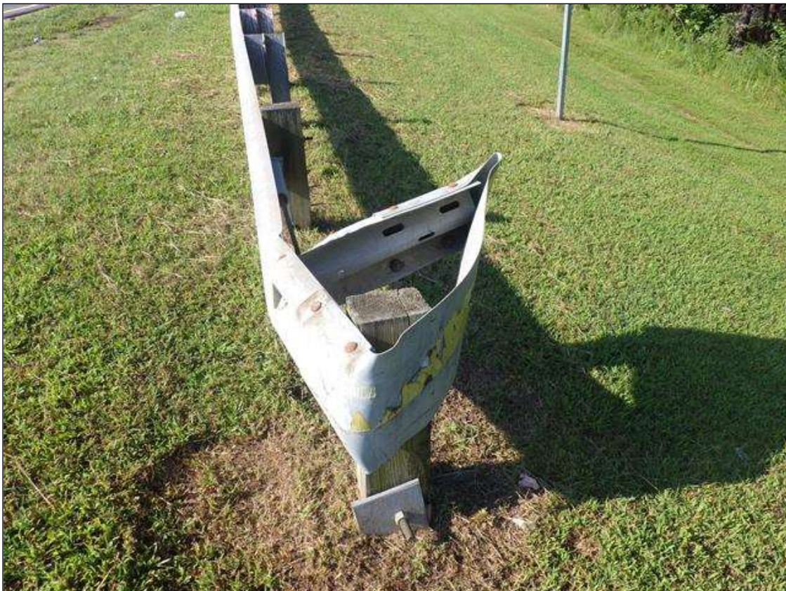
NORTHEAST GUARDRAIL END TREATMENT
