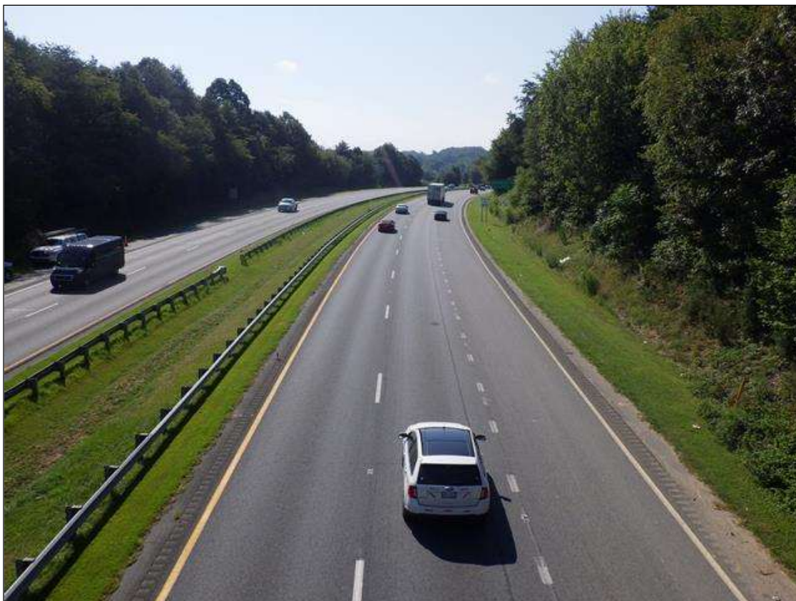
LOOKING SOUTH ALONG US52 SOUTHBOUND LANES FROM SPAN 2
