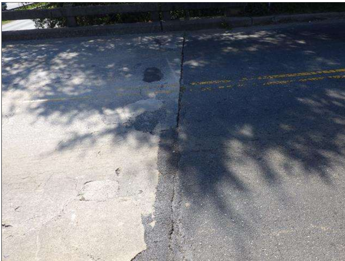
WEST APPROACH TO END BENT 1 TRANSITION
