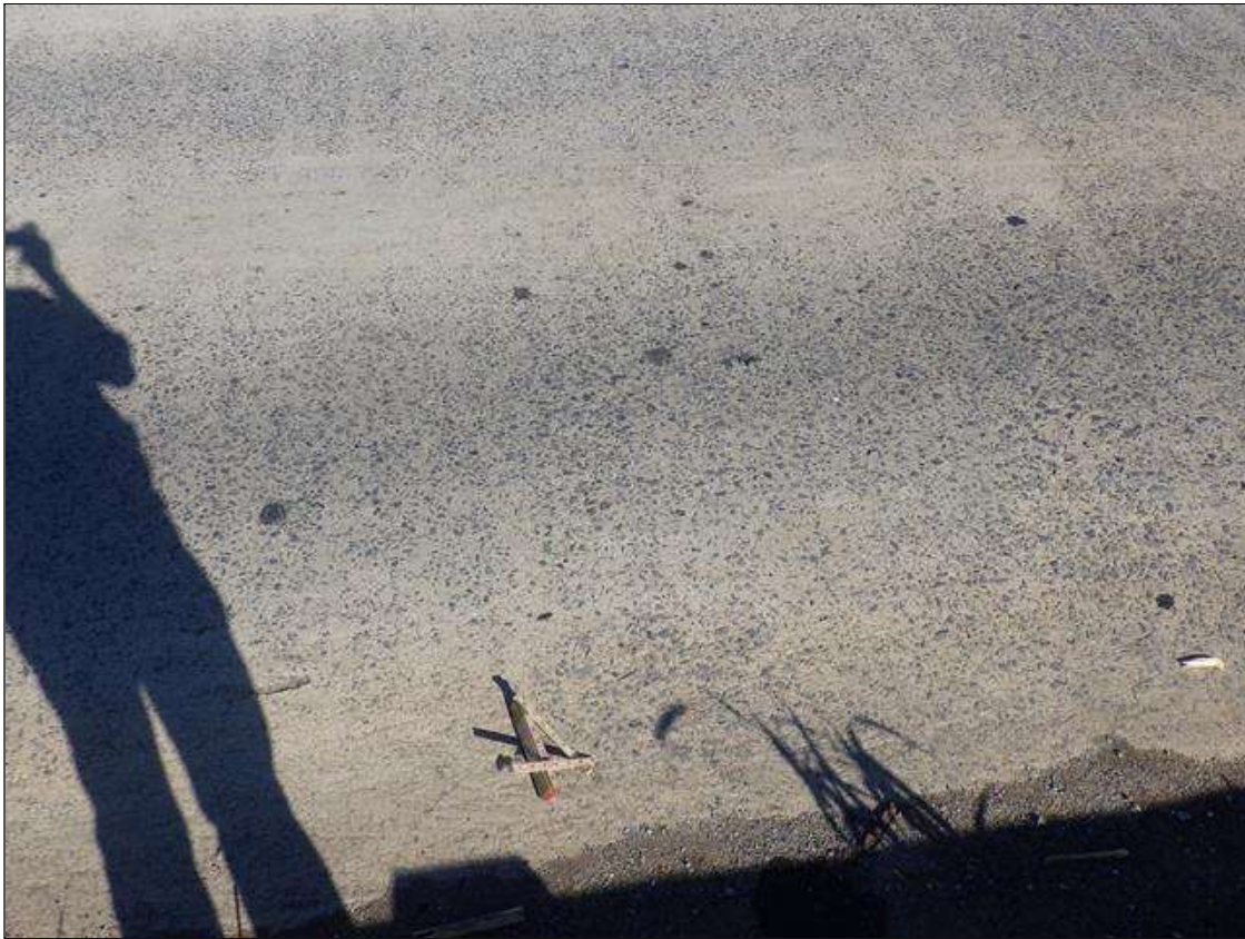
SPAN 3 CONCRETE DECK (OTHER SPANS SIMILAR)
