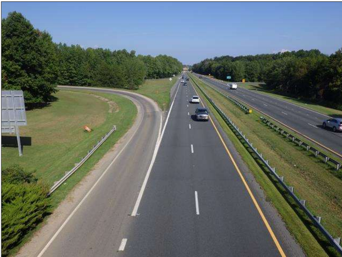
LOOKING NORTH ALONG US52 SOUTHBOUND LANES FROM SPAN 2
