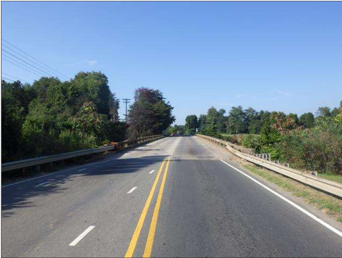
EAST APPROACH LOOKING WEST
