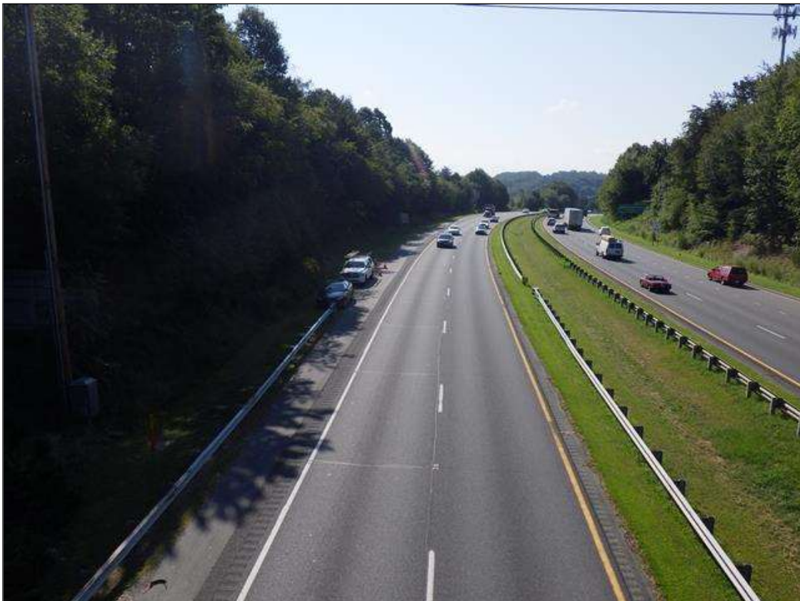
LOOKING SOUTH ALONG US52 NORTHBOUND LANES FROM SPAN 3
