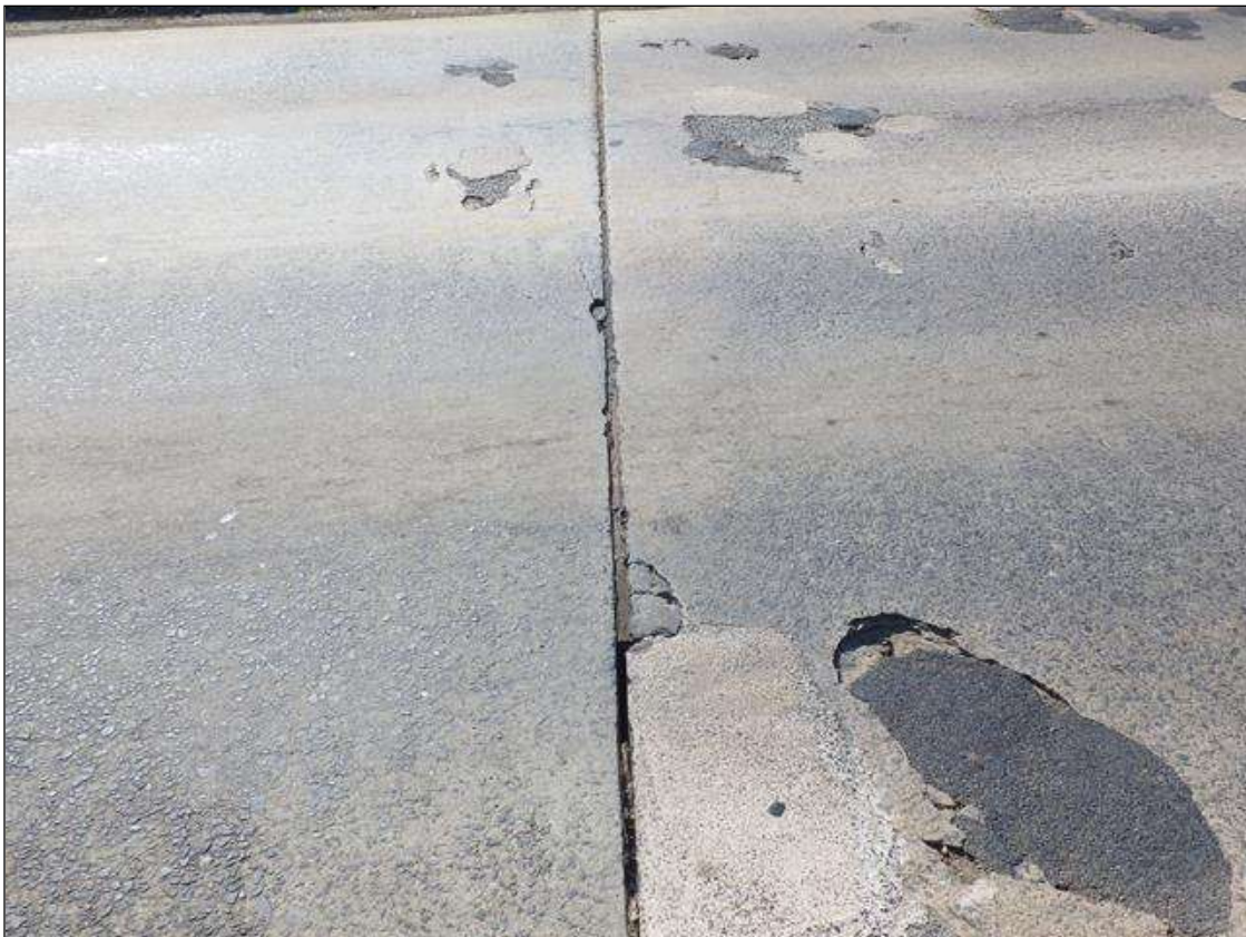
JOINT AT BENT 2
