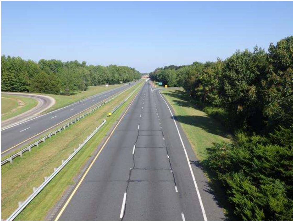
LOOKING NORTH ALONG US52 NORTHBOUND LANES FROM SPAN 3
