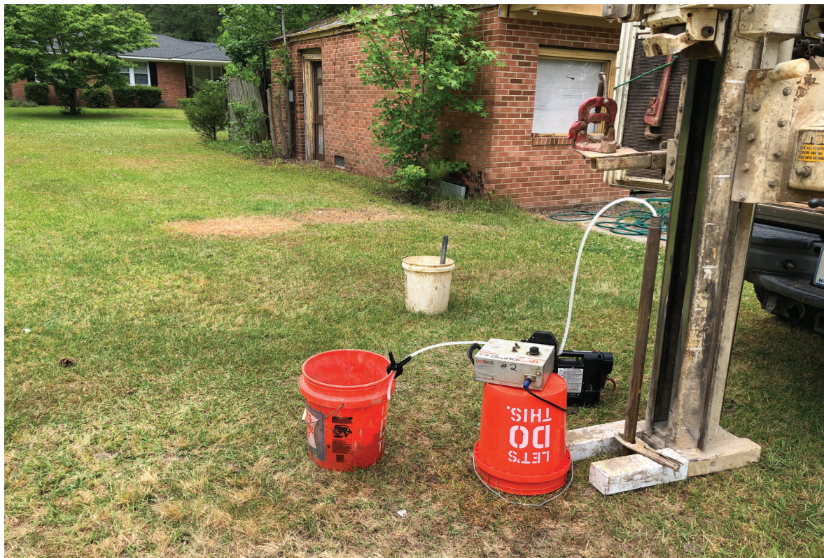
PHOTOGRAPH 2. Location of SB-2, no photograph of SB-3..
