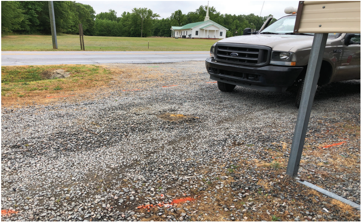
PHOTOGRAPH 3. Location of SB-3.
