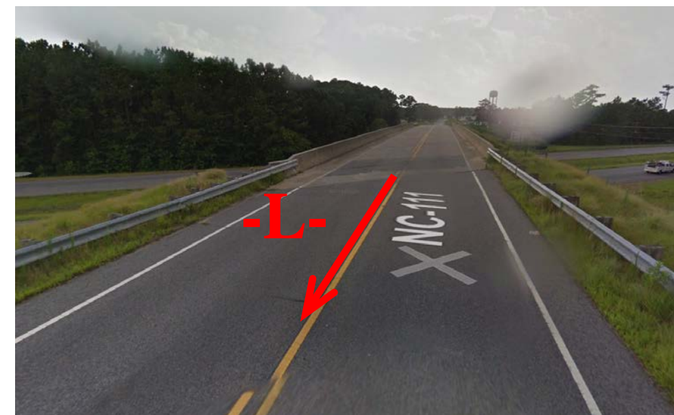
Standing on NC 111 (W. Wilson St.) looking southwest toward End Bent 2
