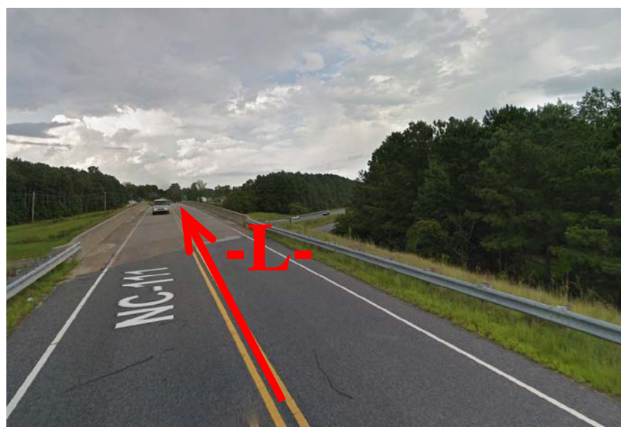
Standing on NC 111 (W. Wilson St.) looking northeast toward End Bent 1
