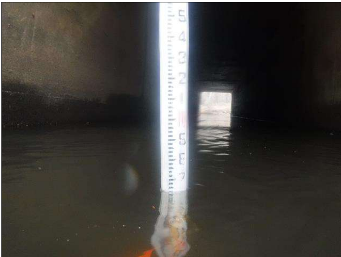
Span 1 Culvert Section 1: UPSTREAM CURTAIN WALL EXPOSURE 2.2' VERT (PAR)
