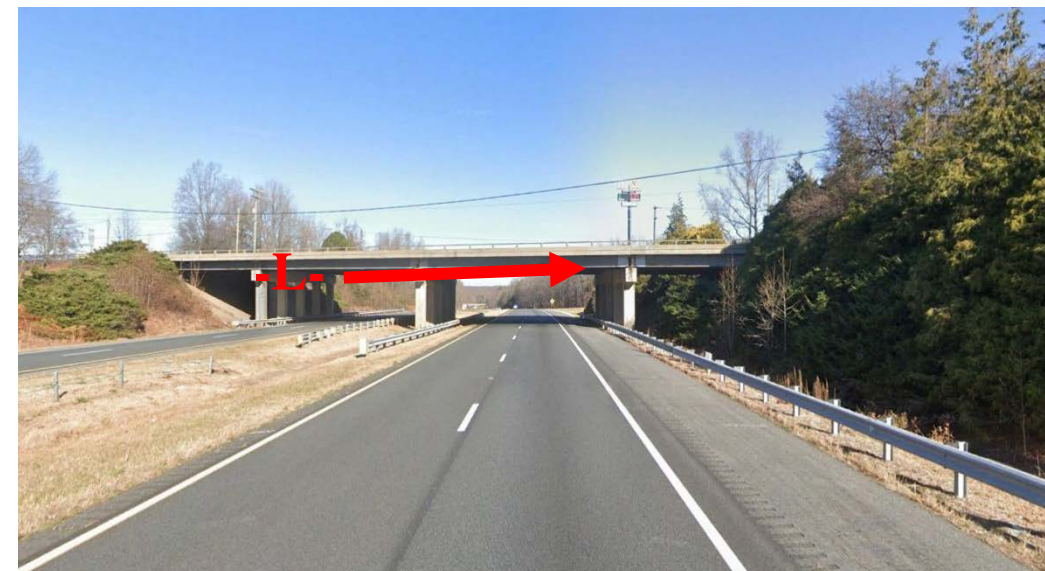
View of Bridge 0001 From South (Upstation Along -Y-)
