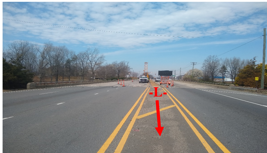
View of Along Bridge 0001 Looking Downstation
