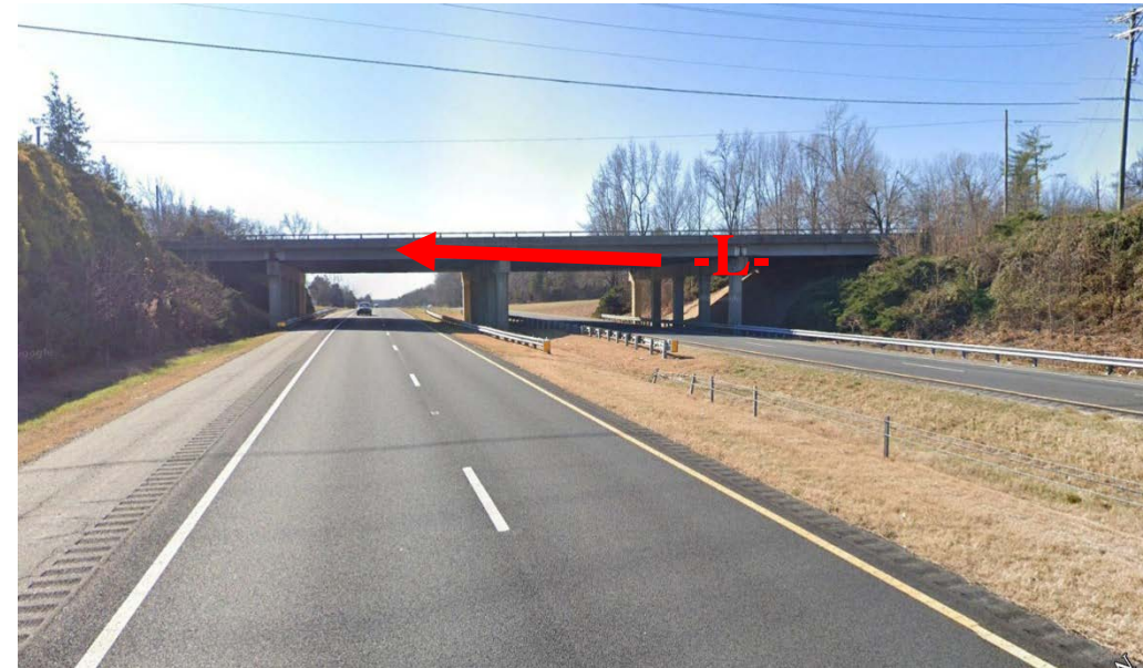
View of Bridge 0001 From North (Downstation along -Y-)
