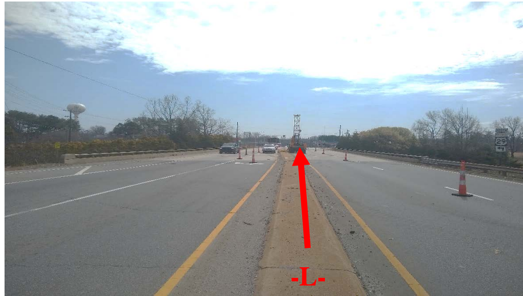
View Along Bridge 0001 Looking Upstation
