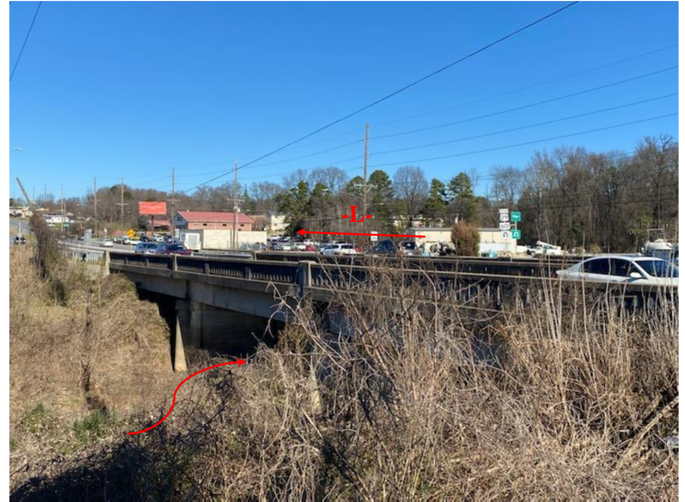
Photograph No. 2: Looking at End Bent 1 toward End Bent 2
