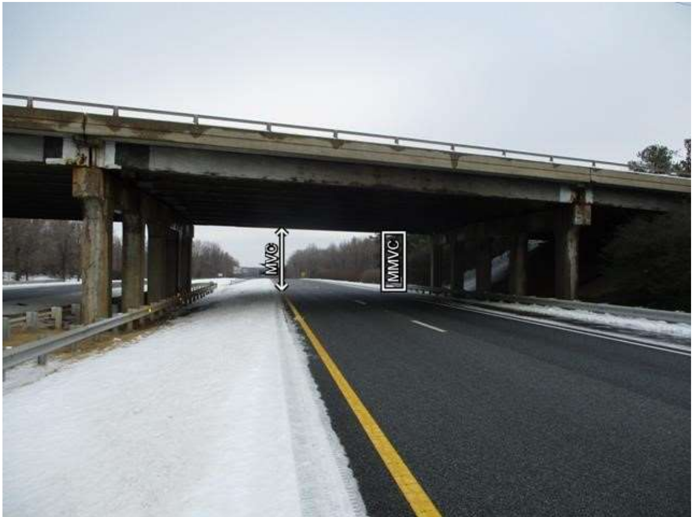
UNDERCLEARANCE PROFILE IN NORTHBOUND TRAVEL LANES
