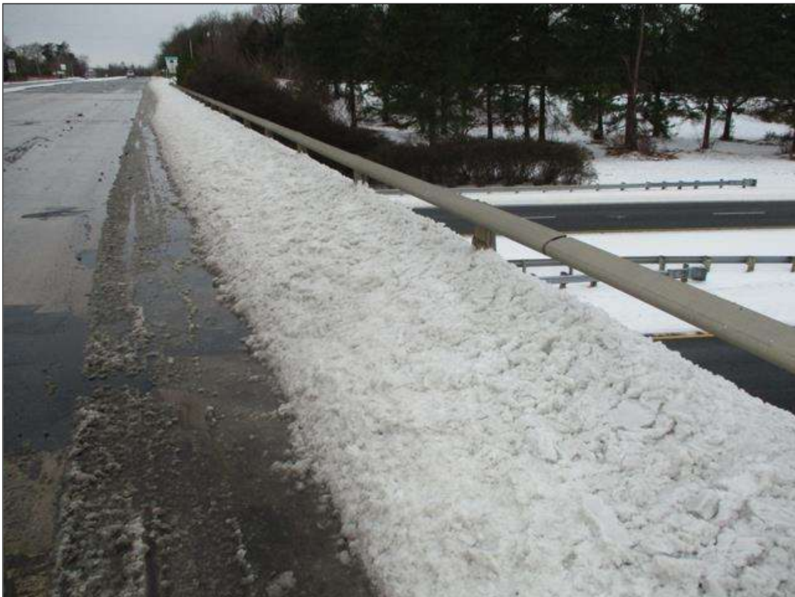
TYPICAL BRIDGE RAIL. OBSURED BY SNOW COVER
