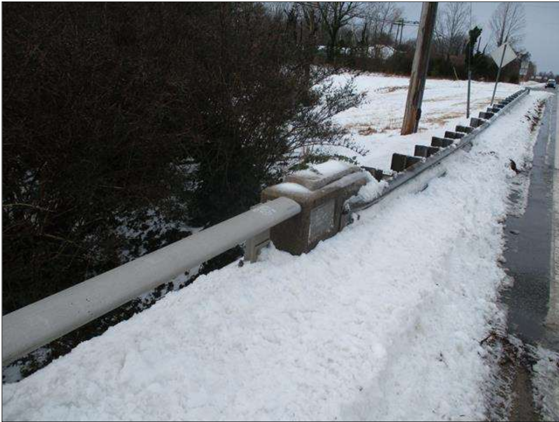
TYPICAL POST SPACING AT BRIDGE AT SOUTHWEST CORNER
