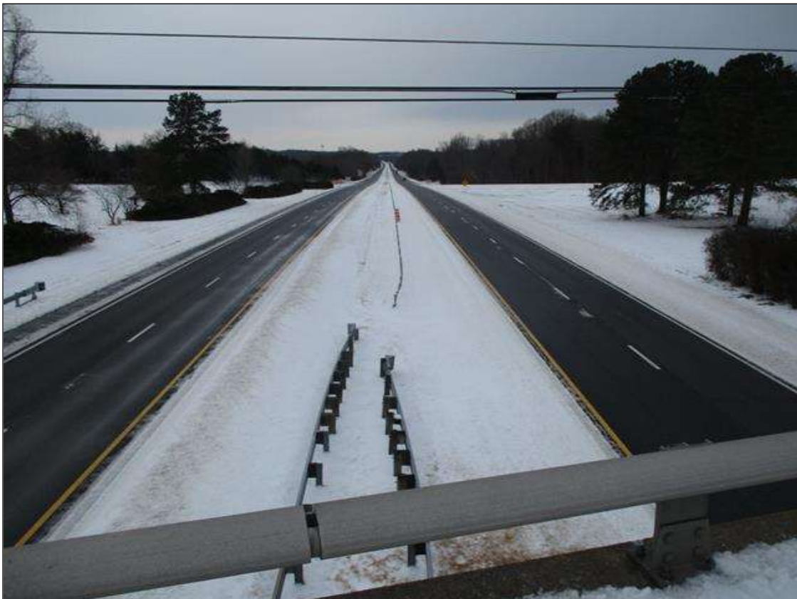
LOOKING SOUTH FROM TOP OF BRIDGE
