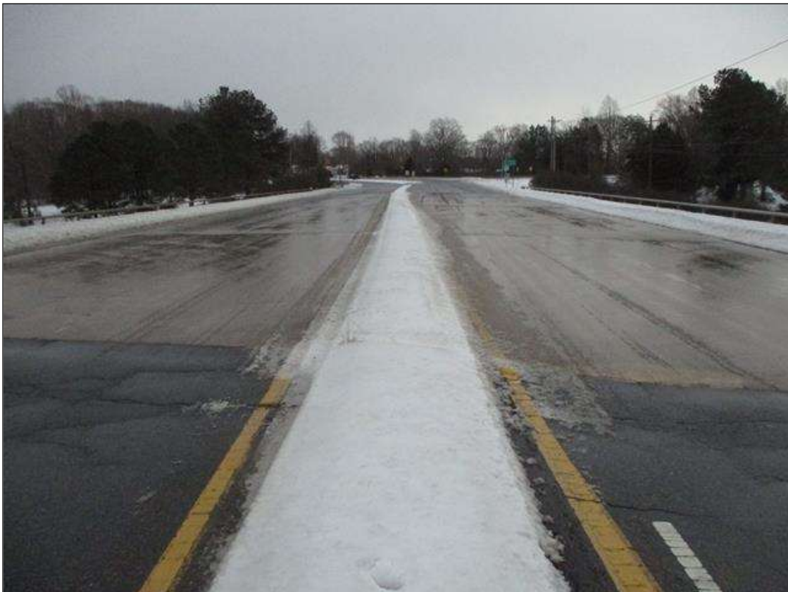
ROADWAY ON THE BRIDGE LOOKING EAST
