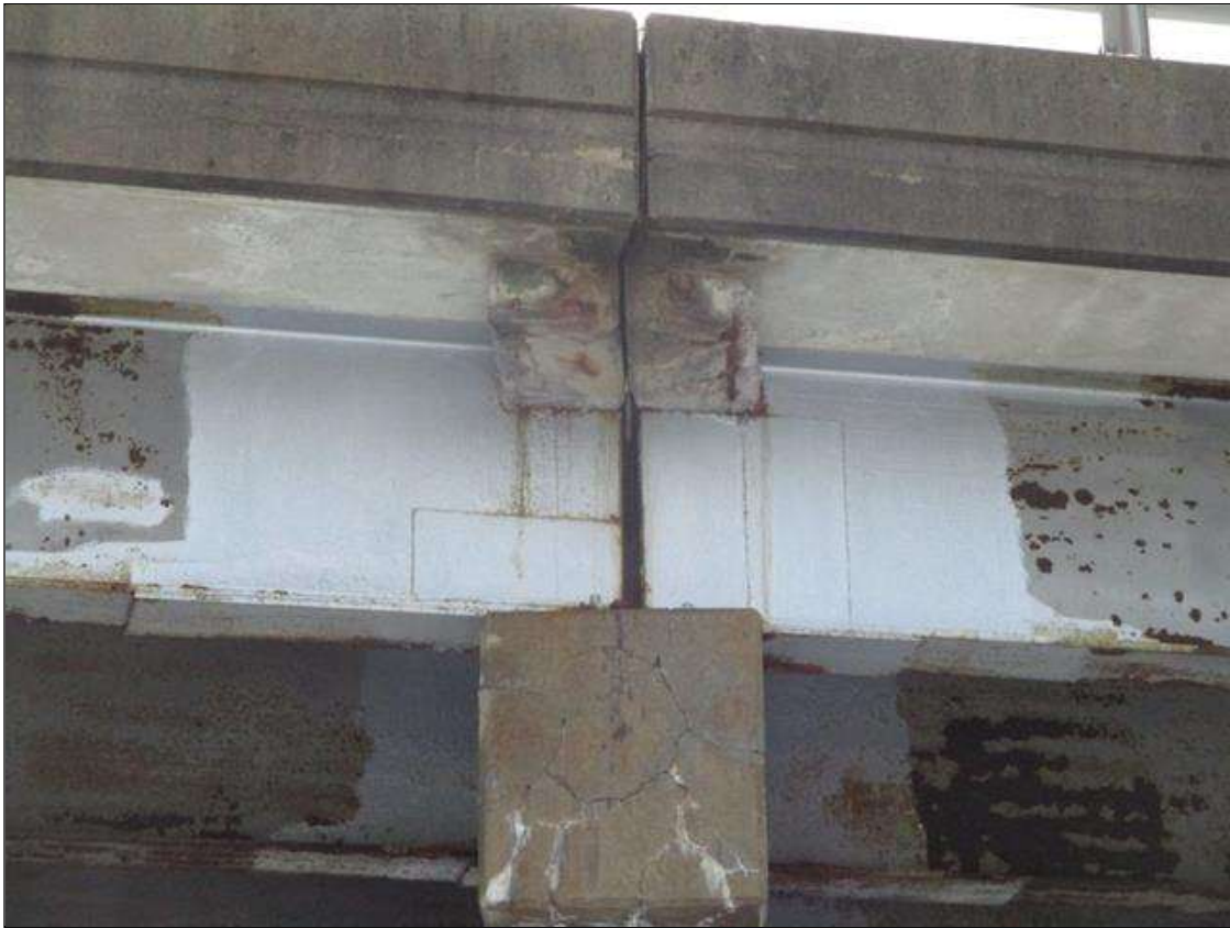
TYPICAL BEAM AND CAP ENDS LOOKING AT GIRDER 1 OVER BENT 2
