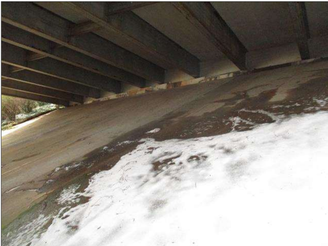
SLOPE PROTECTION AT ABUTMENT 1
