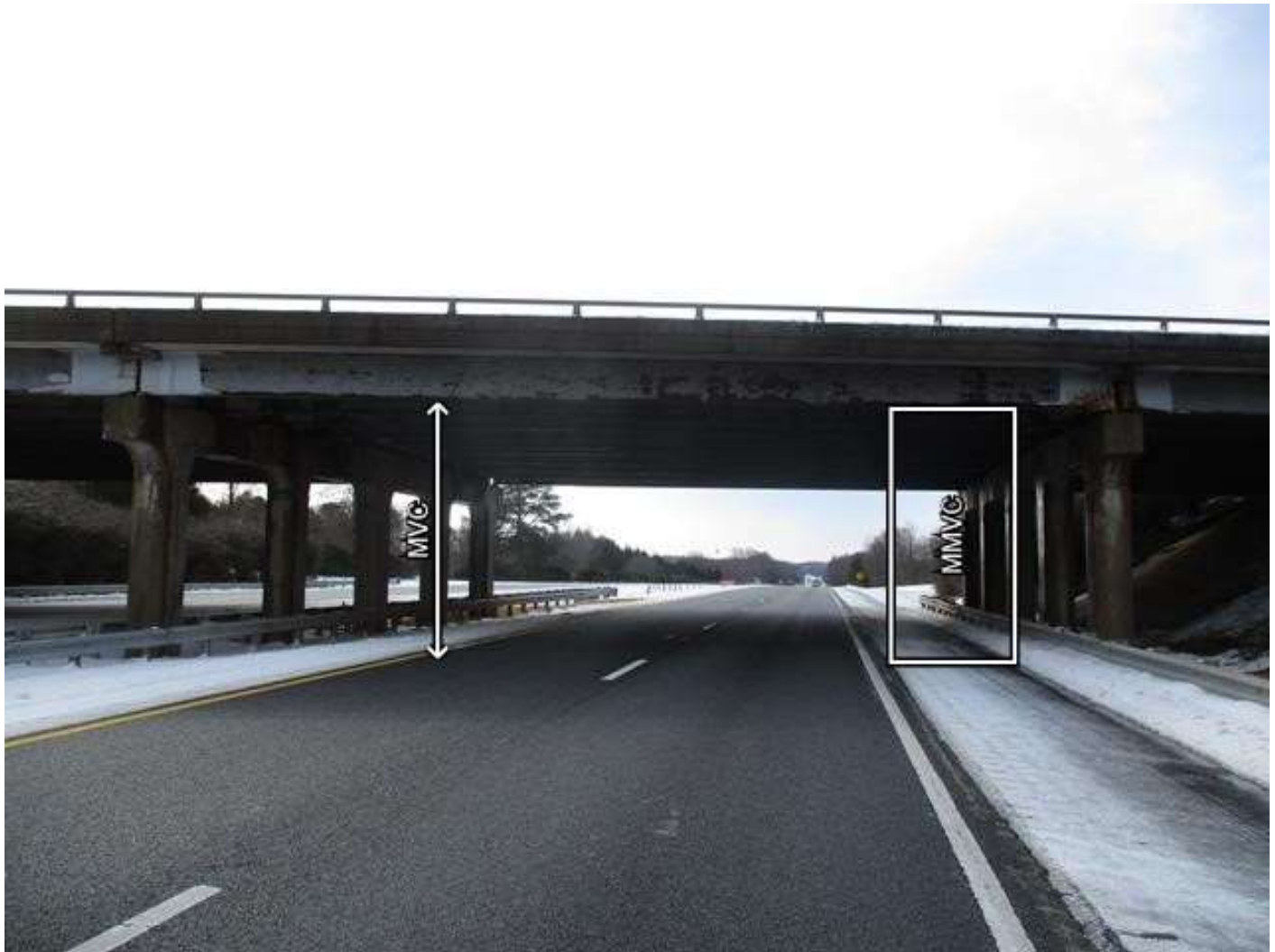
UNDERCLEARANCE PROFILE IN SOUTHBOUND TRAVEL LANES
