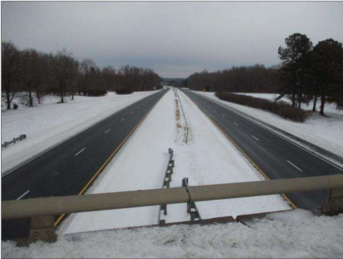
LOOKING NORTH FROM TOP OF BRIDGE
