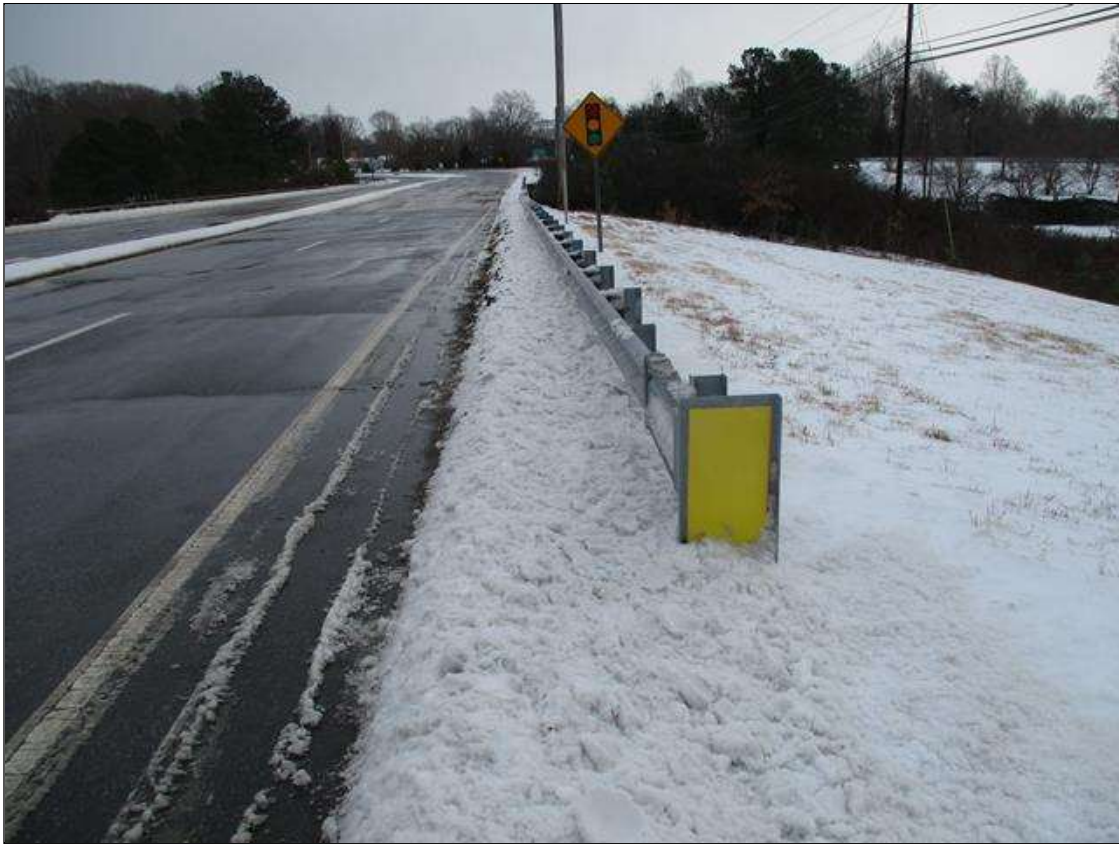
GUARDRAIL END TERMINAL AT SOUTHWEST CORNER
