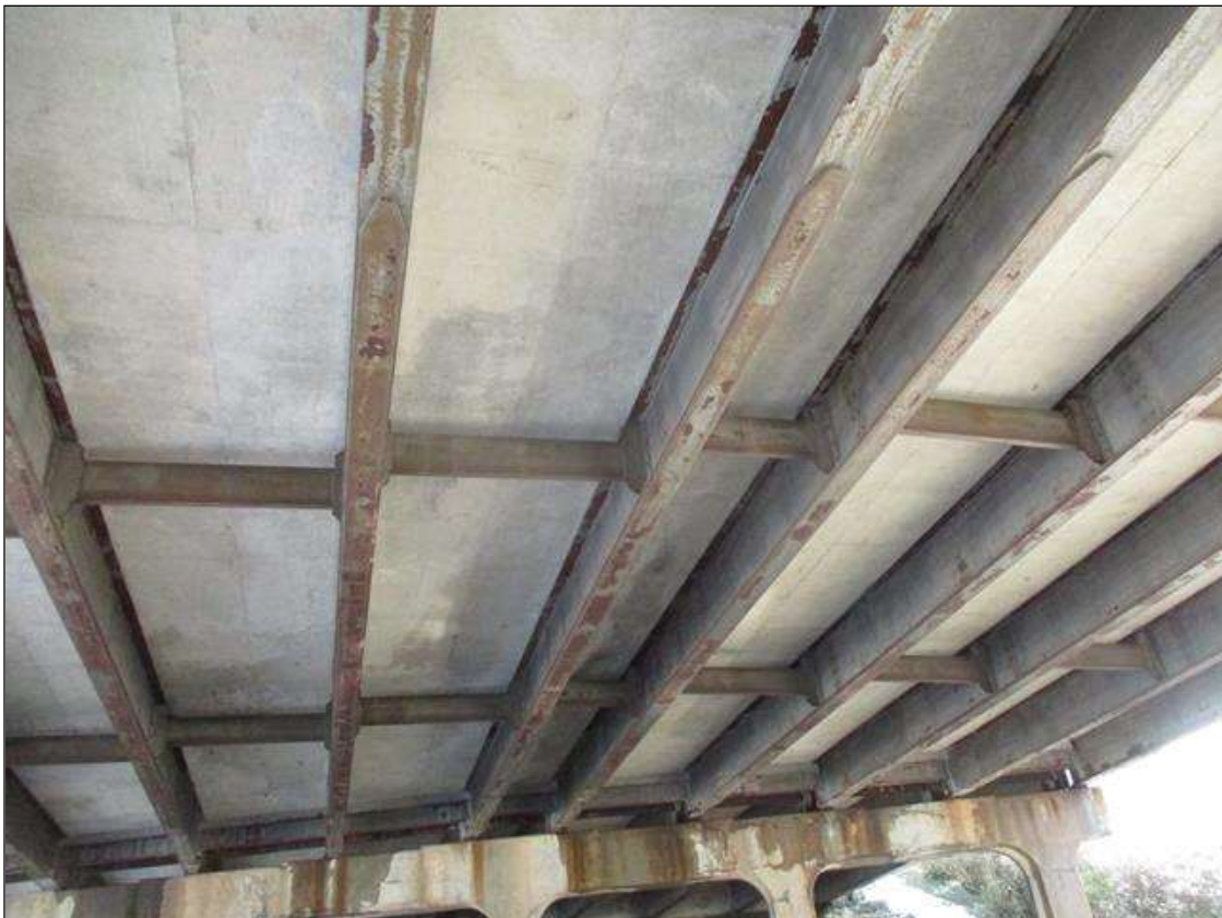
SUPERSTRUCTURE UNDERSIDE. TYPICAL IN ALL SPANS.
