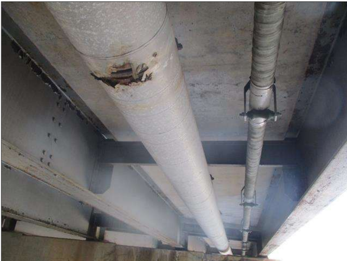
UTILITIES IN BAY 1
