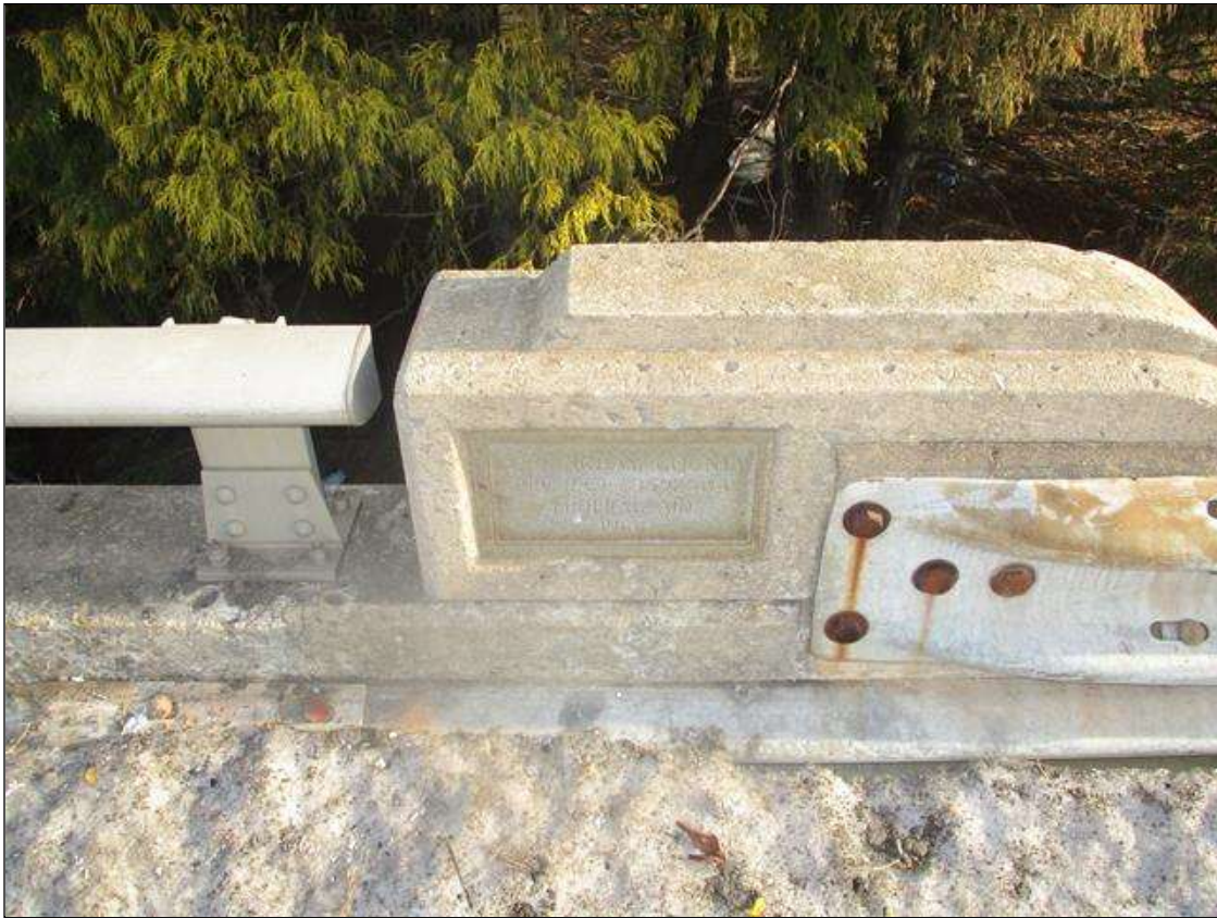
BRIDGE PLAQUE AT SOUTHWEST CORNER. TYPICAL AT NORTHWEST CORNER
