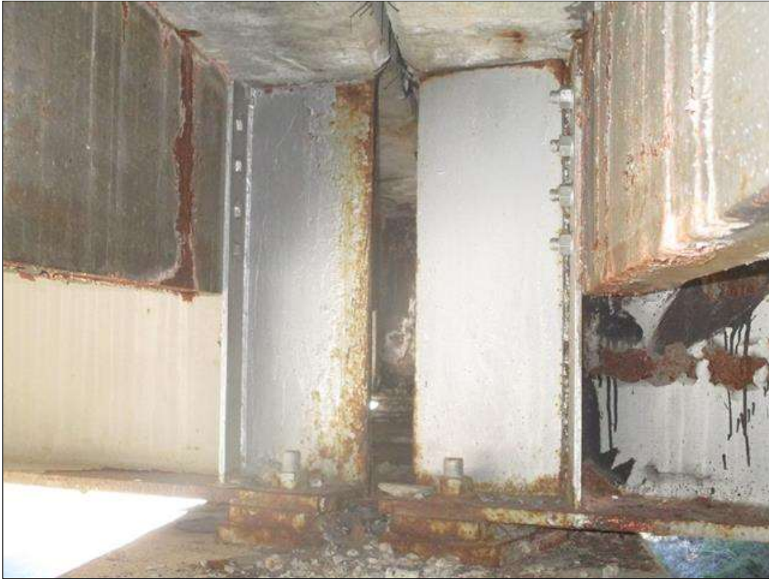
Span 4 Beam 8: WEB SECTION LOSS (UP TO 100%, AVG. 1/8IN REMAIN) TO TOP, 4IN L. X 1IN H.) AT NEAR END WITH REPAIR PLATE (3/4IN) AT RIGHT SIDE, PLATE DOES NOT COVER FULL HT. OF WEB (PAR)
