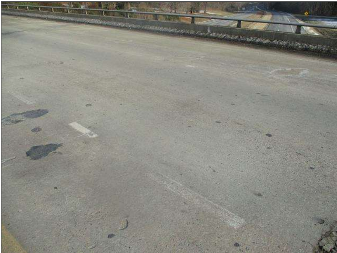
TOP OF DECK, FAIR CONDITION
