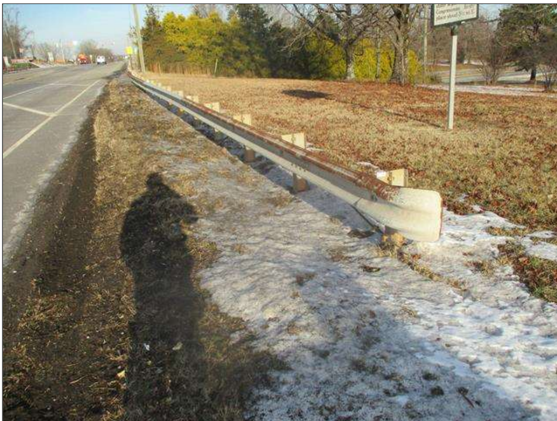
GUARDRAIL END TREATMENT AT SOUTHEAST CORNER. TYPICAL AT NORTHWEST
