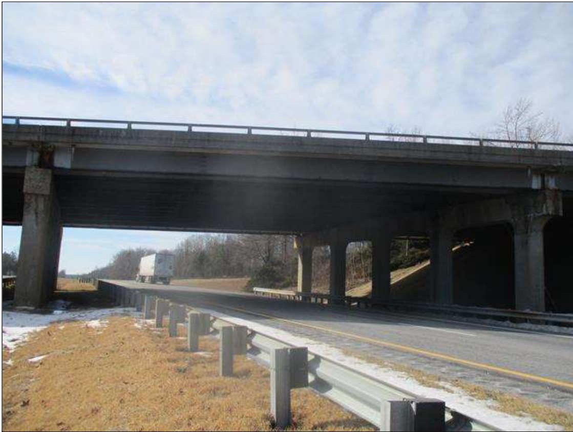
WESTBOUND UNDERCLEARANCE PROFILE IN SPAN 2
