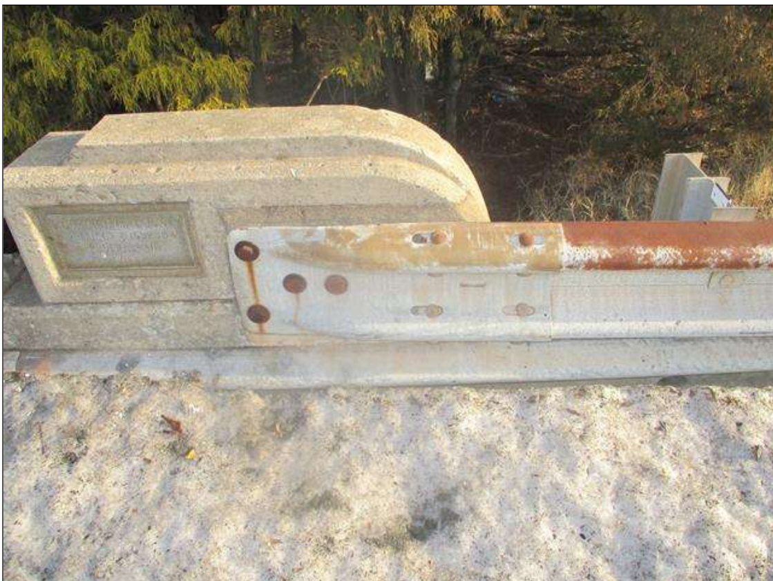
GUARDRAIL TO BRIDGE RAIL ATTACHEMENT AT SOUTHWEST CORNER
