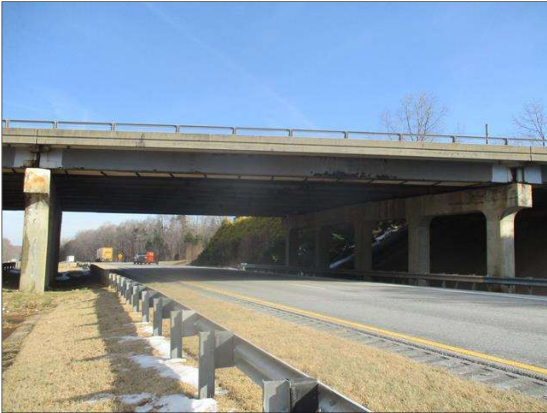
EASTBOUND UNDERCLEARANCE PROFILE IN SPAN 3
