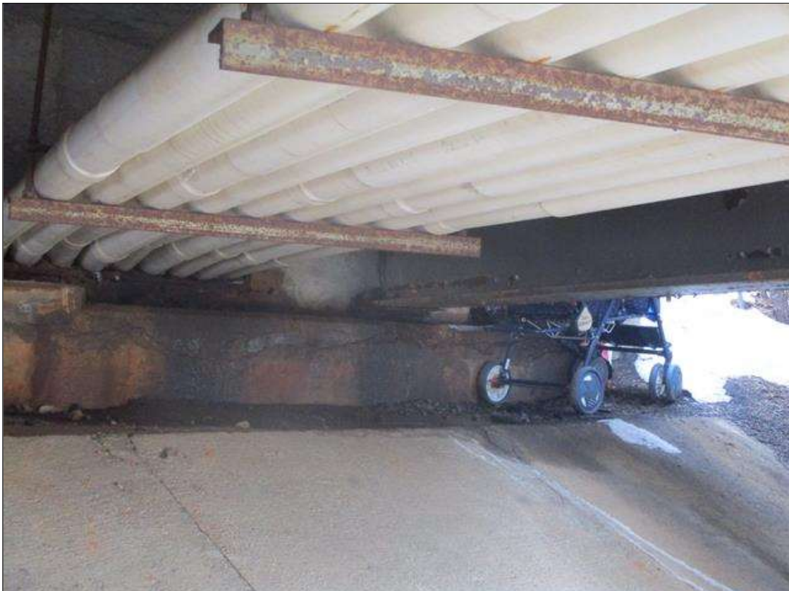
HOMELESS CAMP UNDER SPAN 4
