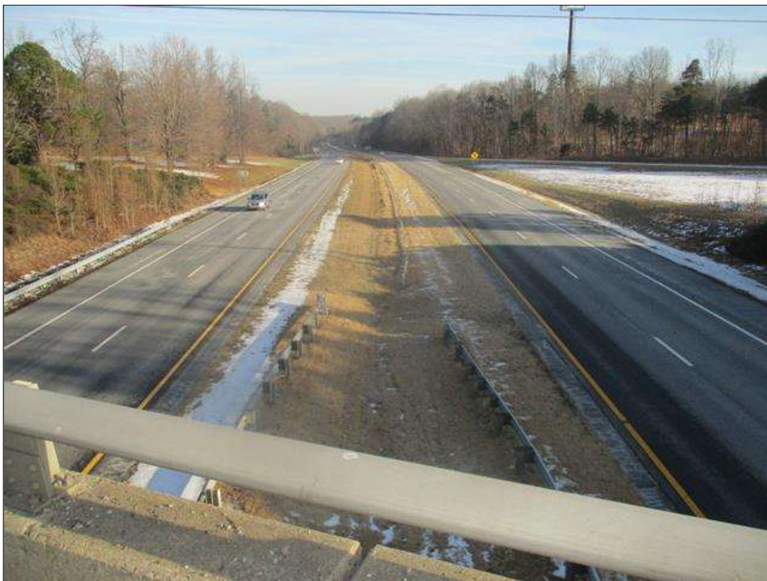
LOOKING EAST FROM TOP OF BRIDGE
