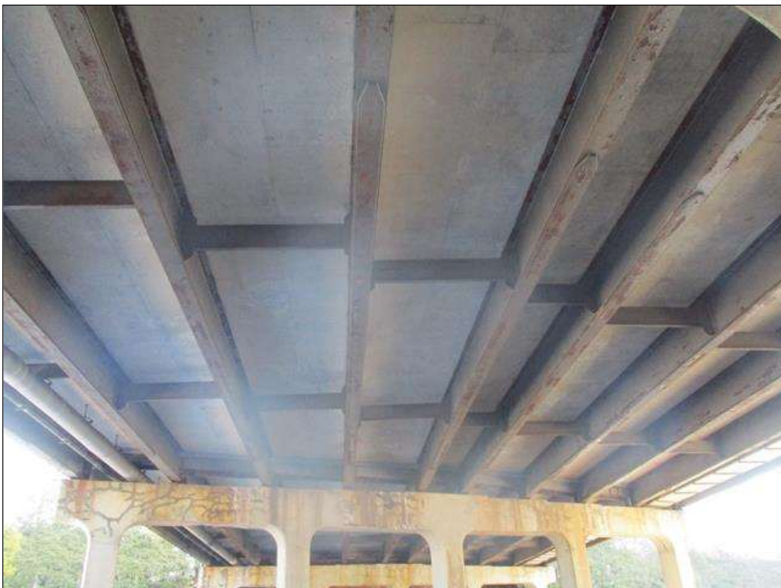
SUPERSTRUCTURE UNDERSIDE IN SPAN 2. TYPICAL IN OTHER SPANS.
