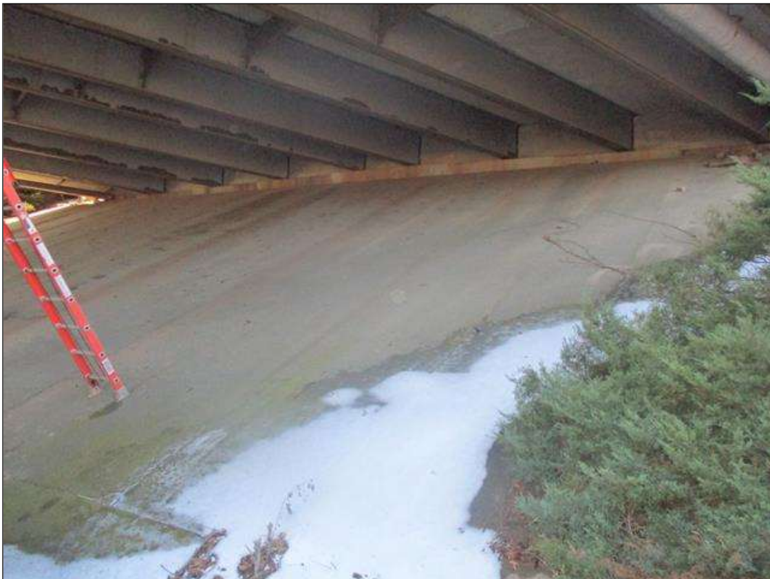
SLOPE PROTECTION AT END BENT 1
