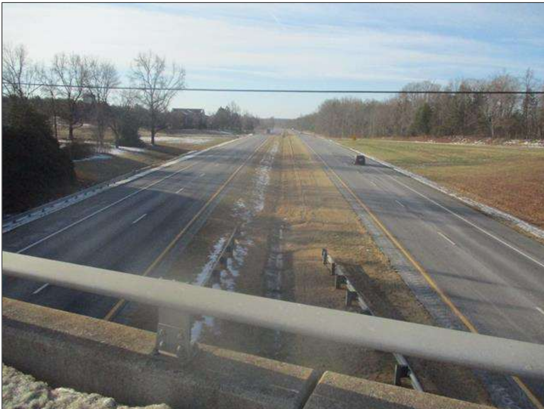
LOOKING WEST FROM TOP OF BRIDGE
