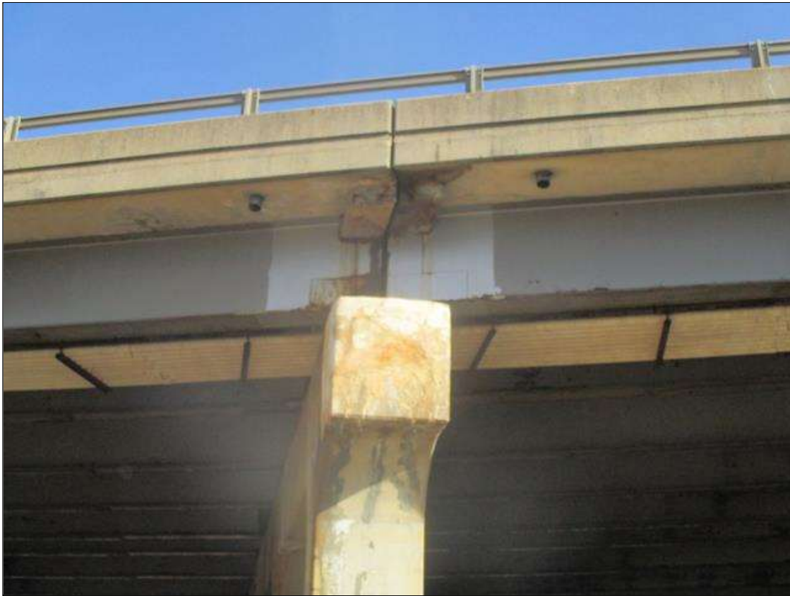
BEAM AND CAP ENDS AT BENT 2. TYPICAL
