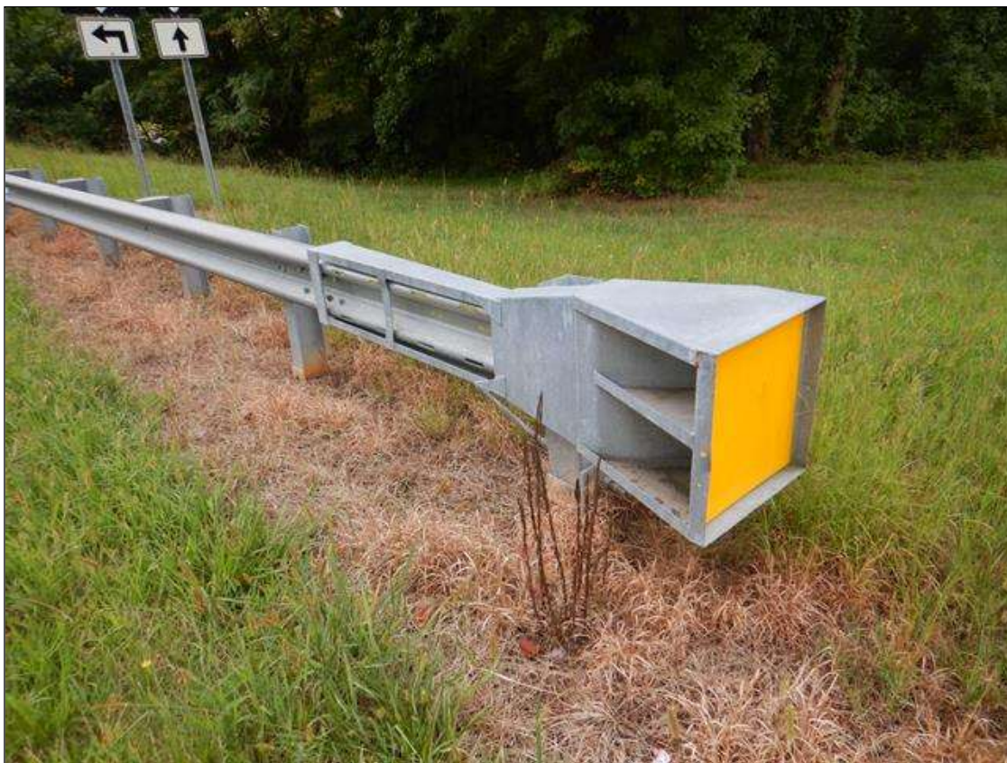
GUARDRAIL END TERMINAL, SOUTHWEST CORNER
