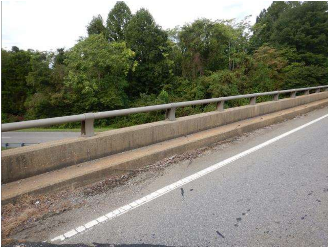
RIGHT BRIDGE RAIL
