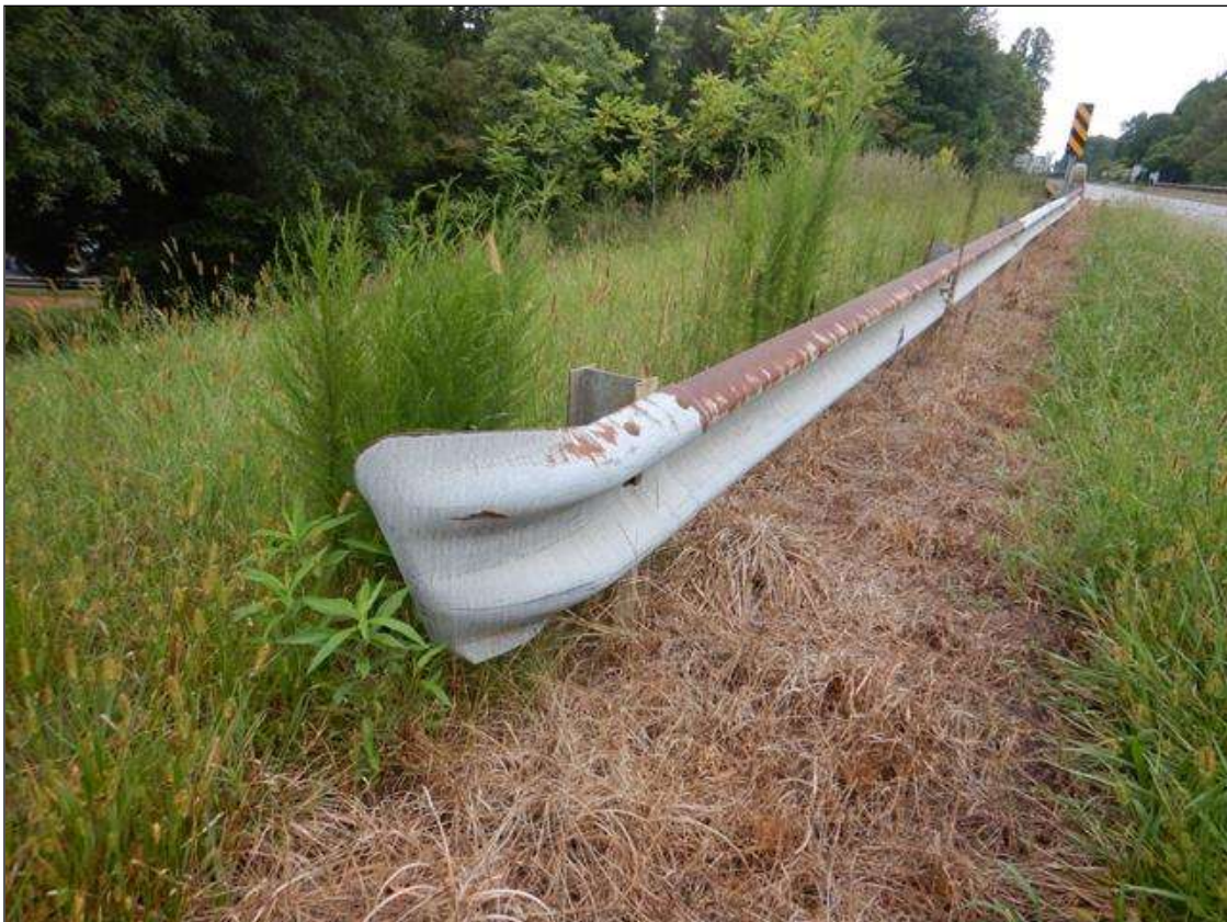
GUARDRAIL END TERMINAL, SOUTHEAST CORNER
