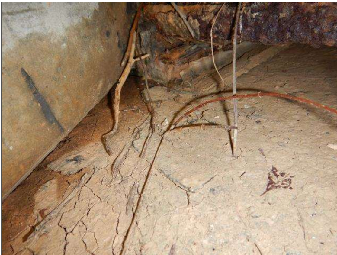
Span 1 Beam 4 - Near Bearing: 1 Each of Corrosion: Freckled rust. Corrosion of the steel has initiated.
