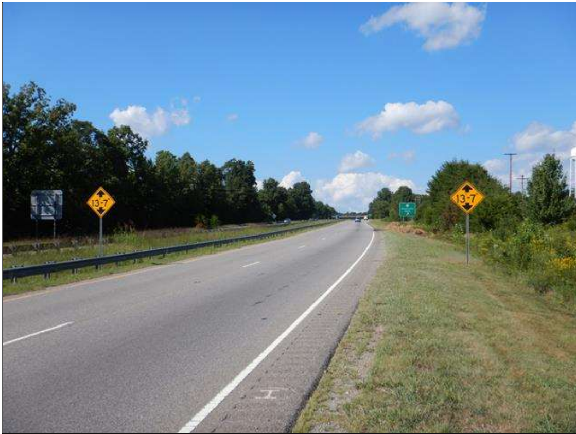
ADVANCE CLEARANCE SIGNS US220 NORTH BOUND LANE
