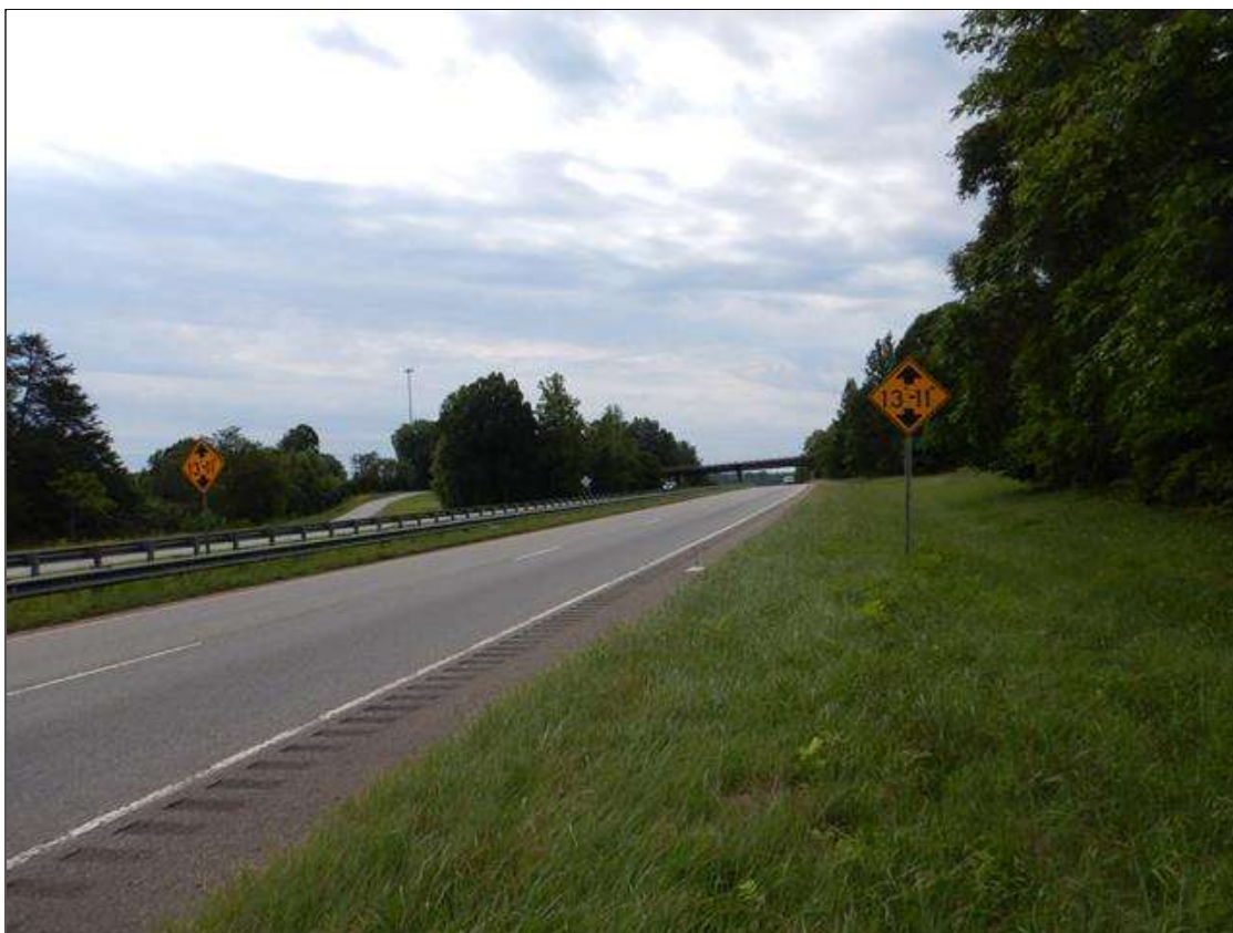
CLEARANCE POSTINGS, US220 SOUTH BOUND
