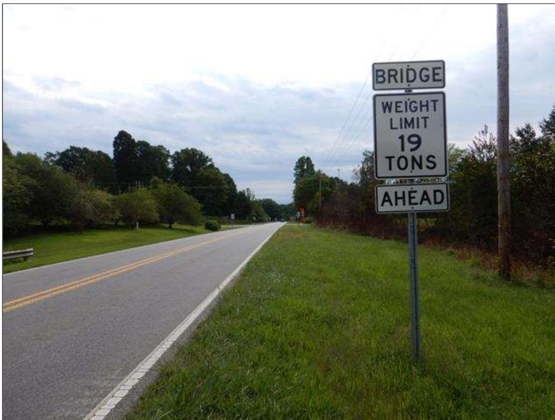
ADVANCED WEIGHT POSTING, WEST APPROACH
