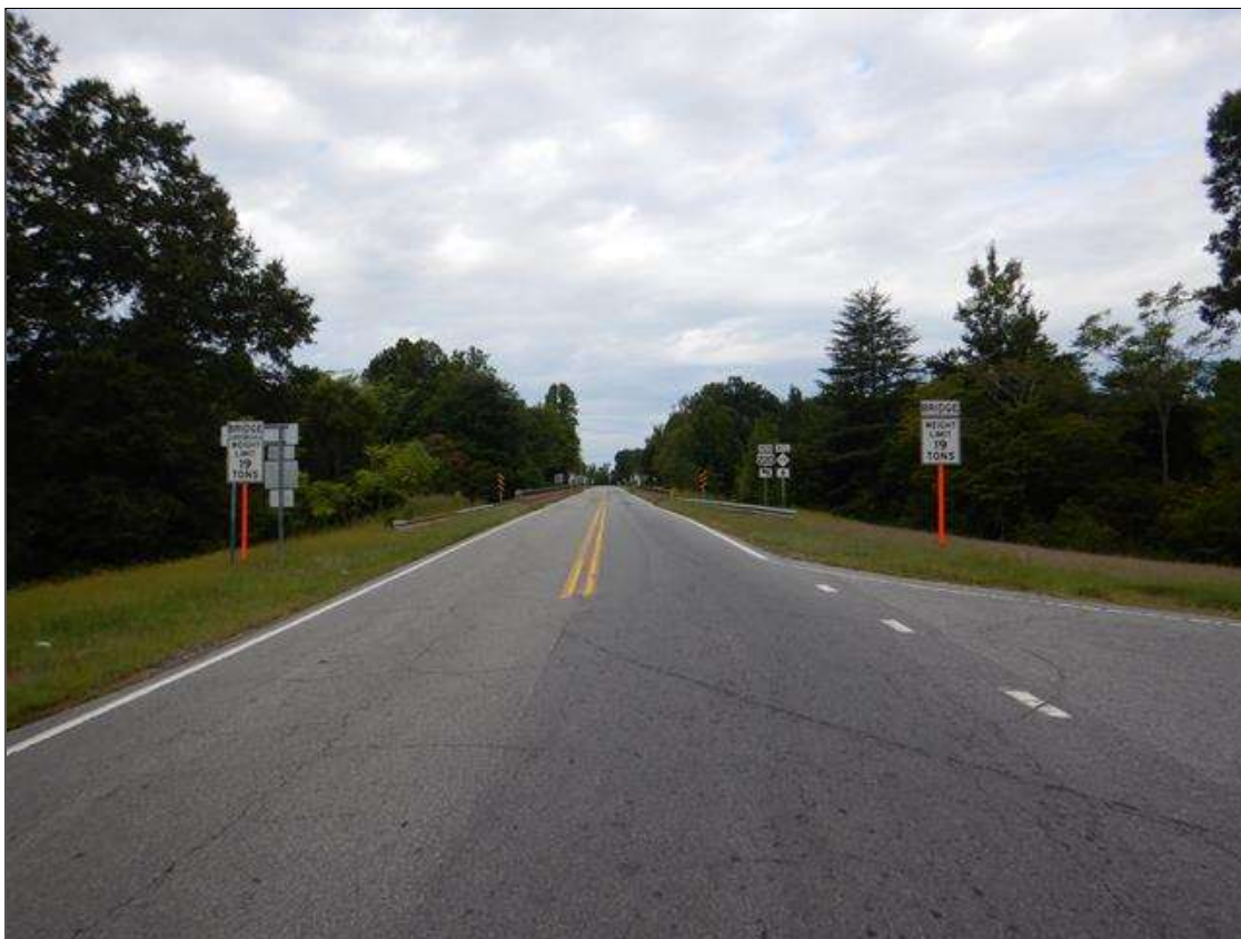
EAST APPROACH WEIGHT POSTINGS, NEWLY INSTALLED SINCE PREVIOUS INSPECTION
