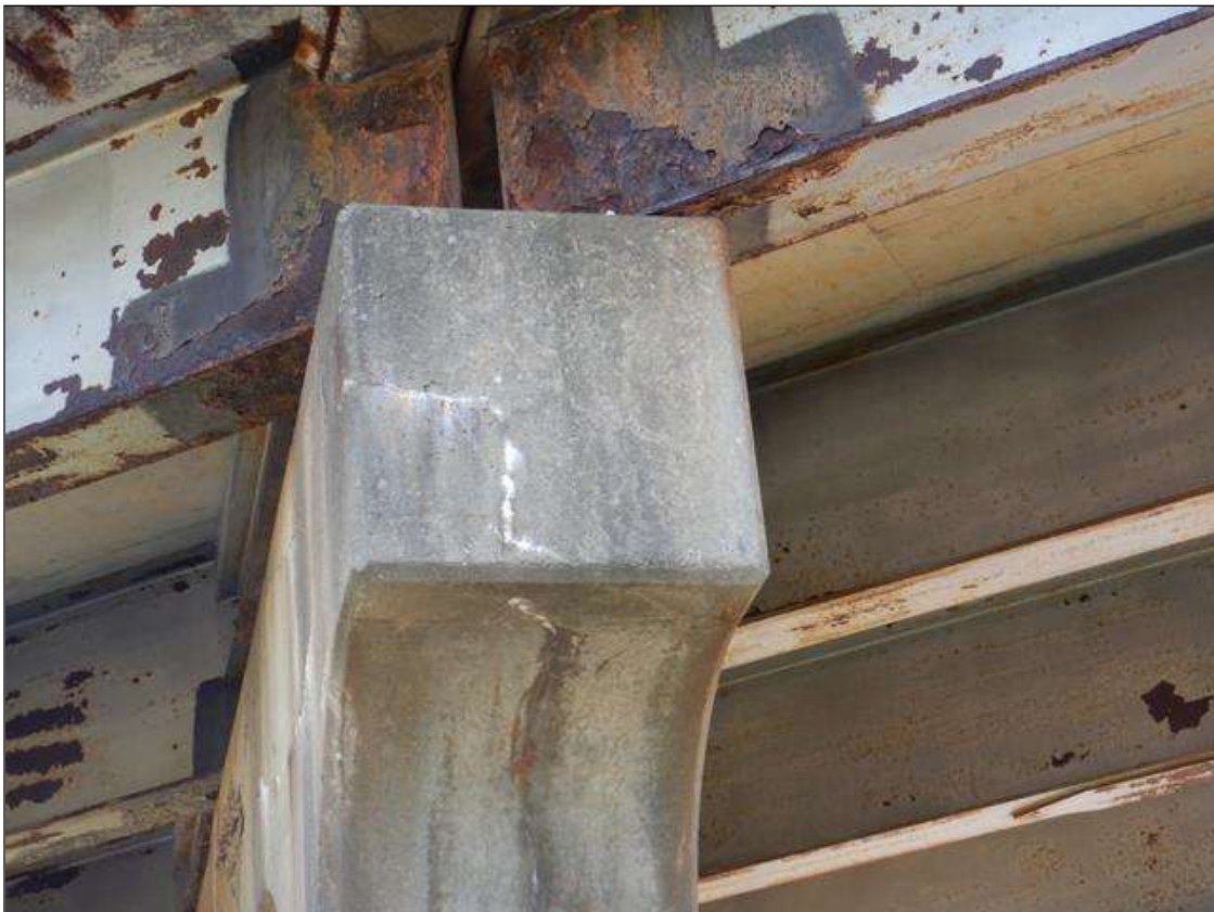
BEAM AND CAP ENDS, LEFT END CAP BENT 2
