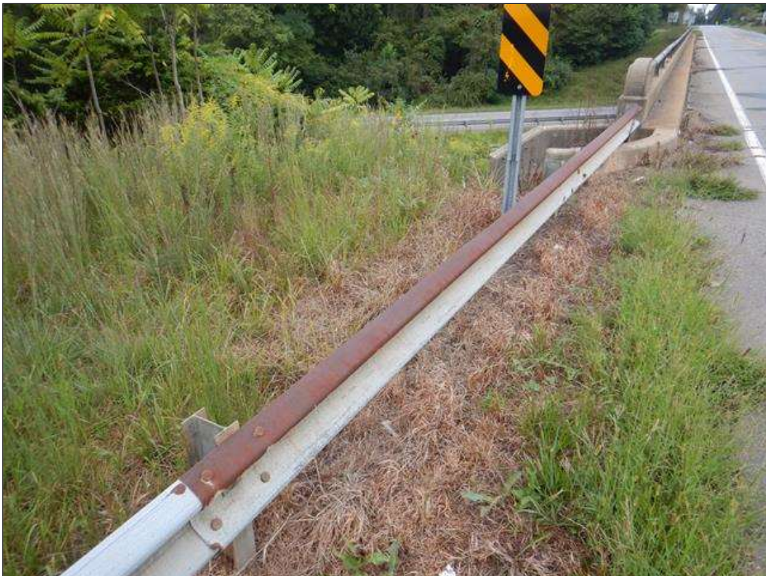
TYPICAL POST SPACING, SOUTHEAST CORNER
