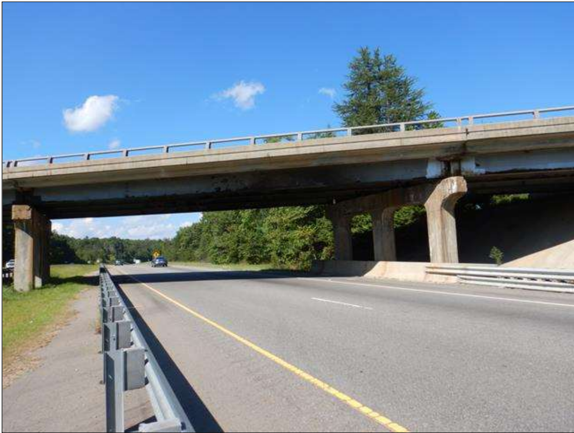
UNDERCLEARANCE US220 NORTH BOUND, LOOKING NORTH
