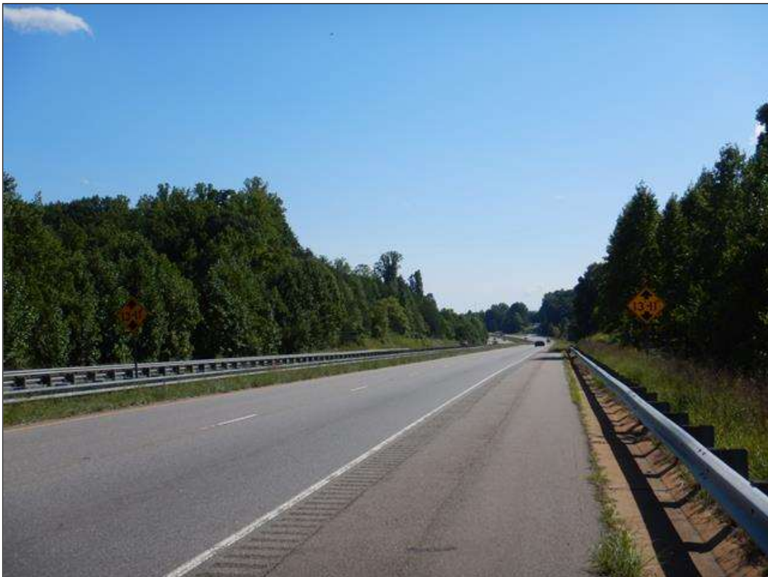
ADVANCE CLEARANCE SIGNS, US220 SOUTH BOUND LANE
