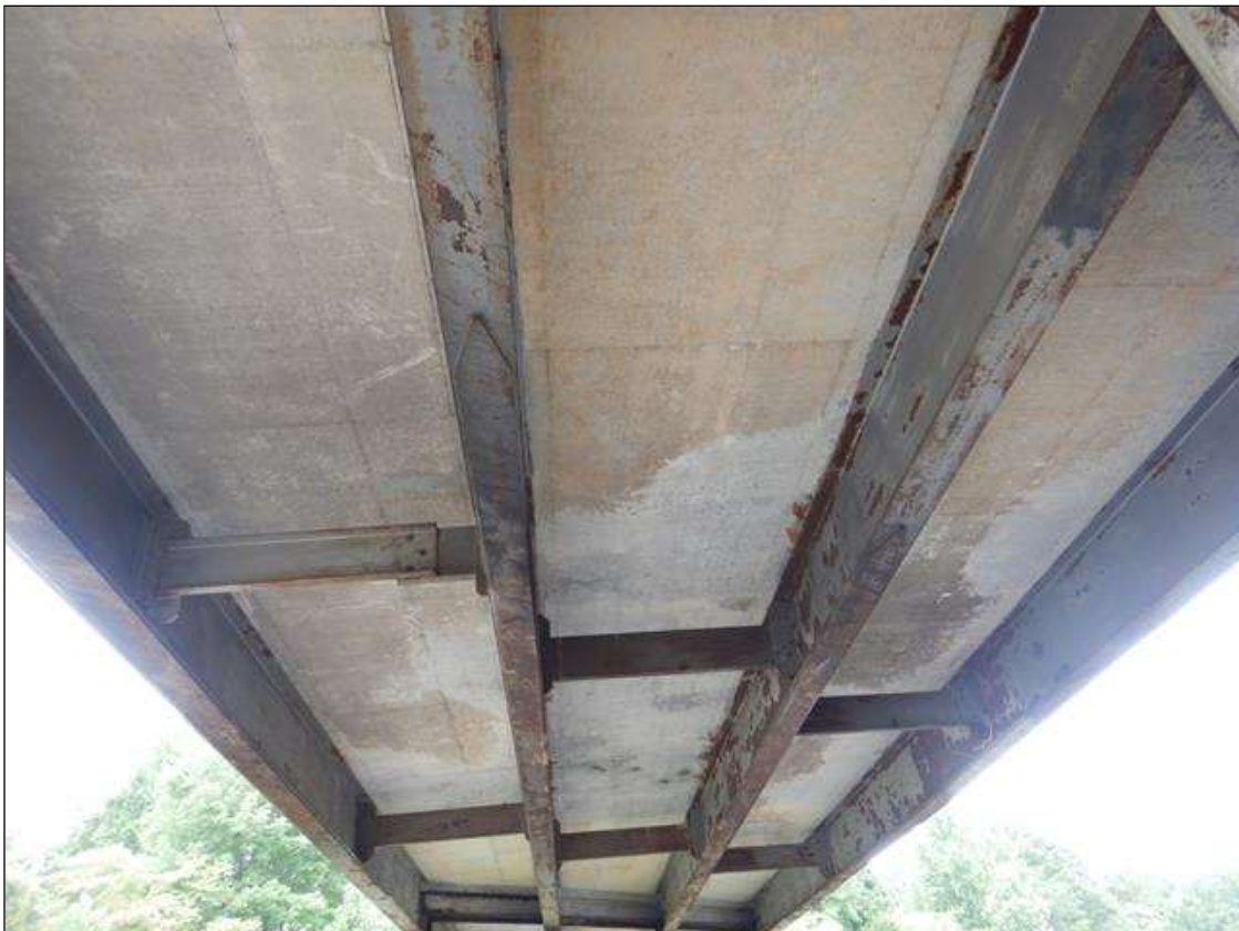
SUPERSTRUCTURE UNDERSIDE, SPAN 3
