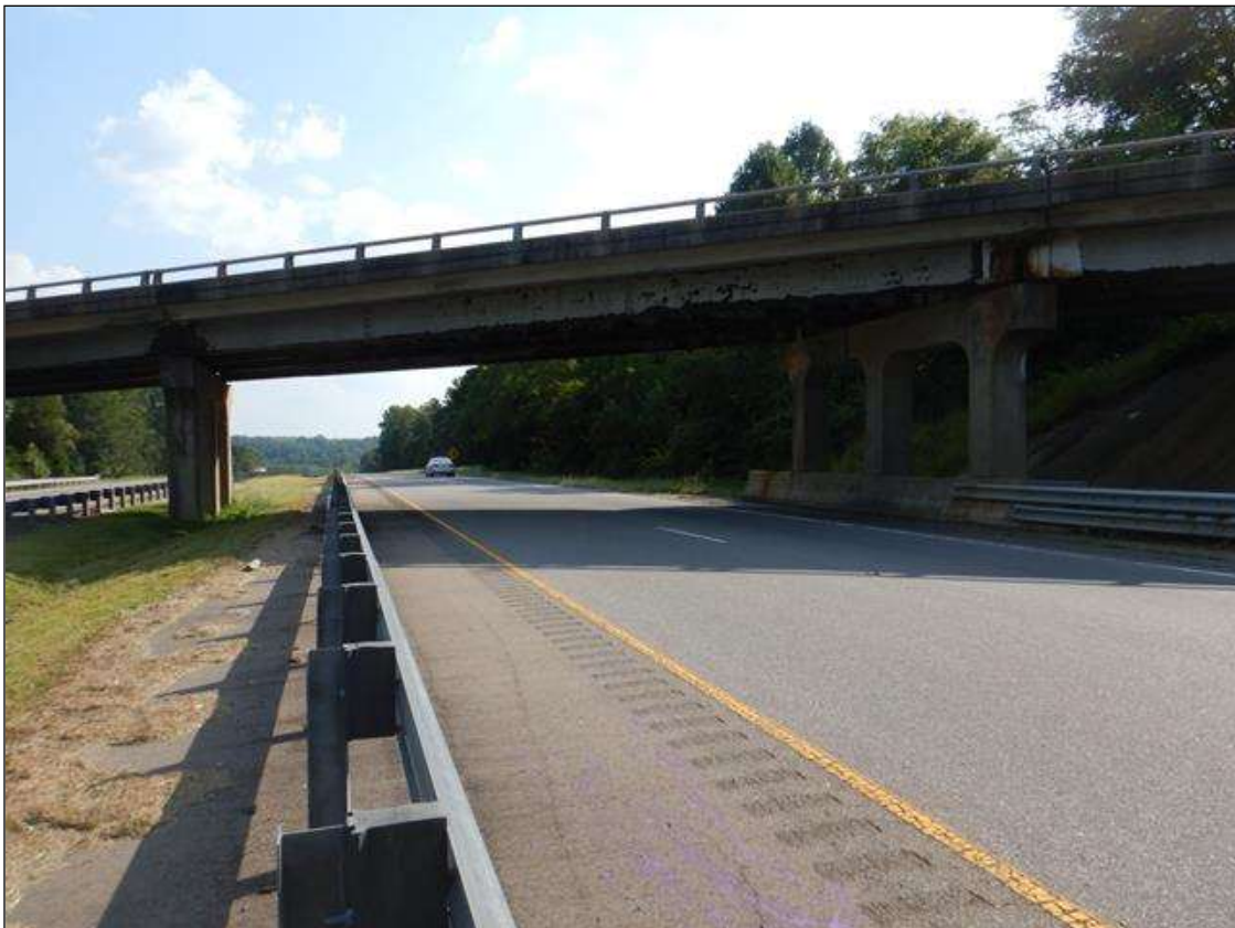
USS220 SOUTHBOUND UNDERCLEARANCE, LOOKING SOUTH
