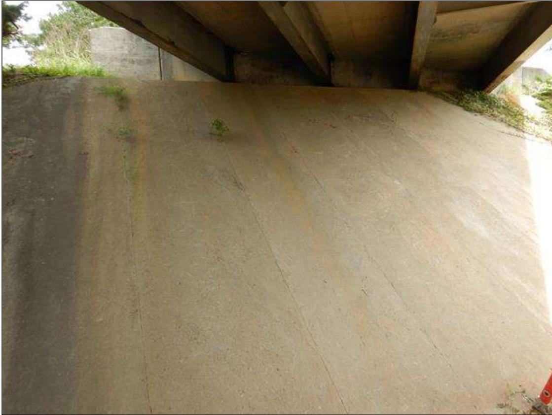
SLOPE PROTECTION END BENT 2
