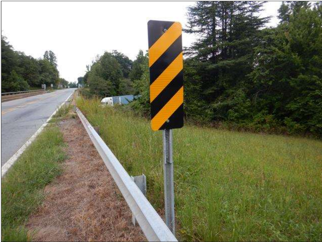
TYPICAL DELINEATOR, NORTHEAST CORNER
