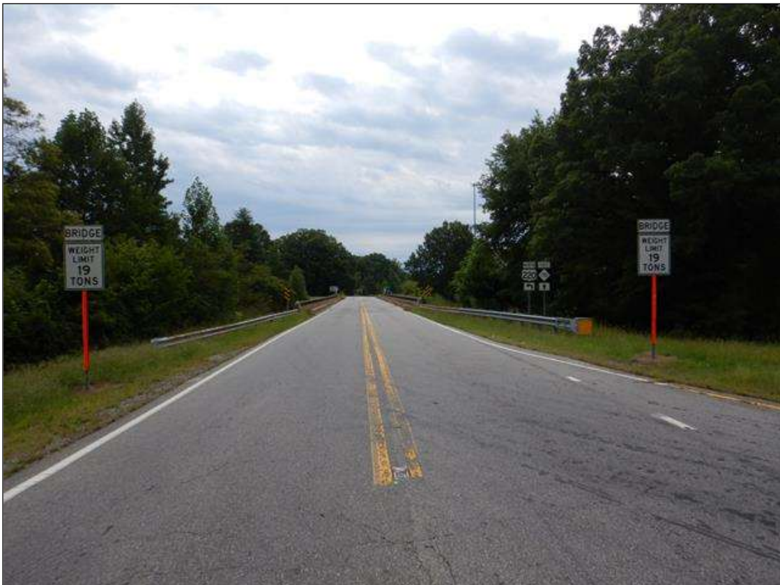
WEIGHT POSTINGS, WEST APPROACH, NEWLY INSTALLED SINCE PREVIOUS INSPECTION
