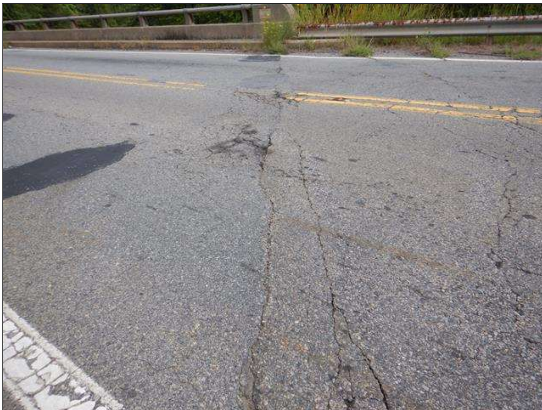
END BENT 2 JOINT
