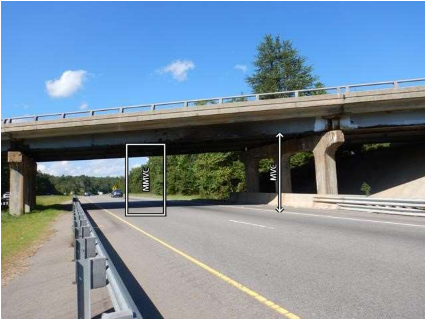
UNDERCLEARANCE US220 NORTH BOUND, LOOKING NORTH
