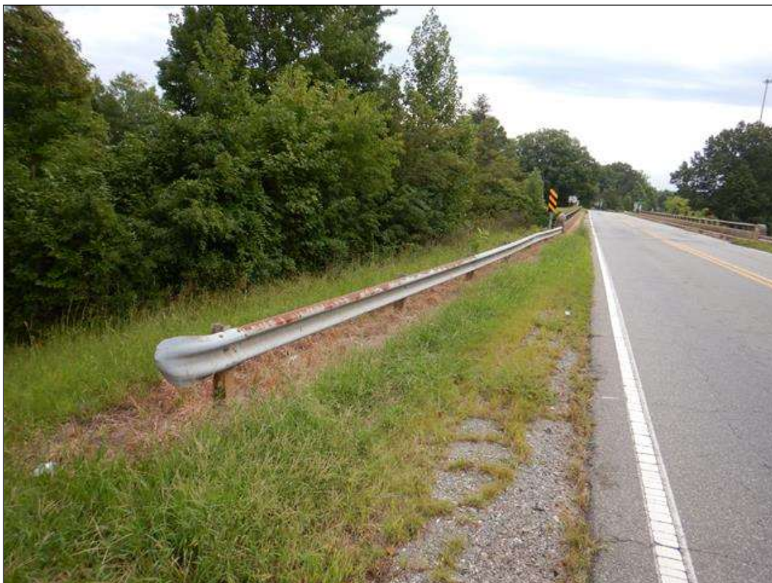
GUARDRAIL, NORTHWEST CORNER
