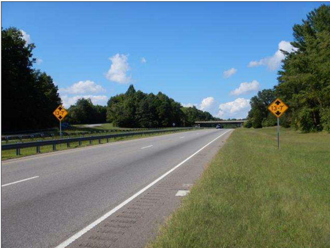
CLEARANCE SIGNS US220 NORTH BOUND LANE
