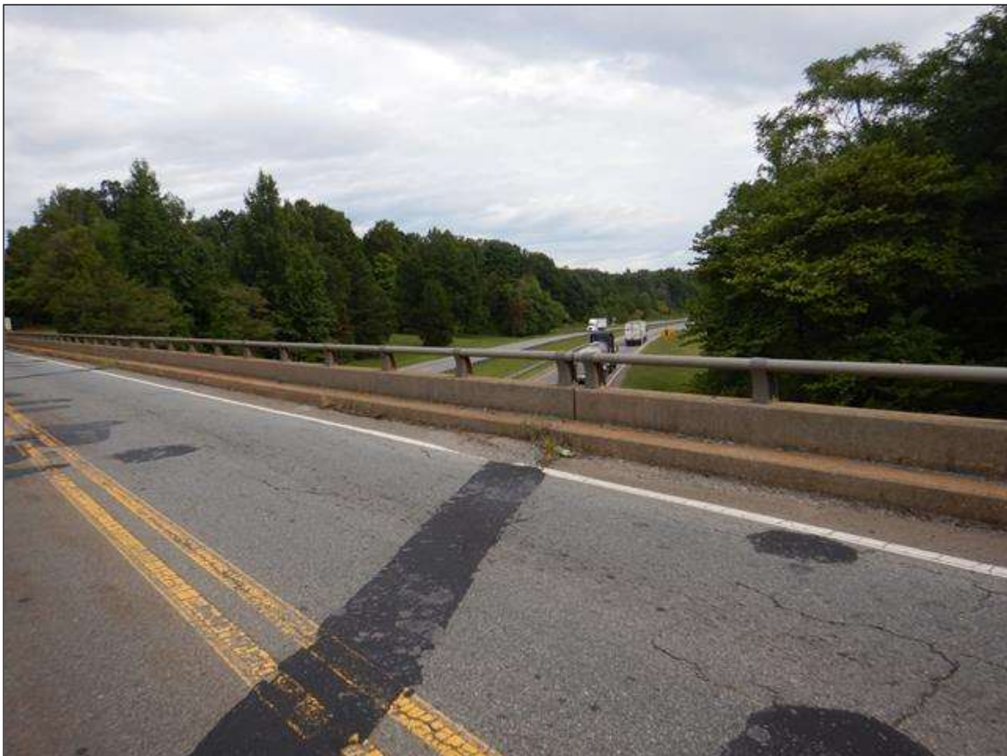
LEFT BRIDGE RAIL
