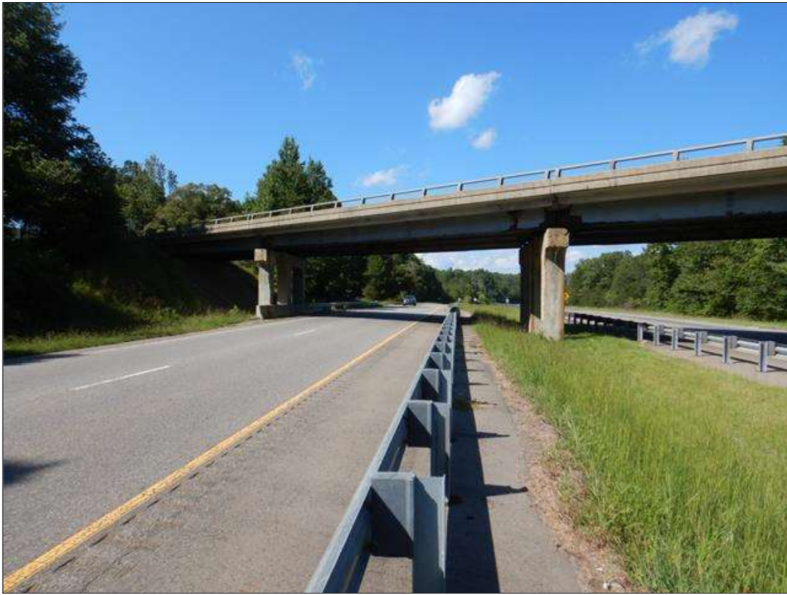
UNDERCLEARANCE US220 SOUTH BOUND, LOOKING NORTH
