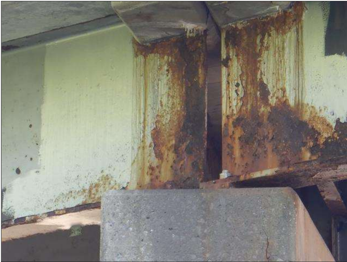
SPAN 1 GIRDER 4 BENT 1 RIGHT FACE
