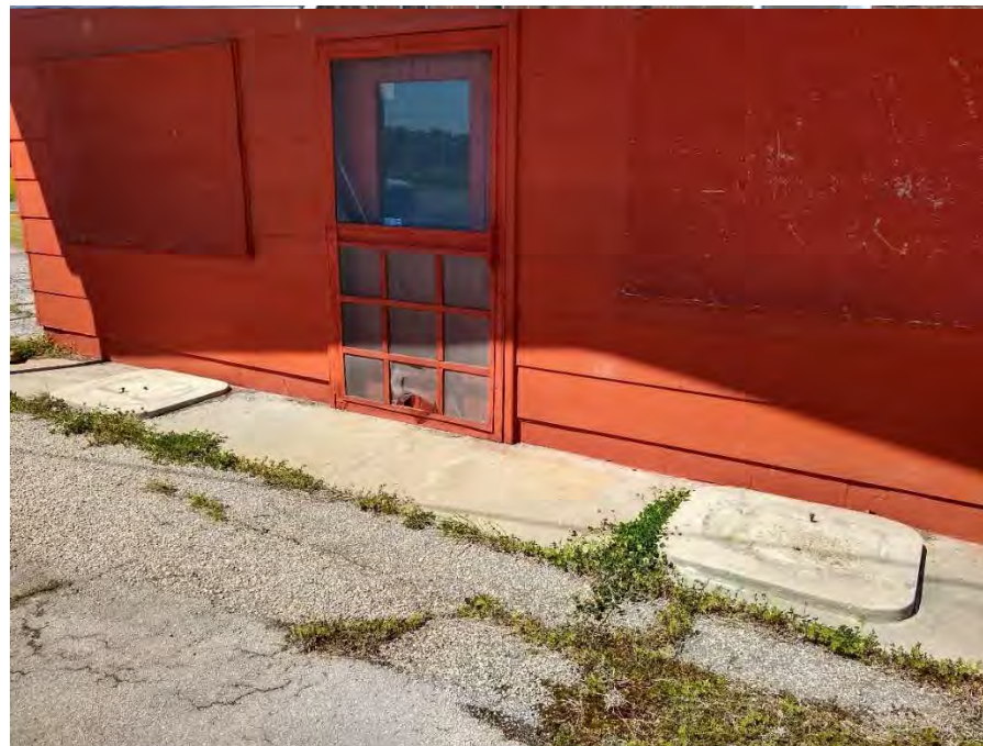
C. Close-up view of old dispenser pedestal locations on the front of the building.
