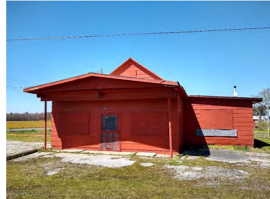
B. Front of former gas station building, photograph taken looking west. Note relic concrete pads on porch from former dispenser locations.
