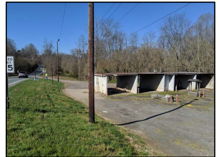
View of Survey Area (Facing Approximately Southwest)
