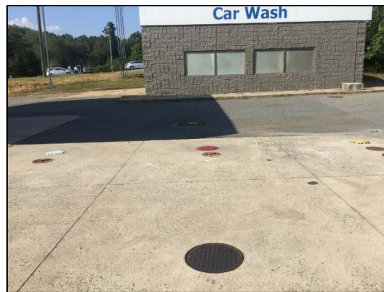
Fuel USTs, with car wash
