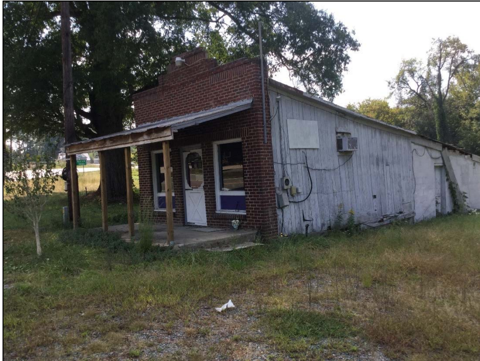
Building front and entrance, facing south.
