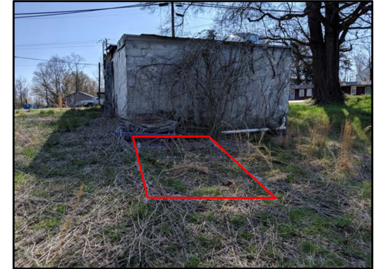
View of Suspected Septic Tank (Facing Approximately East)
