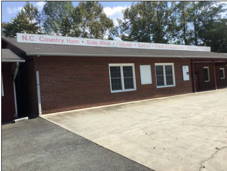
Looking SE from S. Main St. (US 311) at the front of facility
