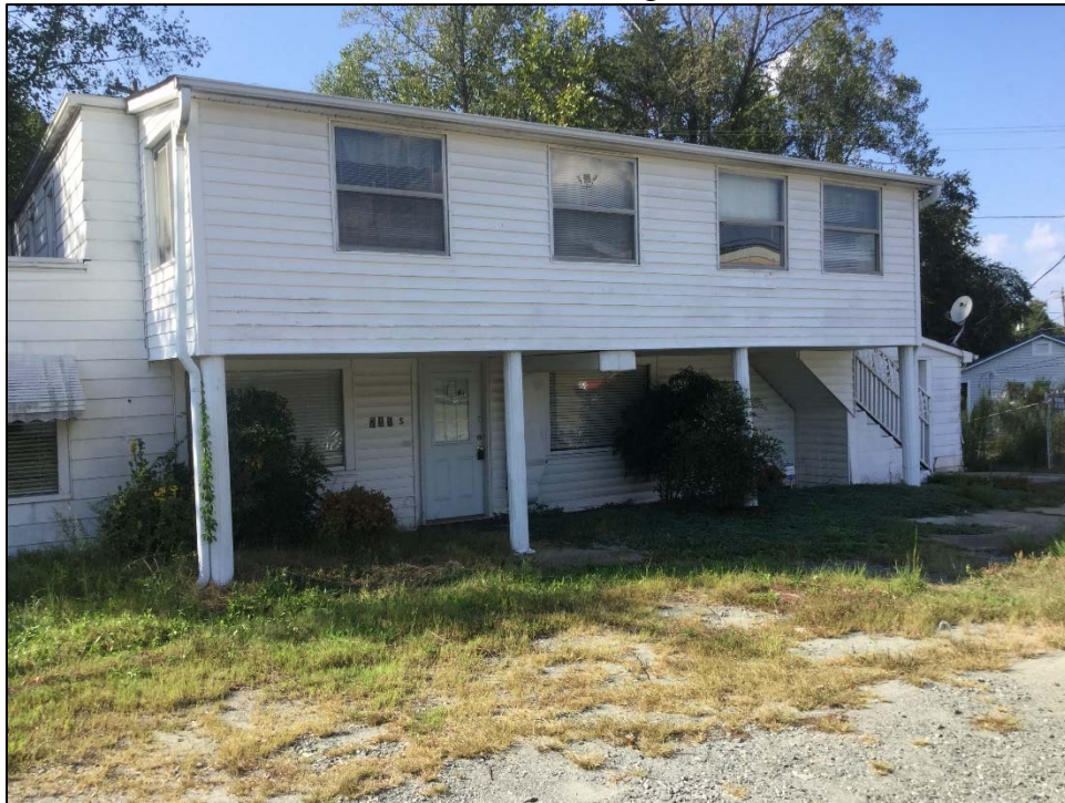
Front of building
