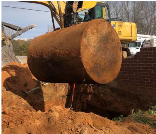
Removal of the Heating Oil UST from the subsurface (12.01.2021)
