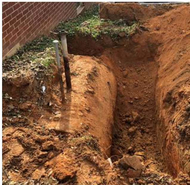
Uncovering the west sidewall of the Heating Oil UST (12.01.2021)
