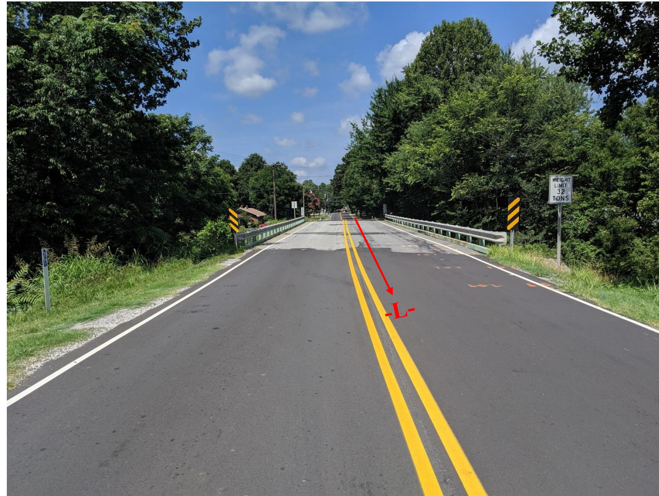
Photograph No. 1: Looking from End Bent 2 toward End Bent 1
