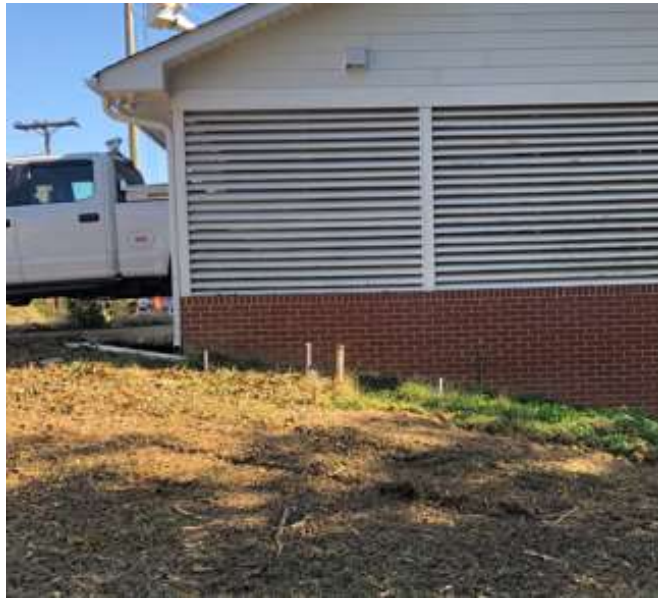
Heating Oil UST located adjacent to the west facing exterior wall of the single-family residential structure (11.16.2021)
