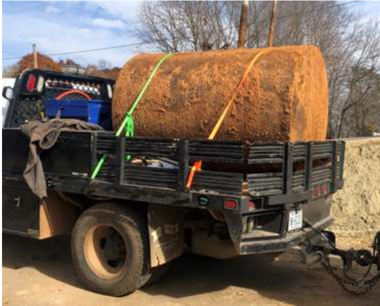
Transportation of Heating Oil UST by CERT (12.01.2021)
