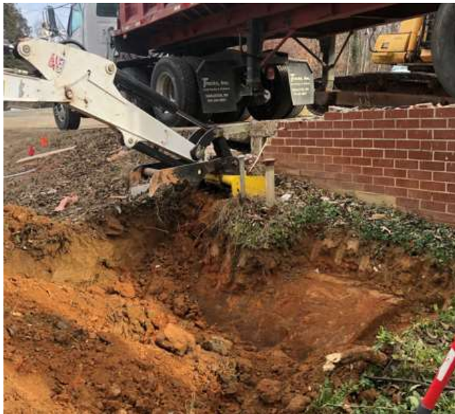
Uncovering the top of the Heating Oil UST (12.01.2021)
