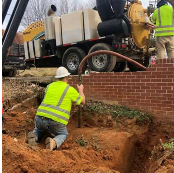
Vacuum extraction of Heating Oil UST contents prior to removal (12.01.2021)
