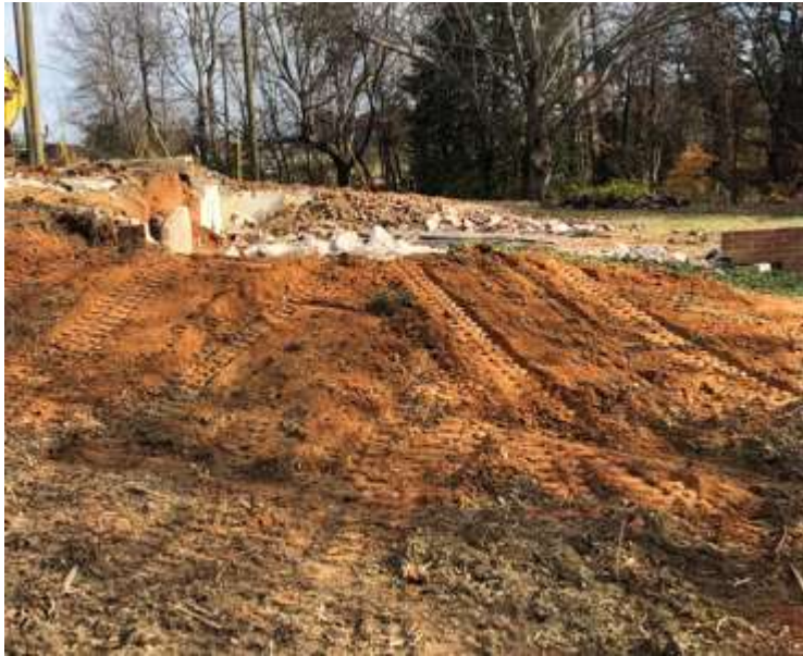
View of former Heating Oil UST location upon site departure (12.01.2021)
