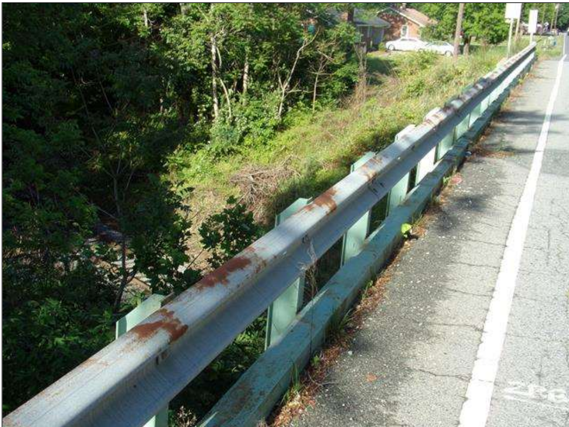
South bridge rail (North bridge rail similar)
