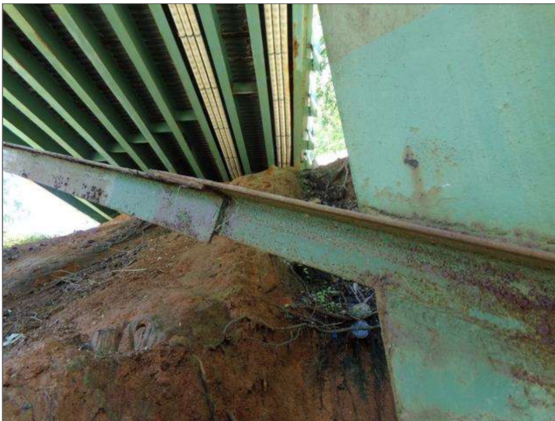
BENT 1 PILE 1: 2' REPAIRED CROSS BRACING ANGLE ON EAST BRACING CONNECTION.
