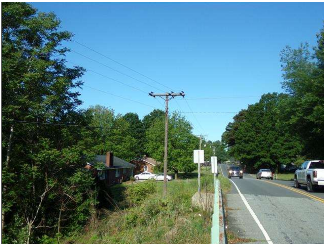
Overhead utilities on South and West sides of bridge
