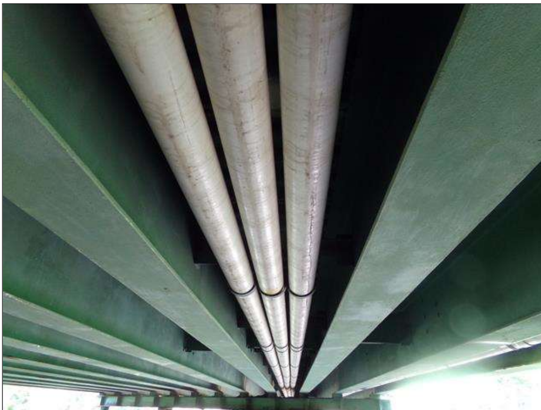
(3) 4" diameter utilities in Bay 3
