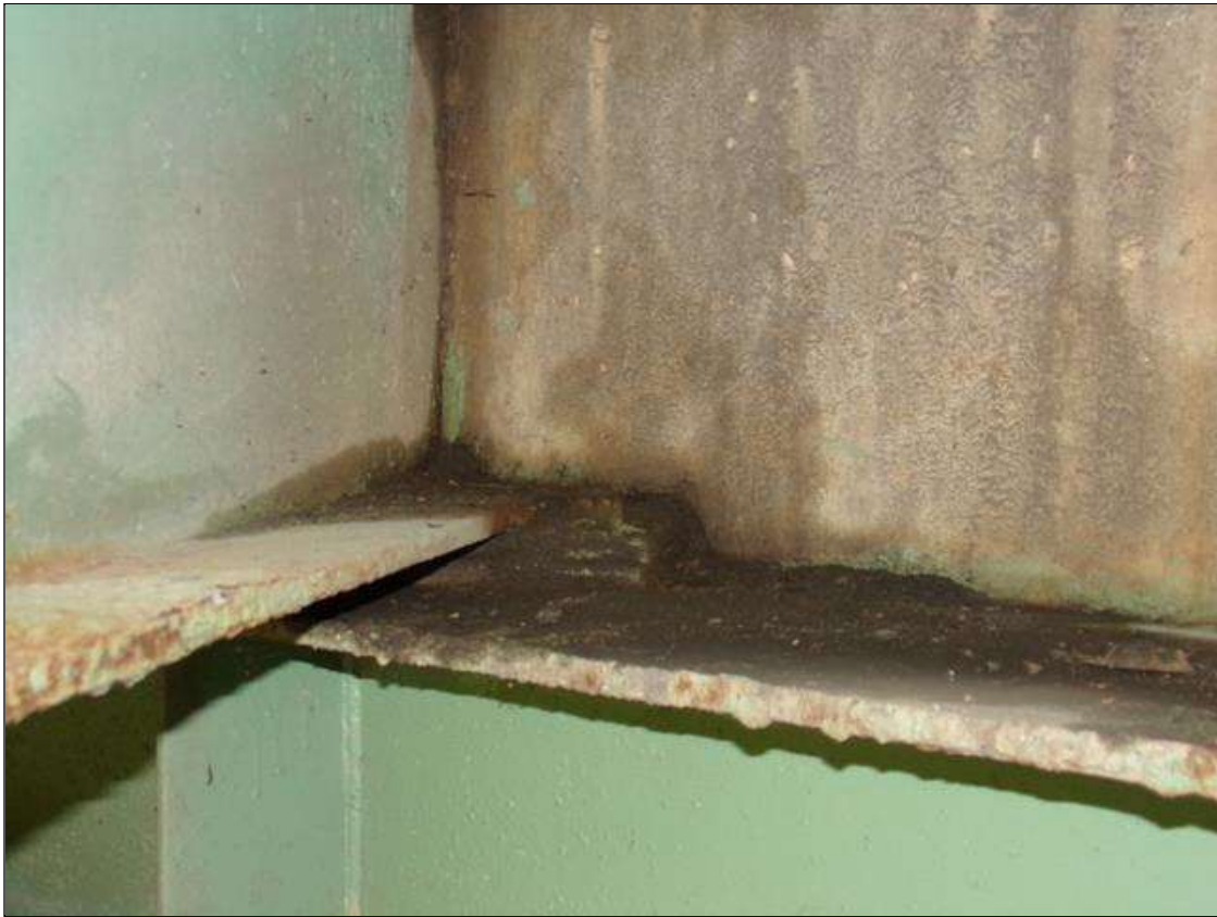
End Bent bearing (Beam 10, End Bent 2 shown)
