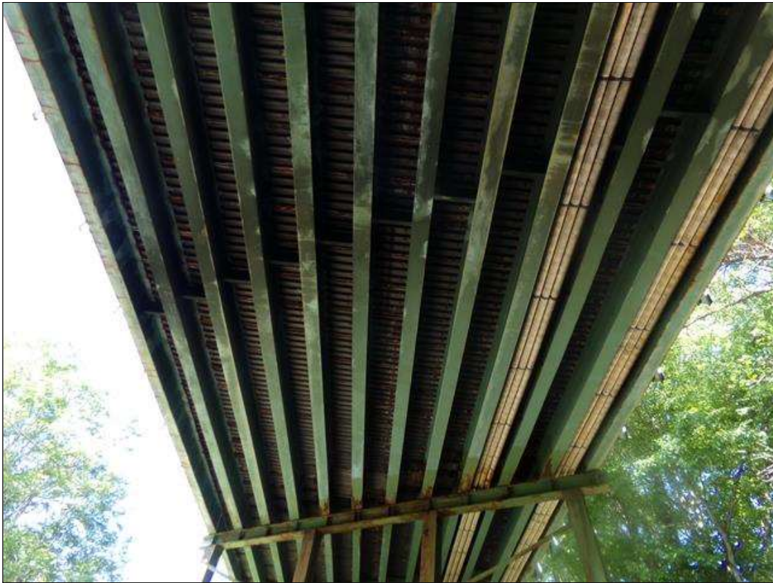
Underside of superstructure (Span 2 shown)
