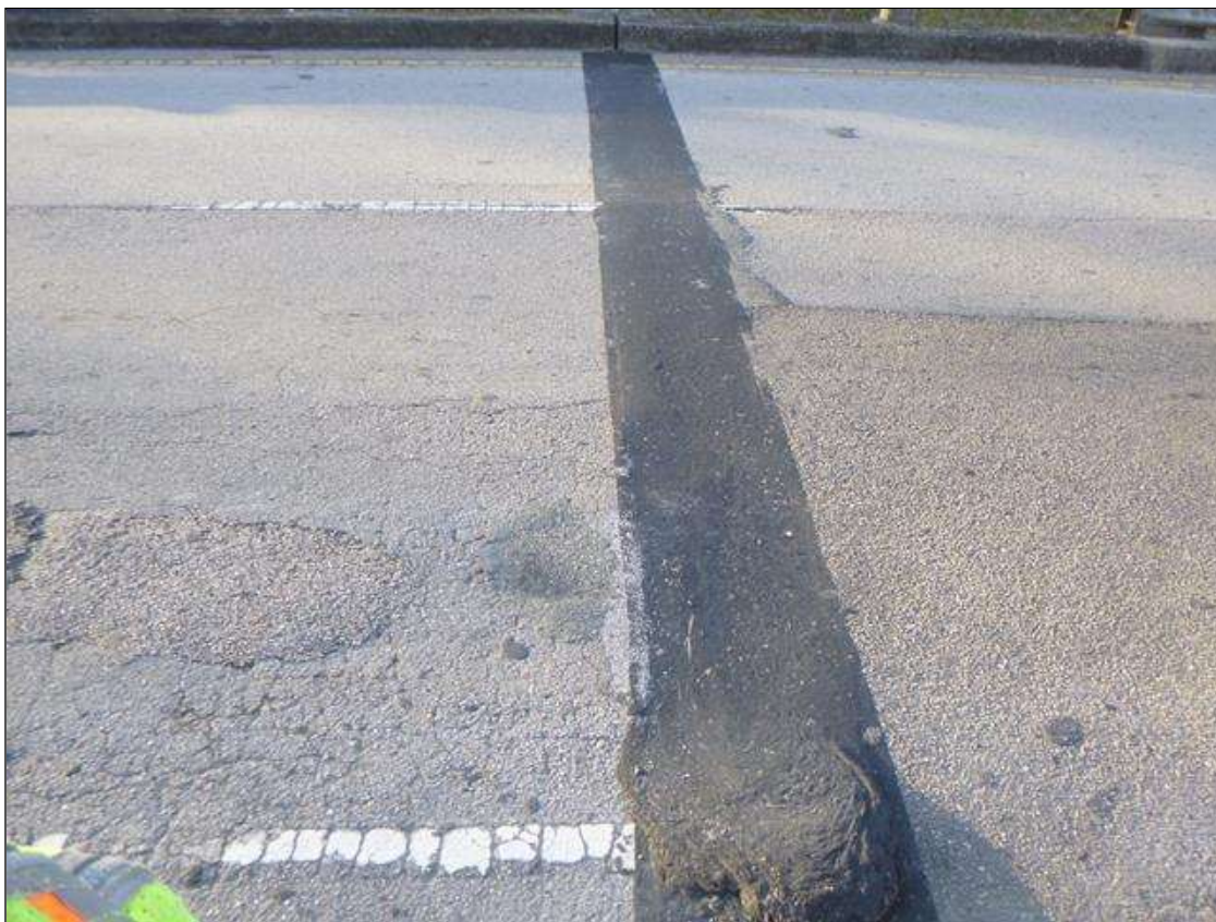
ASPHALT WEARING SURFACE OVER BENT 2 LOOKING WEST
