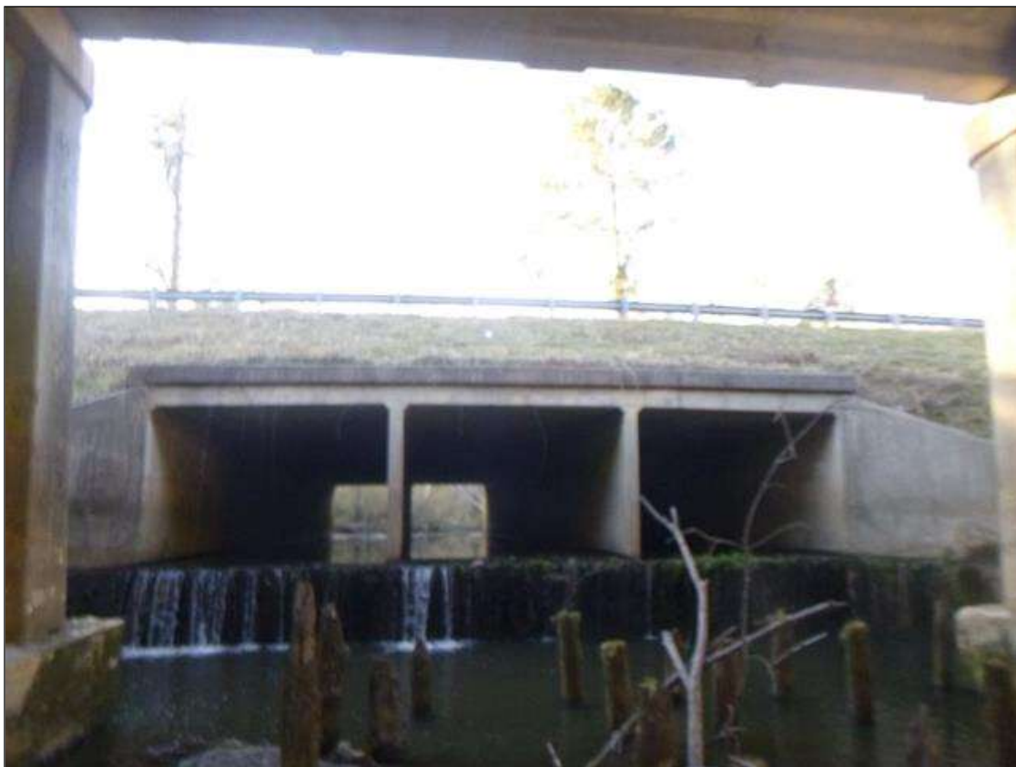
UPSTREAM VIEW LOOKING WEST
