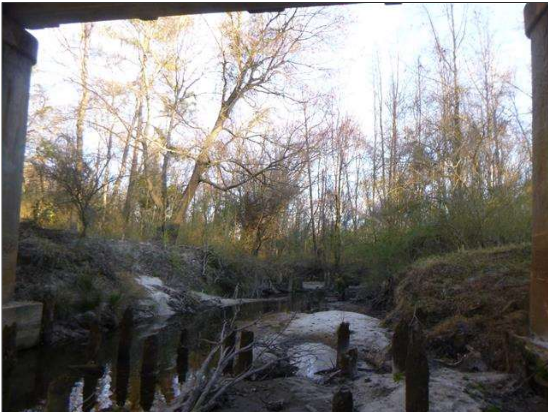
DOWNSTREAM VIEW LOOKING EAST
