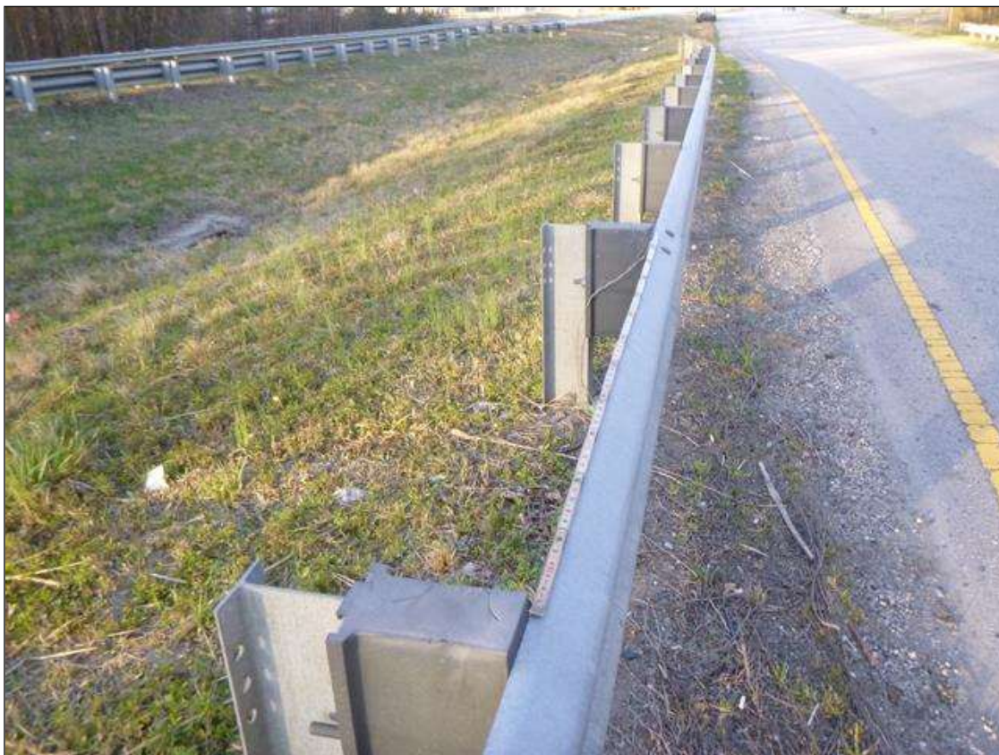
NORTHWEST TYPICAL GUARDRAIL POST SPACING 75" (OTHERS SIMILAR)
