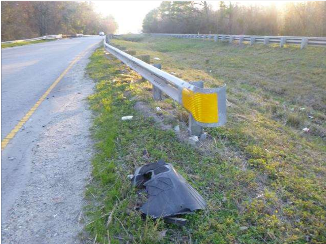
NORTHWEST GUARDRAIL TERMINAL, NORTHEAST SIMILAR
