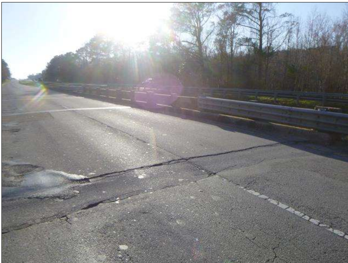
WEST BRIDGE RAIL
