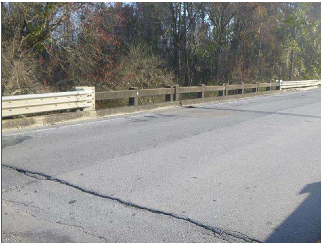
EAST BRIDGE RAIL
