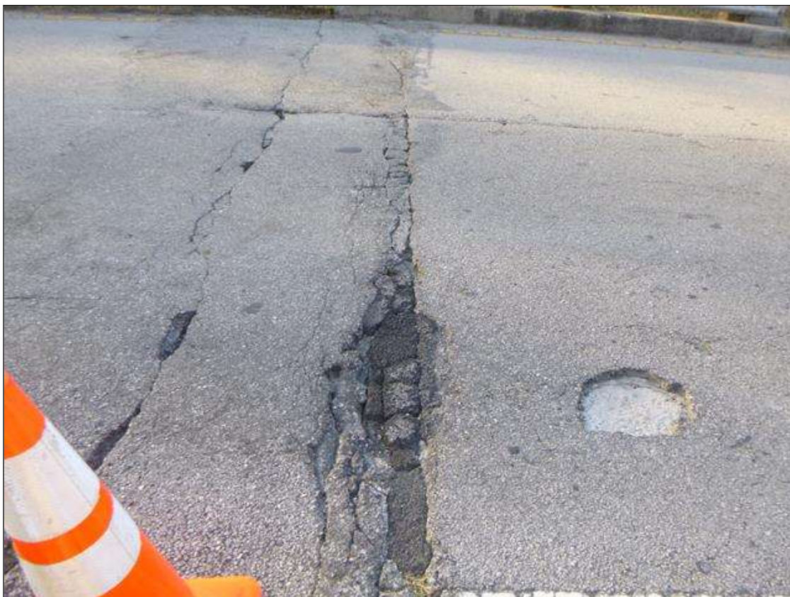
ASPHALT WEARING SURFACE OVER END BENT 1 LOOKING WEST
