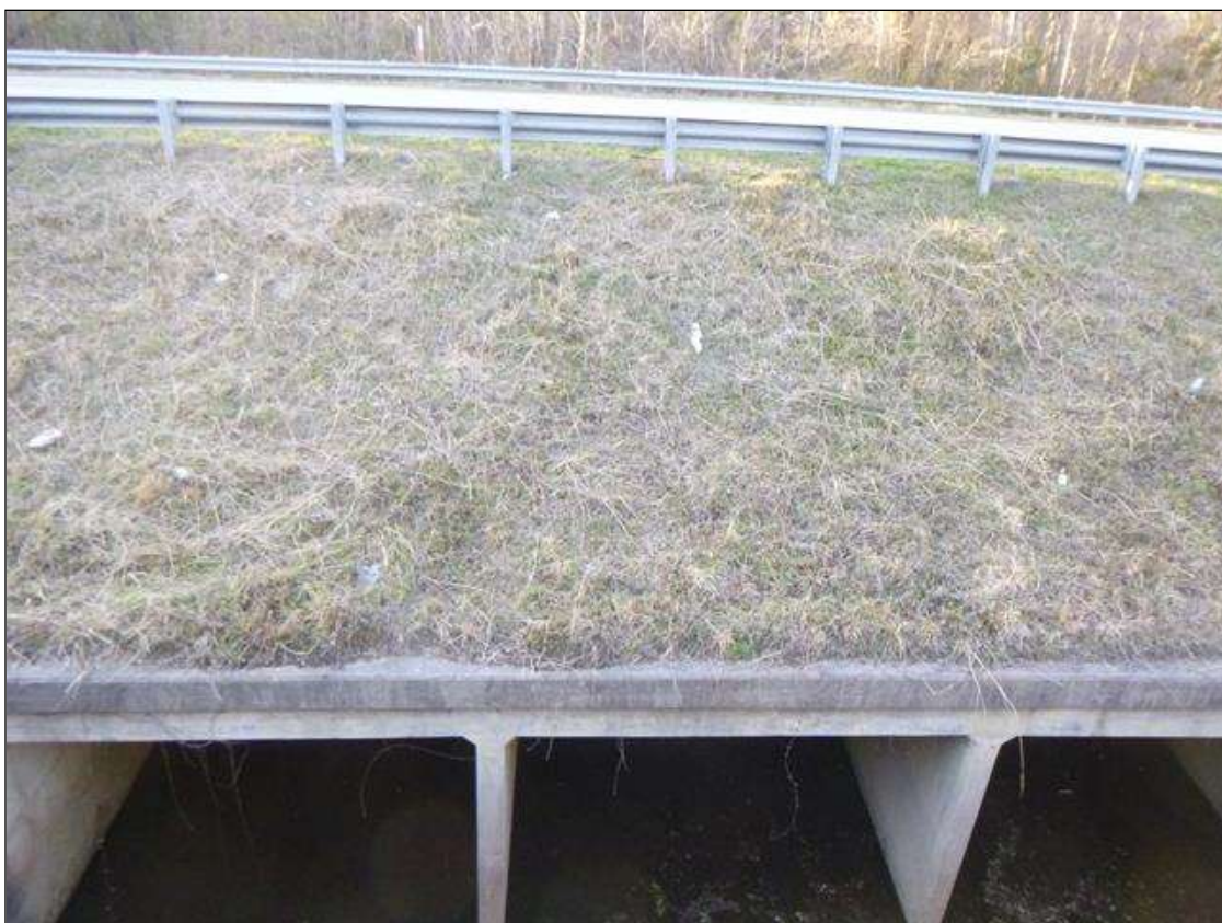
UPSTREAM VIEW FROM BRIDGE LOOKING WEST
