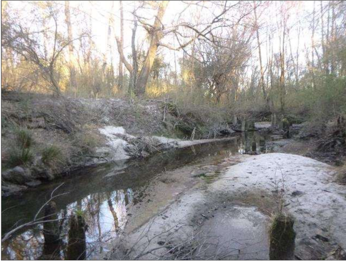
WATERWAY ADEQUACY: BANK EROSION ON BOTH EMBANKMENTS AT DOWNSTREAM SIDE OF BRIDGE DUE TO HIGH WATER EVENTS WITH FALLEN TREES ALONG BOTH BANKS
