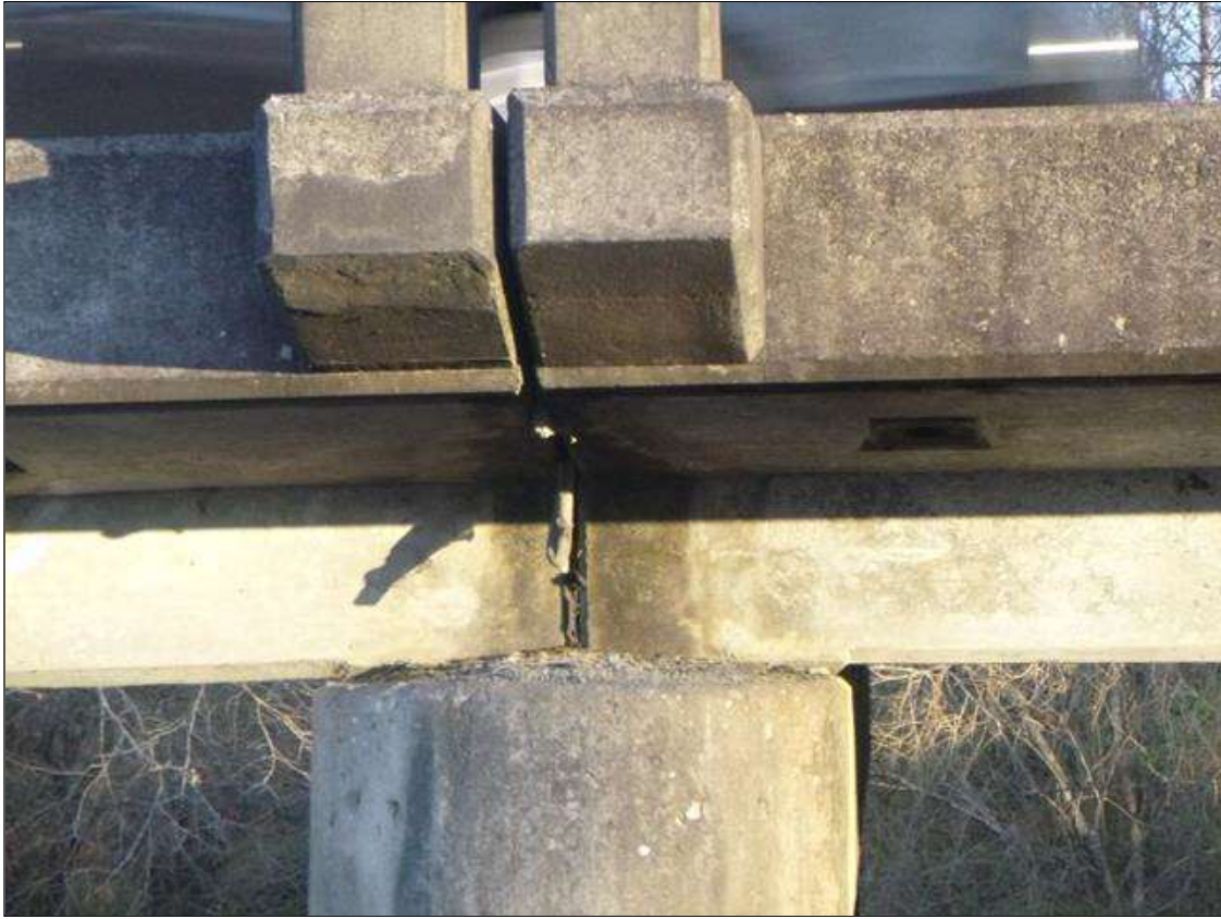
BEAM 1 BEARING OVER BENT 1 (OTHERS SIMILAR)
