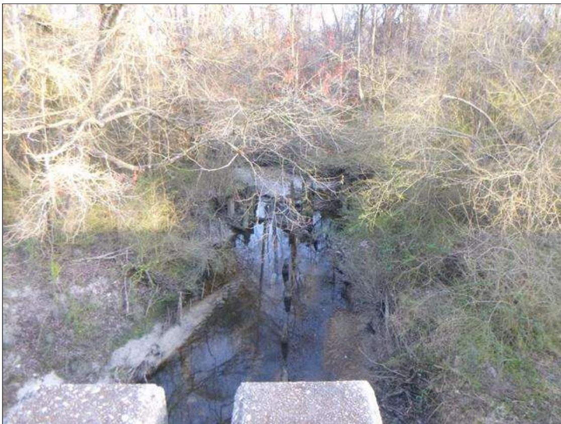
DOWNSTREAM VIEW FROM BRIDGE LOOKING EAST
