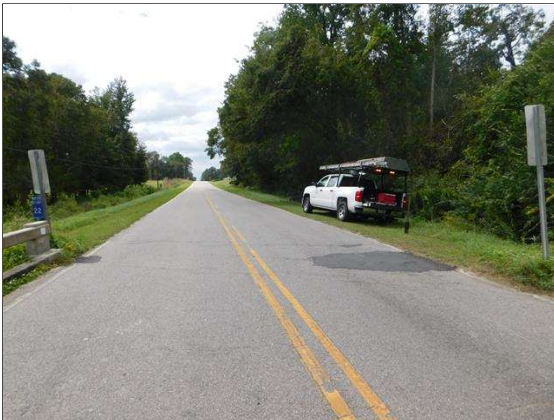
FROM BRIDGE LOOKING SOUTH
