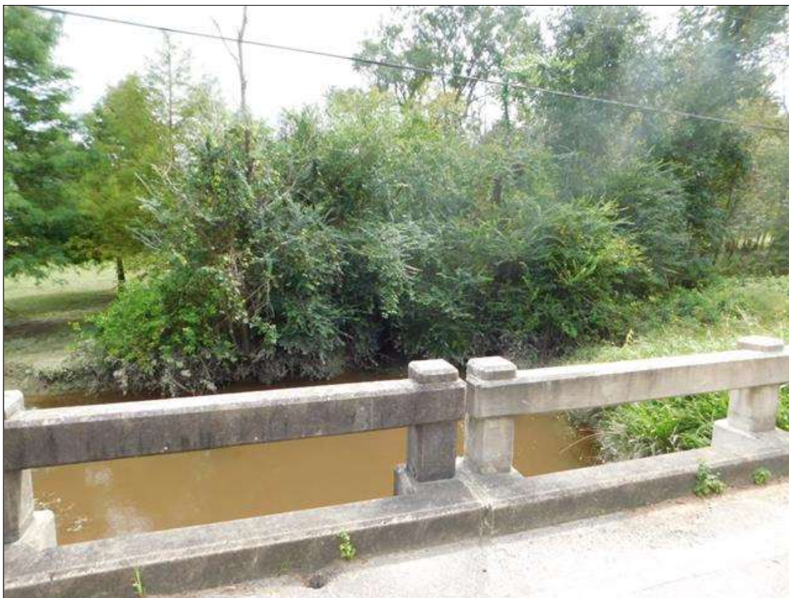
FROM BRIDGE LOOKING EAST UPSTREAM
