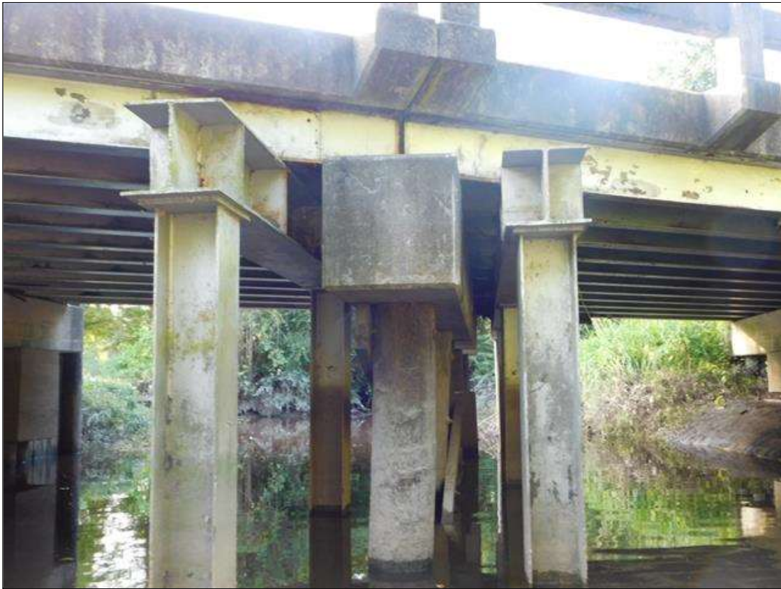
END OF BENT 1 AND CRUTCH BENT CAPS
