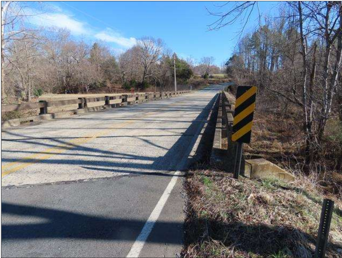
TYPICAL DELINEATOR, NEAR RIGHT (SW)
