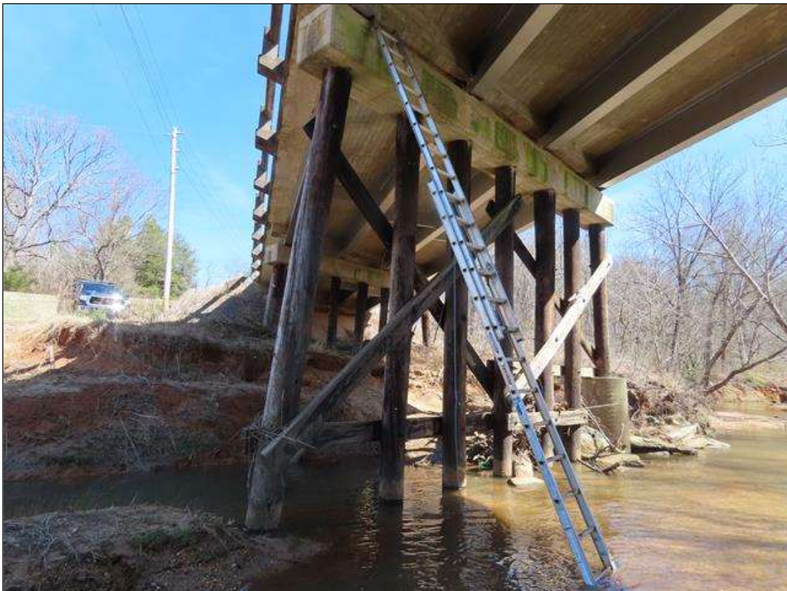
BENT 3, NEAR SIDE
