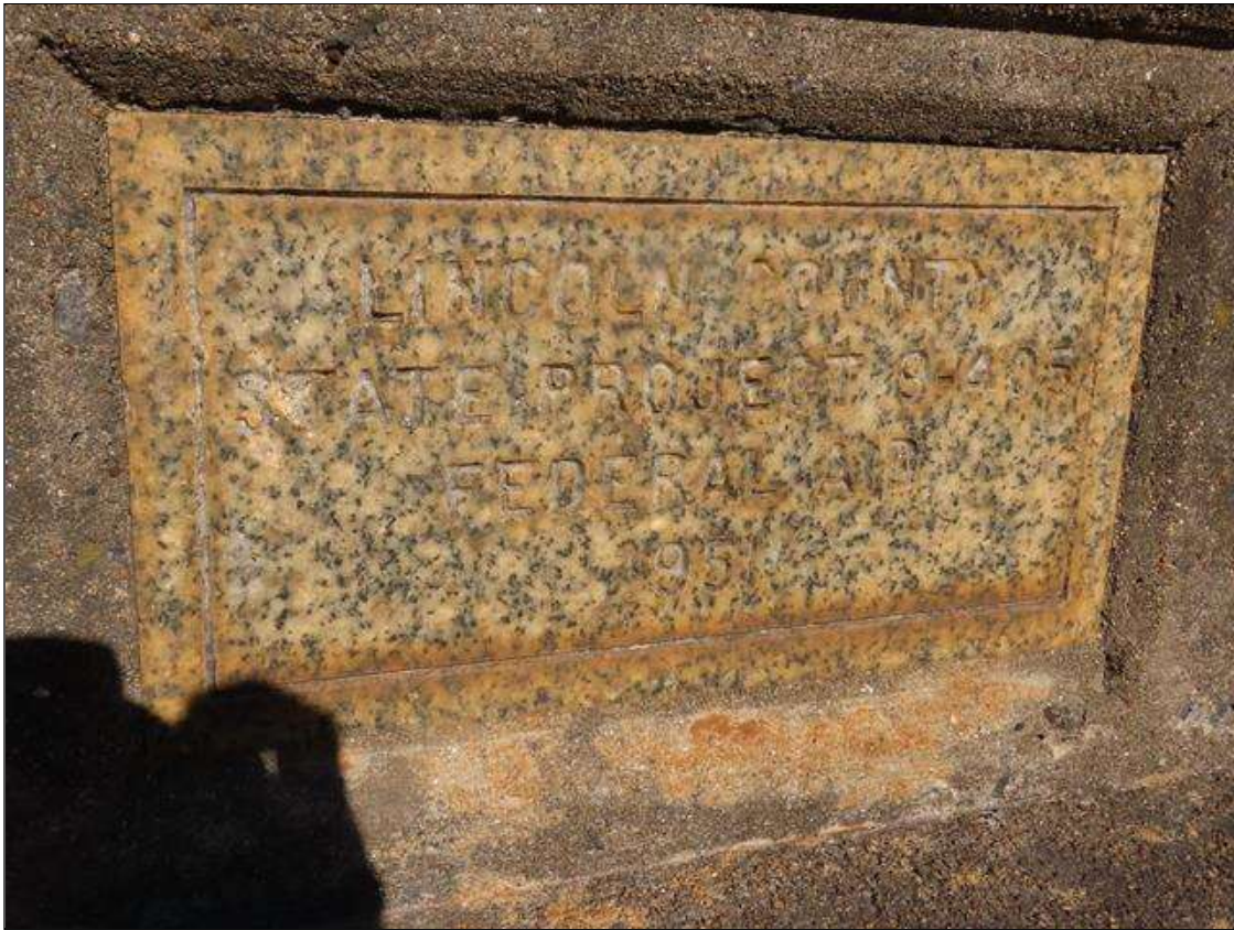
BRIDGE PLAQUE, FAR LEFT
