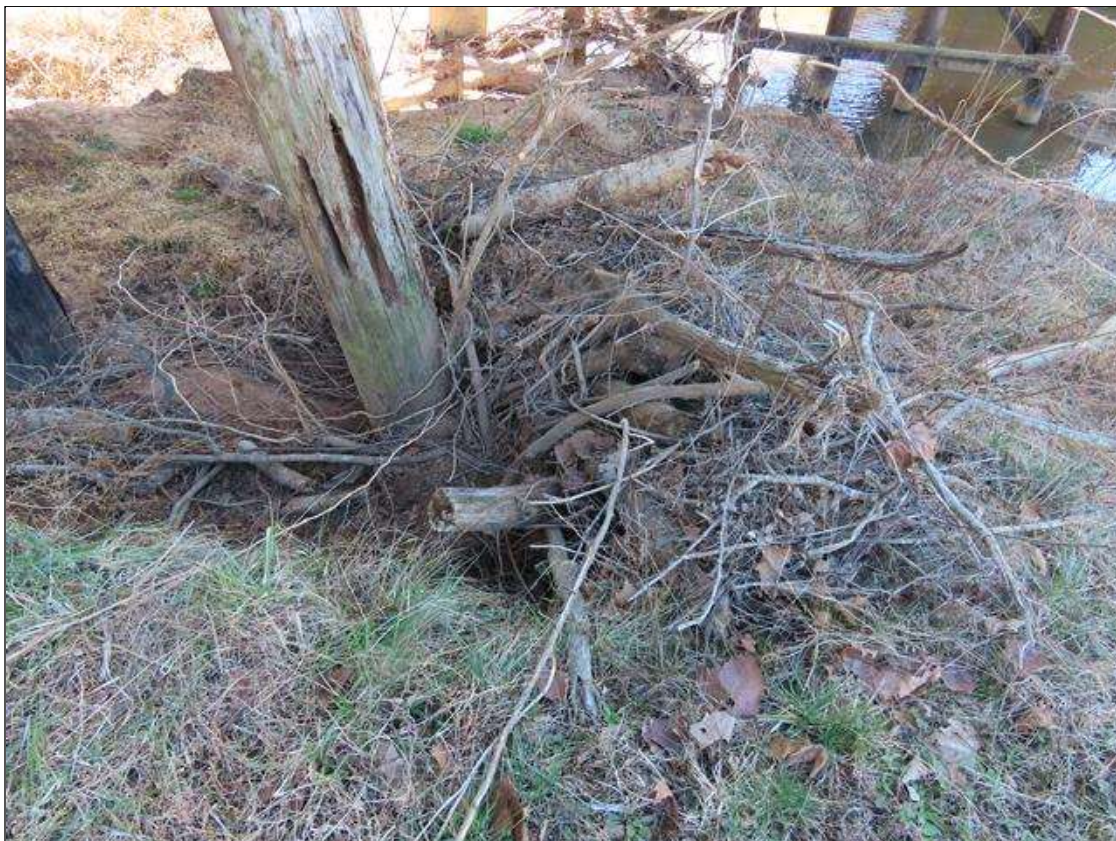
DRIFT (12CUFT) AT LEFT SIDE OF BENT 4 PILE 1
