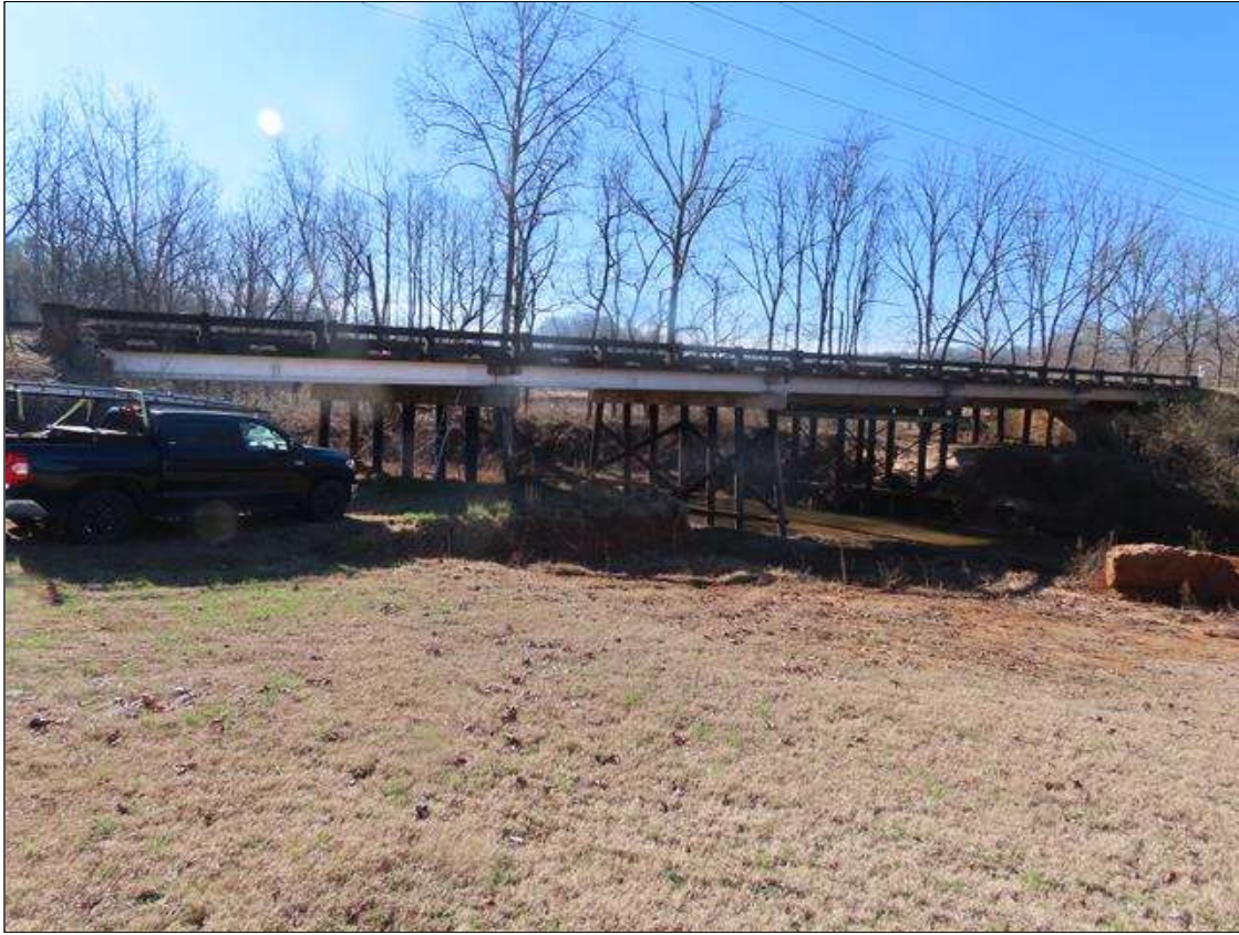
UPSTREAM ELEVATION, LOOKING BACK
