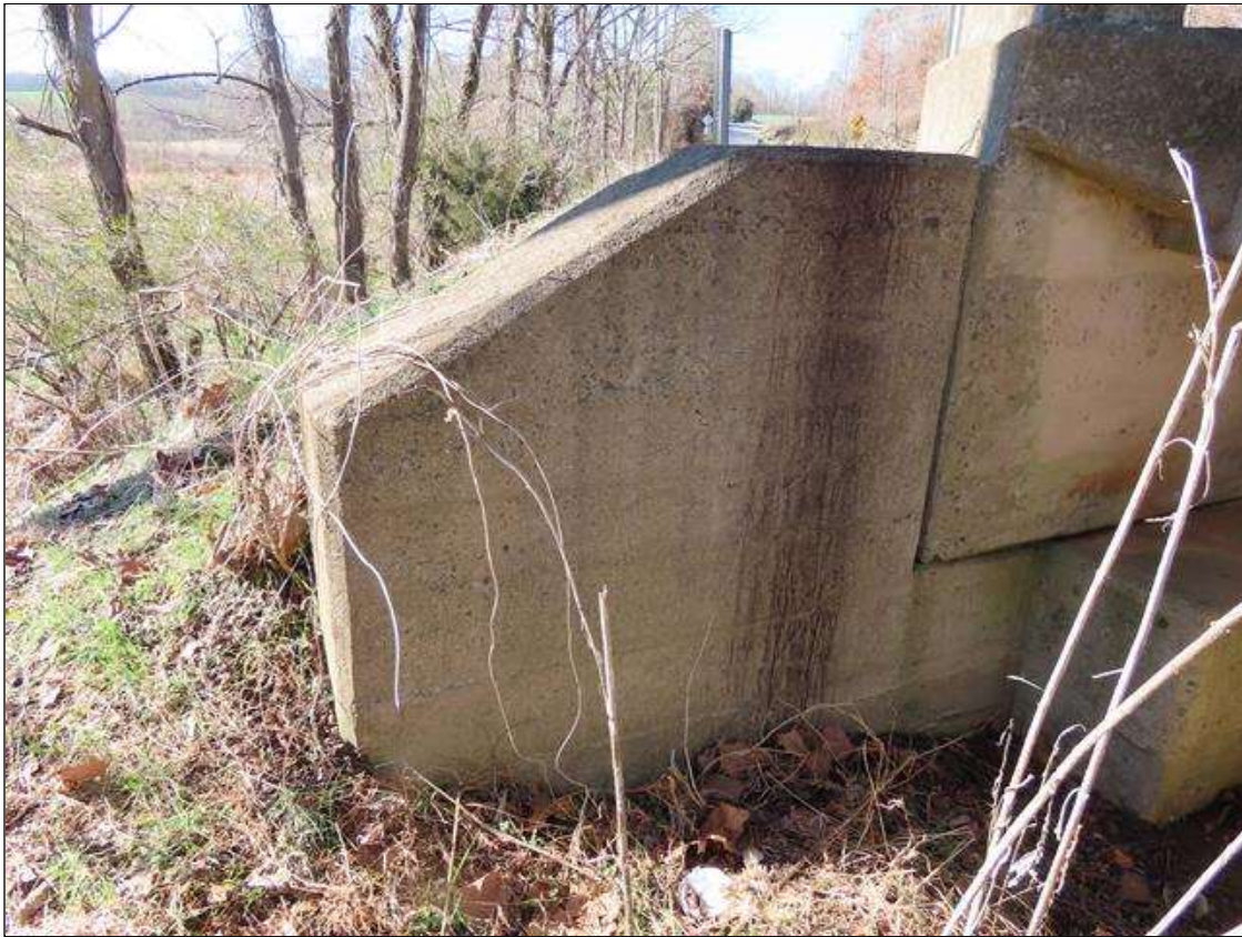
TYPICAL WINGWALL, NEAR RIGHT (SW)
