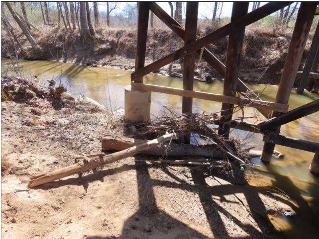
DRIFT (50CUFT) AT FAR SIDE OF BENT 3 AT DOWNSTREAM END
