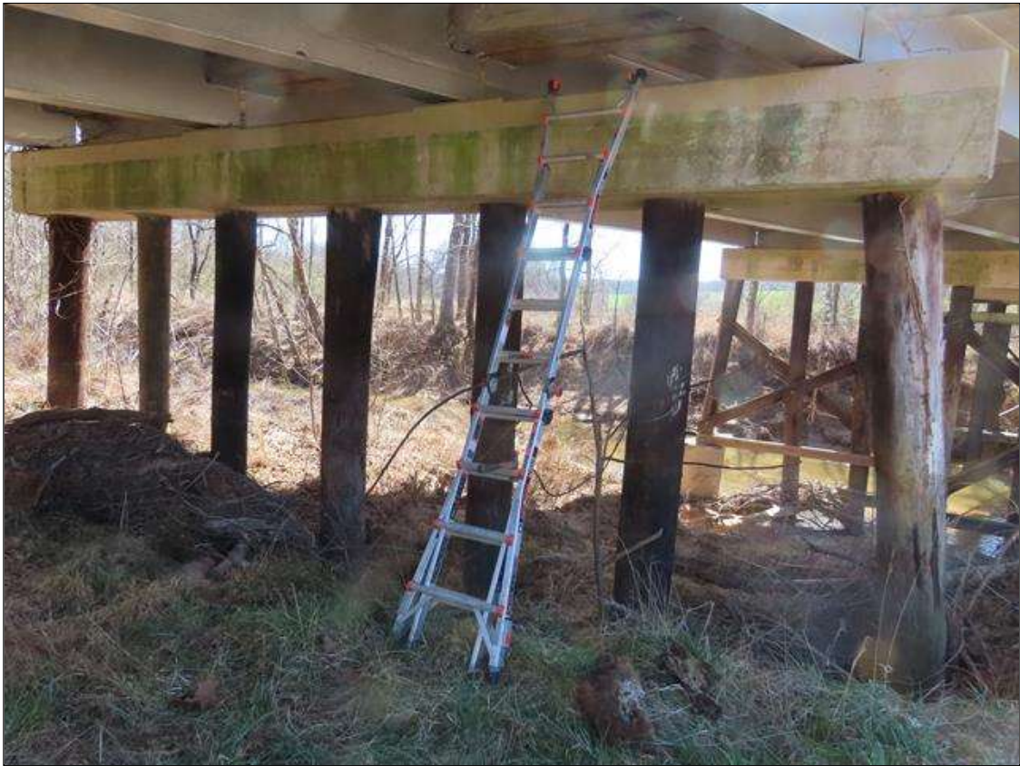
BENT 4, FAR SIDE
