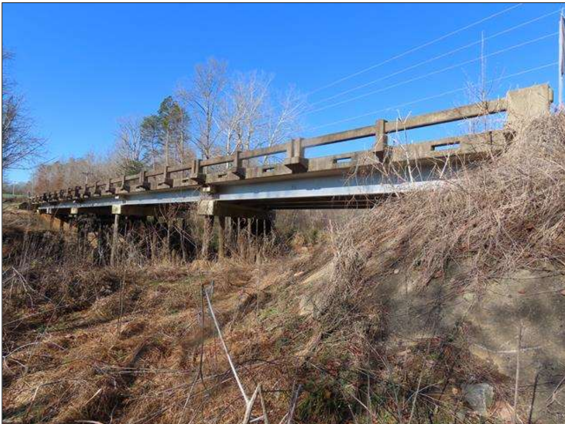
DOWNSTREAM ELEVATION, LOOKING BACK
