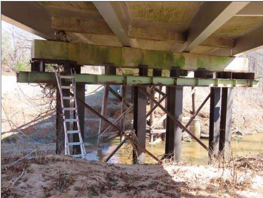
BENT 2, NEAR SIDE
