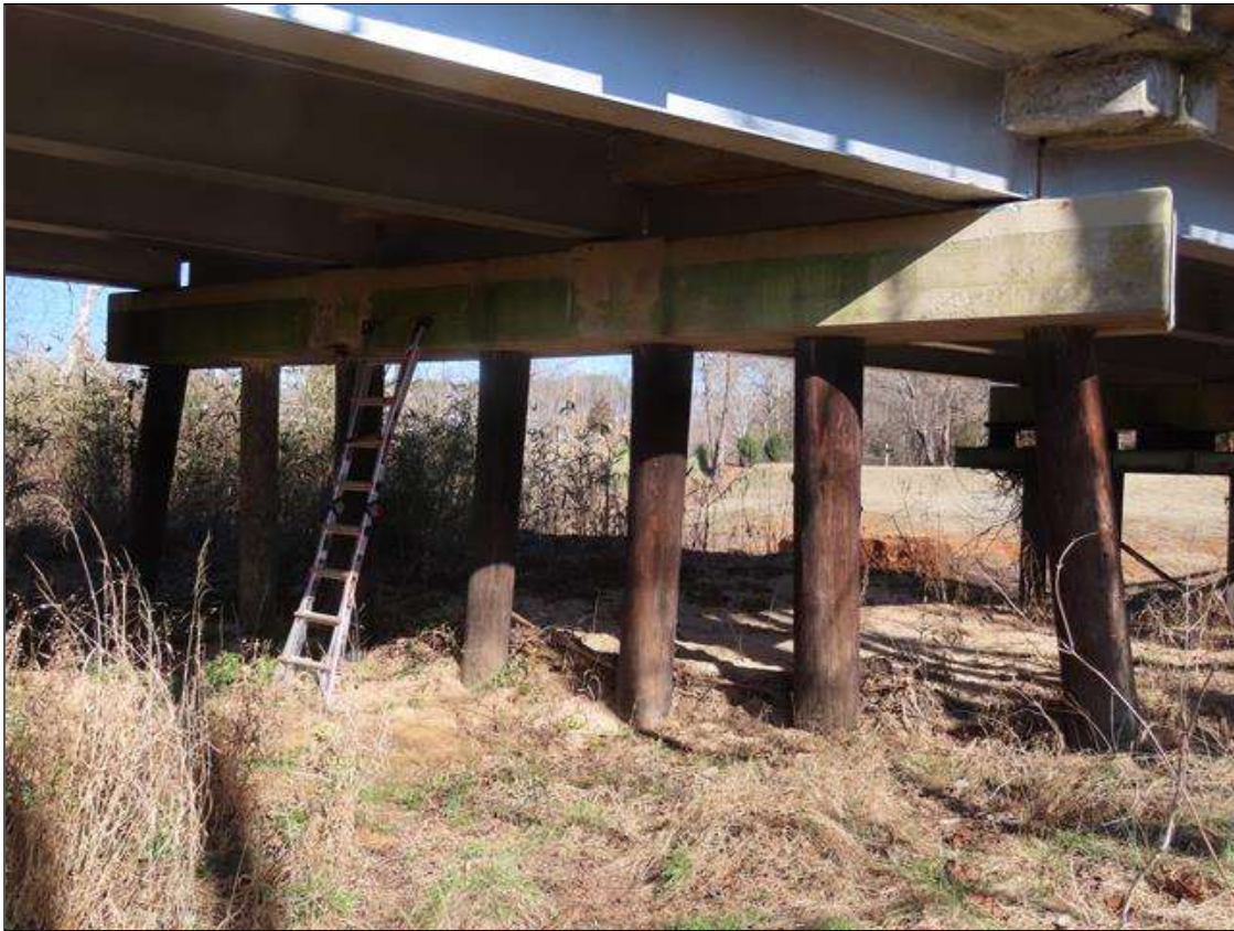
BENT 1, NEAR SIDE
