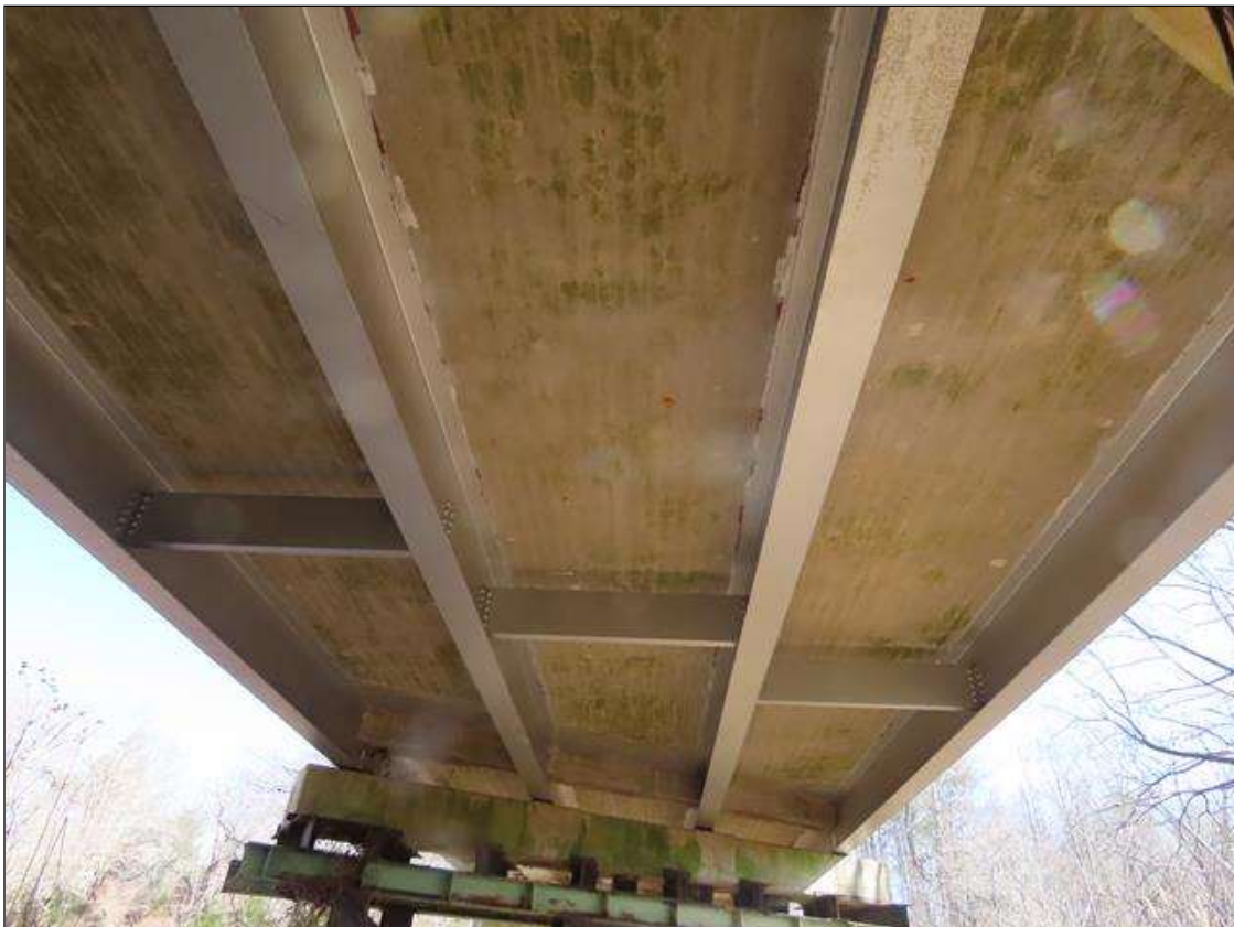
TYPICAL SUPERSTRUCTURE, SPAN 2 LOOKING AHEAD
