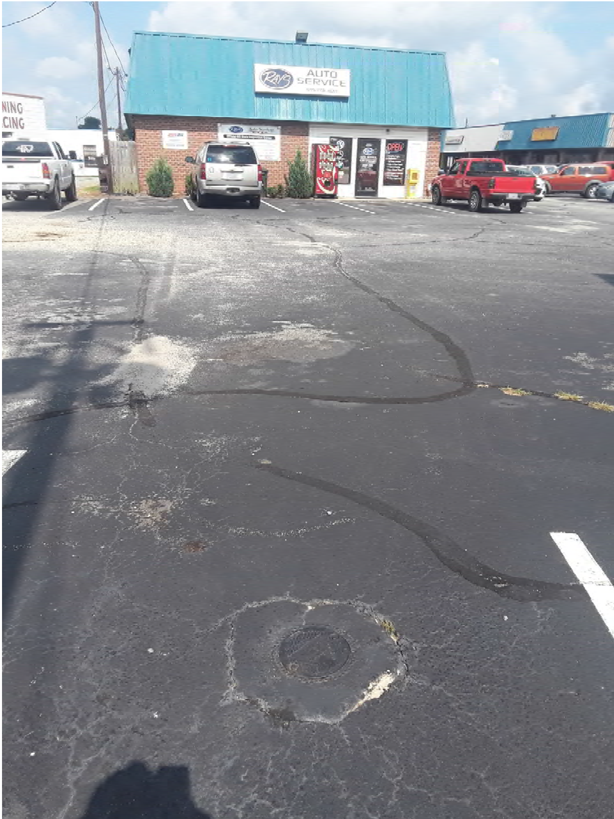
Photo 3 – A view of well MW-2 (not abandoned), looking northwest.
