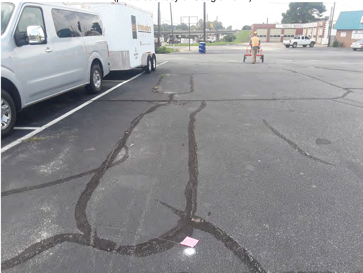
Photo 2 – Apparent former pump island area, looking southwest.
