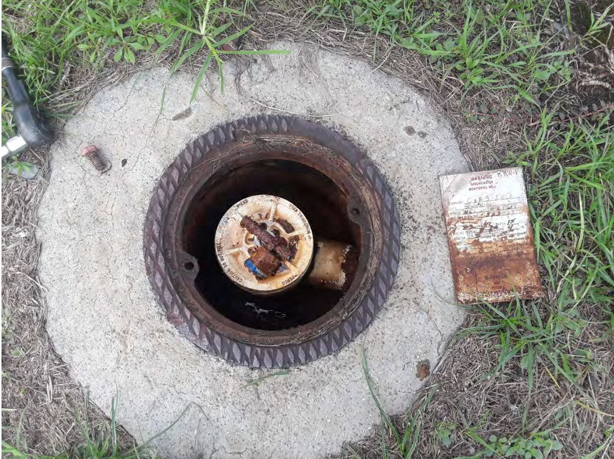
Photo 3 – A close-up view of well RMW-1 (not abandoned) – note horizontal pipe connected to well.
