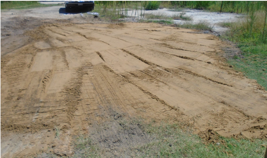
Photograph 8 – Backfilling and grading with clean soil.
