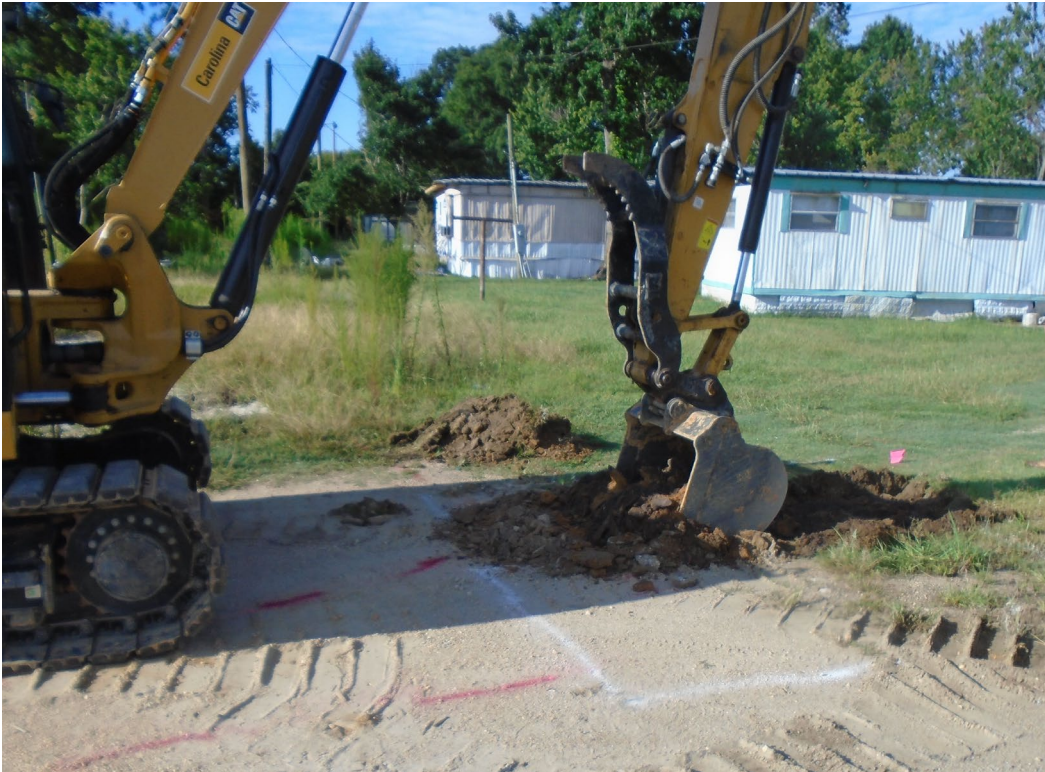
Photograph 2 – View of excavator removing the overburden.
