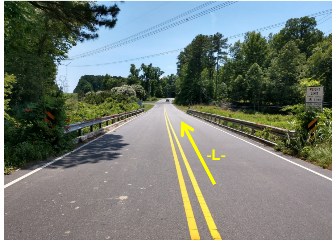
View of SR 2044 looking south.
