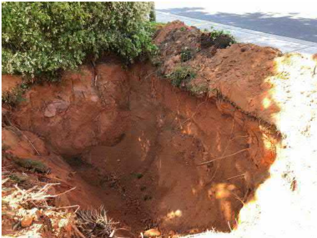
Photo 4 - View of interior of UST basin facing south
