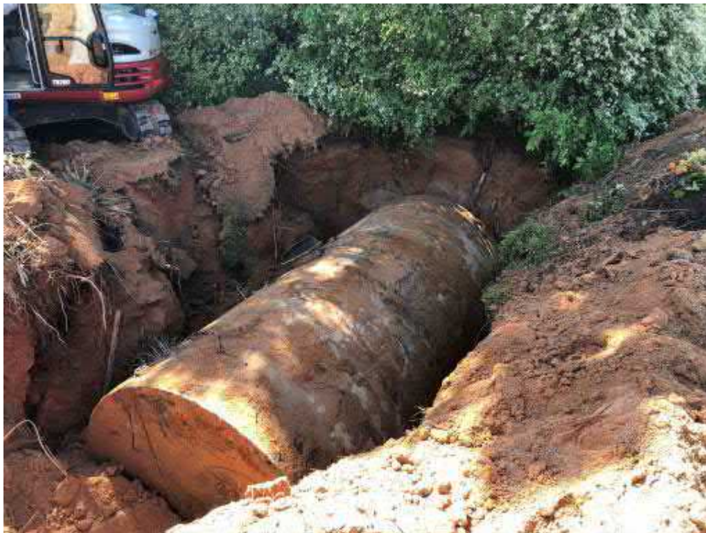
Photo 2 - Additional view of excavation facing east-southeast
