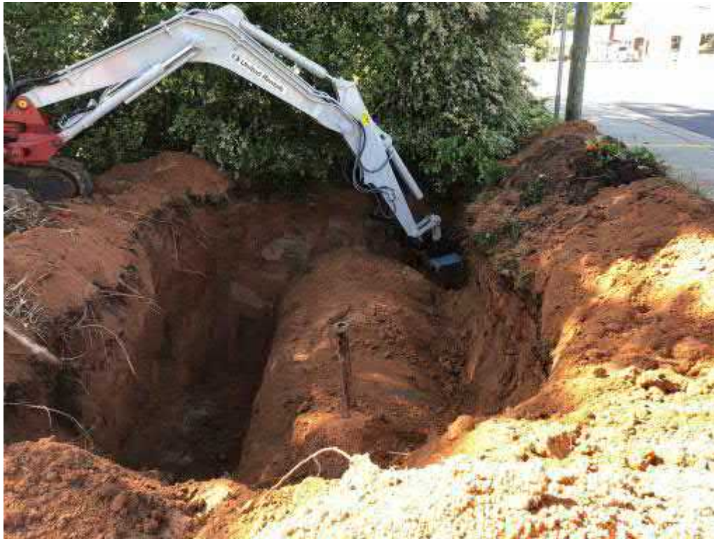
Photo 1 - View of excavation facing south-southeast
