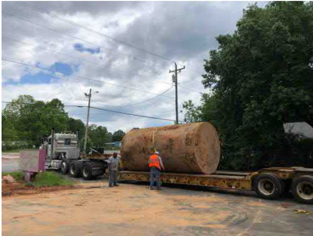
Photo 9 - View of UST being loaded onto tractor trailer for off-site disposal
