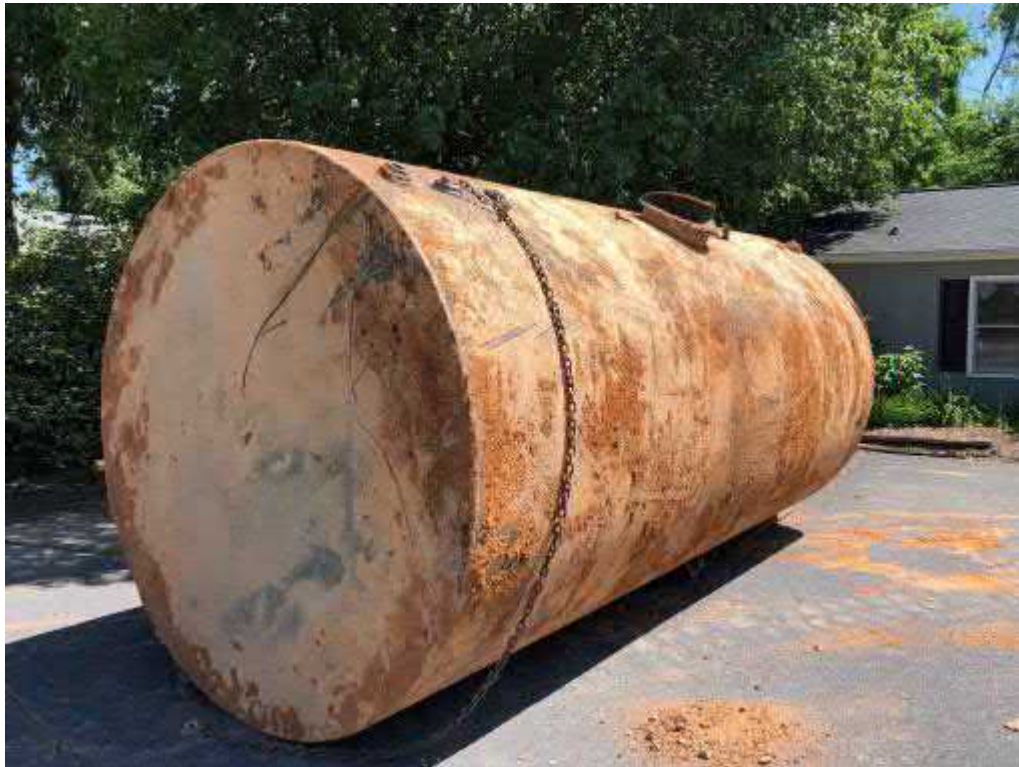
Photo 7 - Additional view of 6,000-gallon UST after excavation
