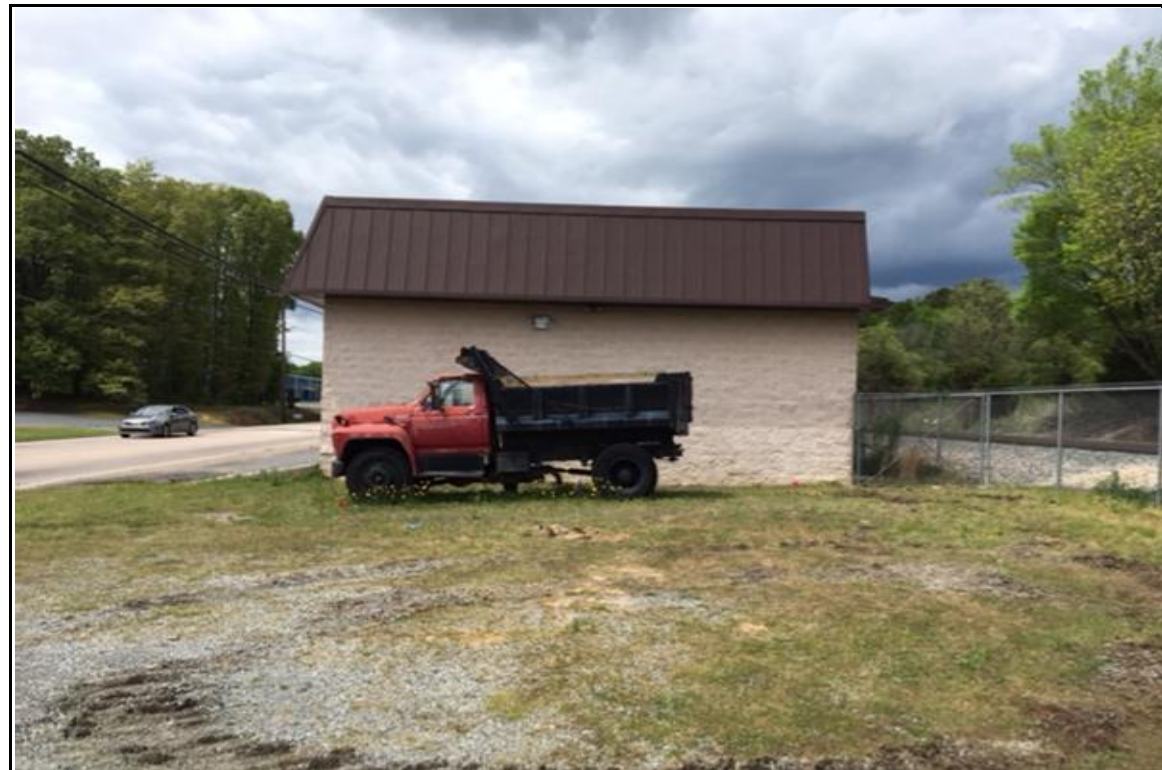
PHOTOGRAPH NO. 2: SOUTH OF -L- ALIGNMENT, LOOKING NORTH ACROSS INTERIOR BENT NO. 1
