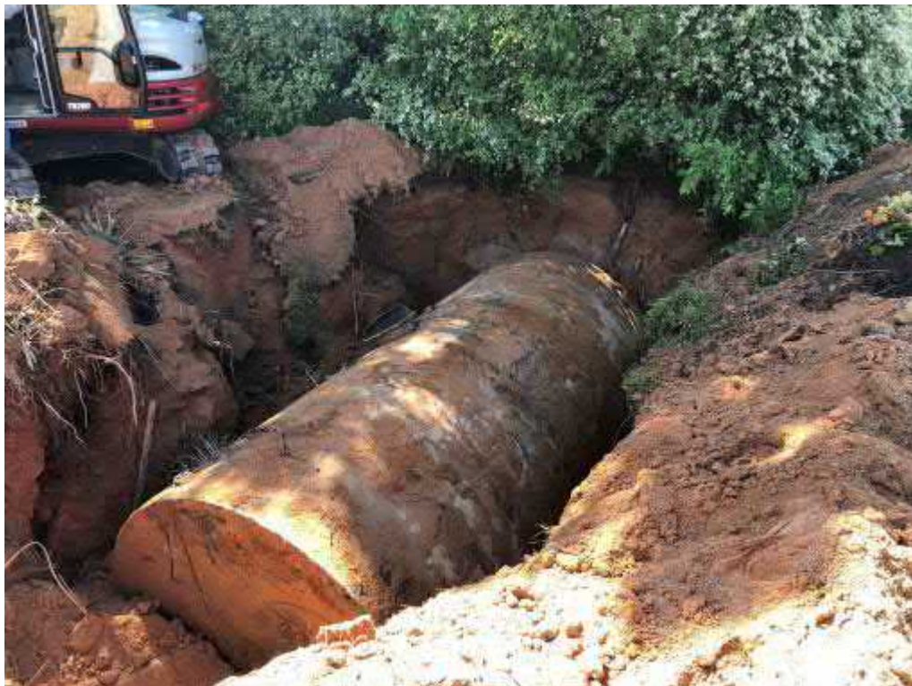
Photo 2 - Additional view of excavation facing east-southeast
