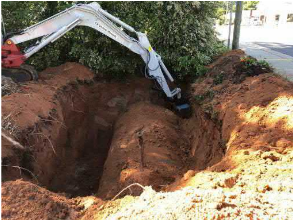
Photo 1 - View of excavation facing south-southeast
