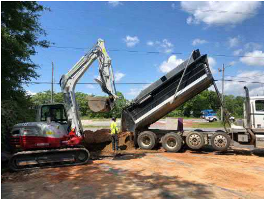
Photo 8 - View of backfilling of UST basin facing west
