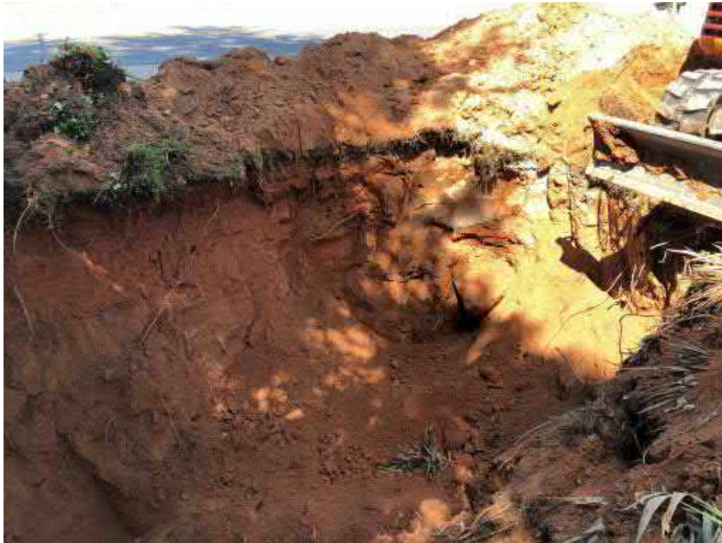
Photo 5 - View of interior of UST basin facing west
