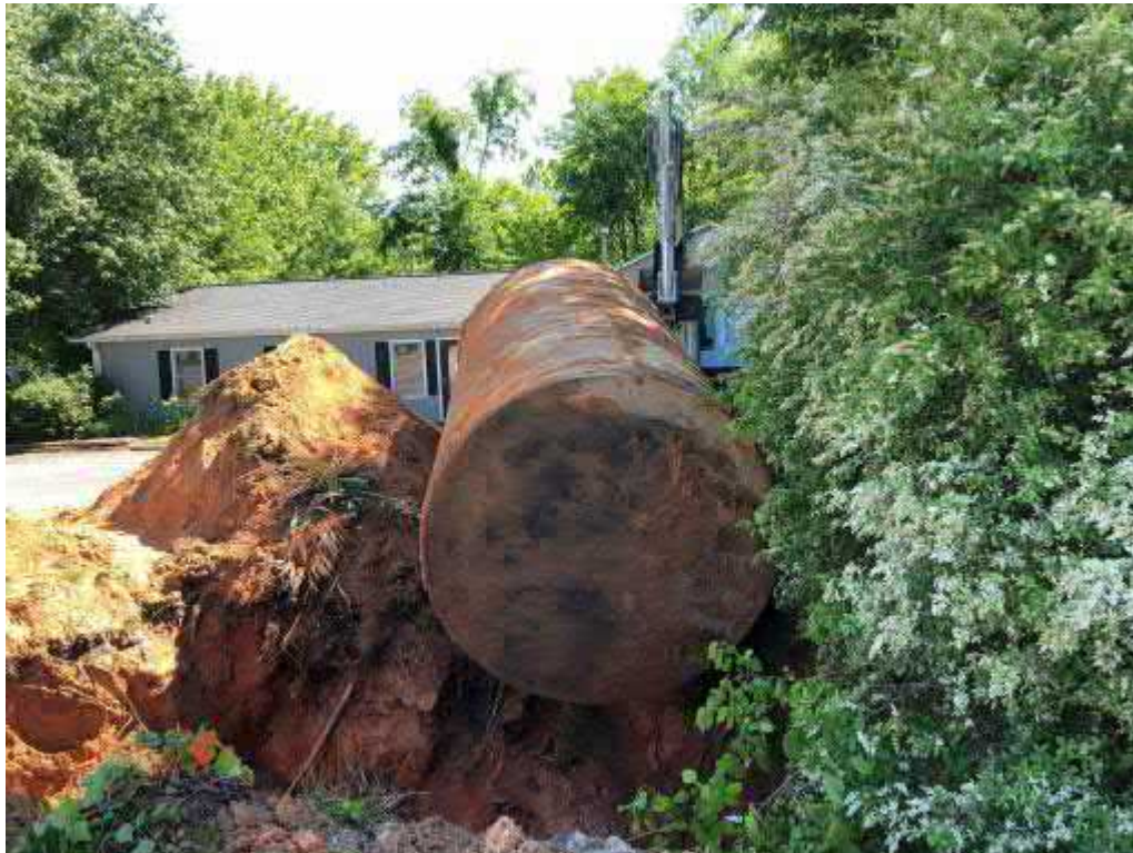
Photo 3 - View of UST being pulled from excavation
