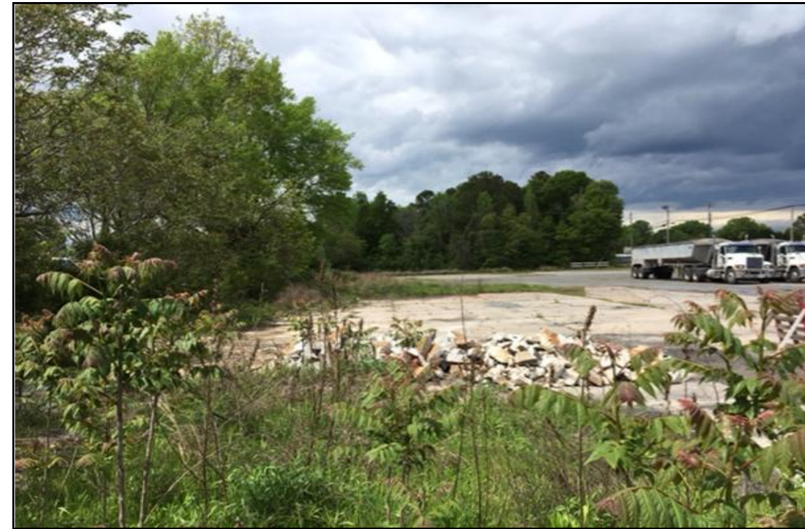
PHOTOGRAPH NO. 3: SOUTH OF -L- ALIGNMENT, LOOKING NORTH ACROSS INTERIOR BENT NO. 2
