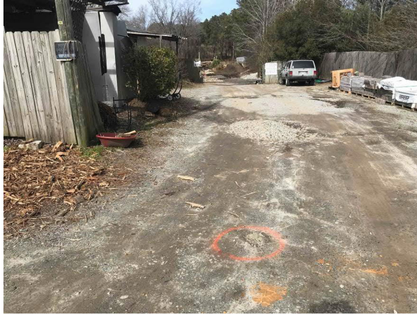
Photo #3 View of the eastern portion of the site; facing north.
