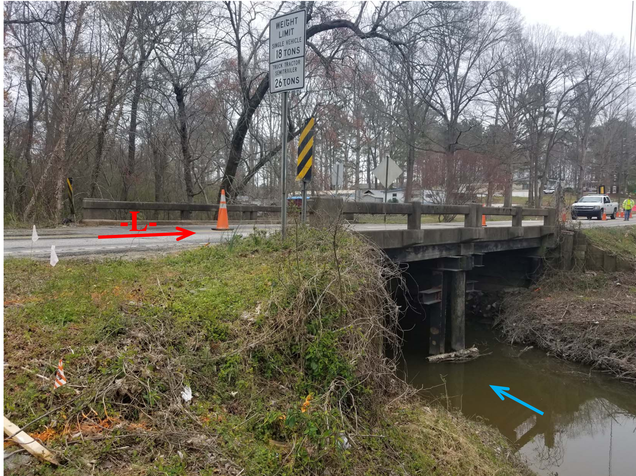
Looking Southeast towards End Bent 2
