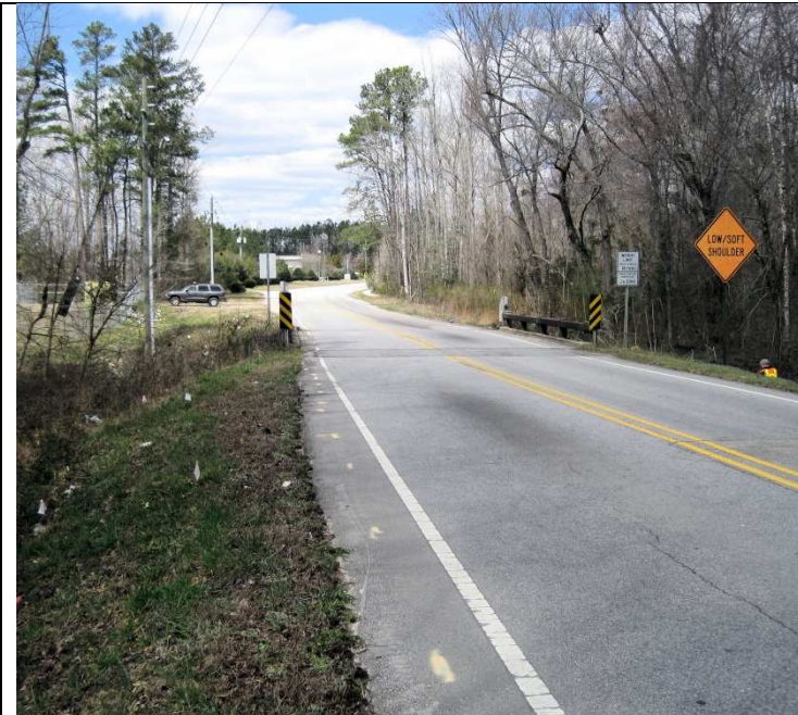
Bridge 247 on SR 2555 (Raynor Road). View to the northwest.
