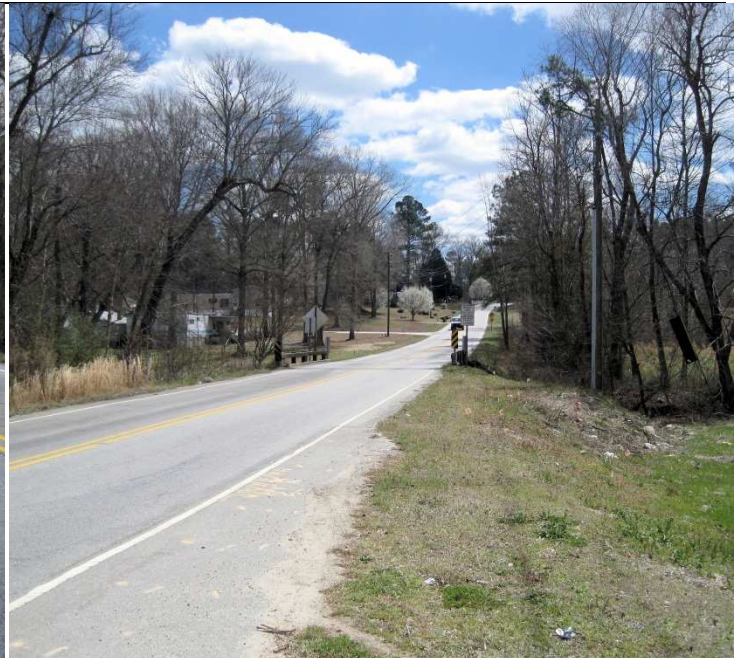
Bridge 247 on SR 2555 (Raynor Road). View to the southeast.
