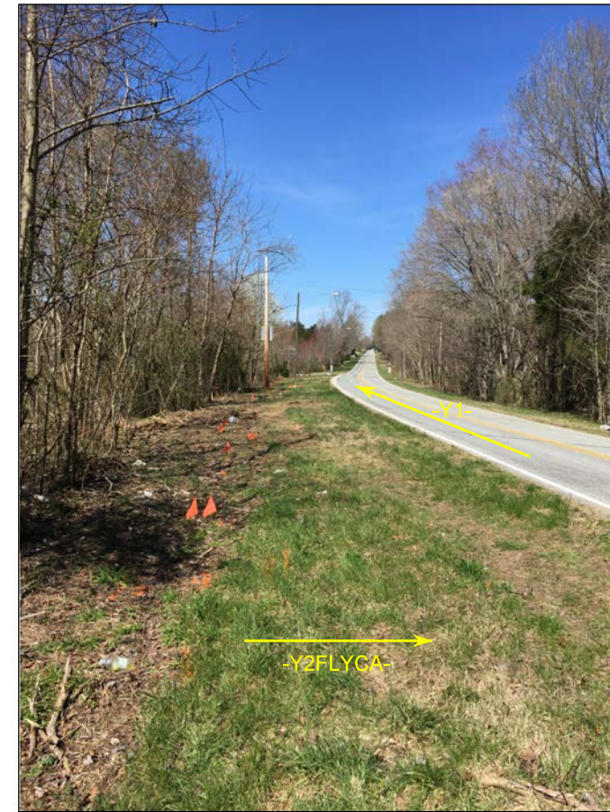
PHOTO 2: VIEW AT END BENT 2 LOOKING DOWNSTATION ALONG -Y1- (EXISTING HIGH POINT ROAD)
