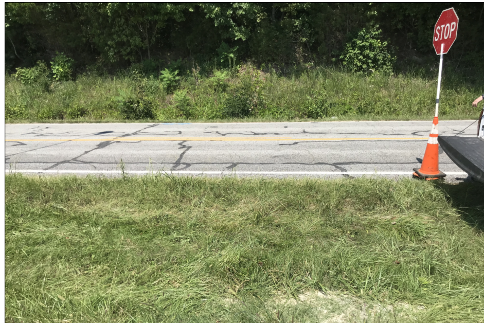
VIEW ALONG END BENT 1 FROM EB1-B TOWARD EB1-A
