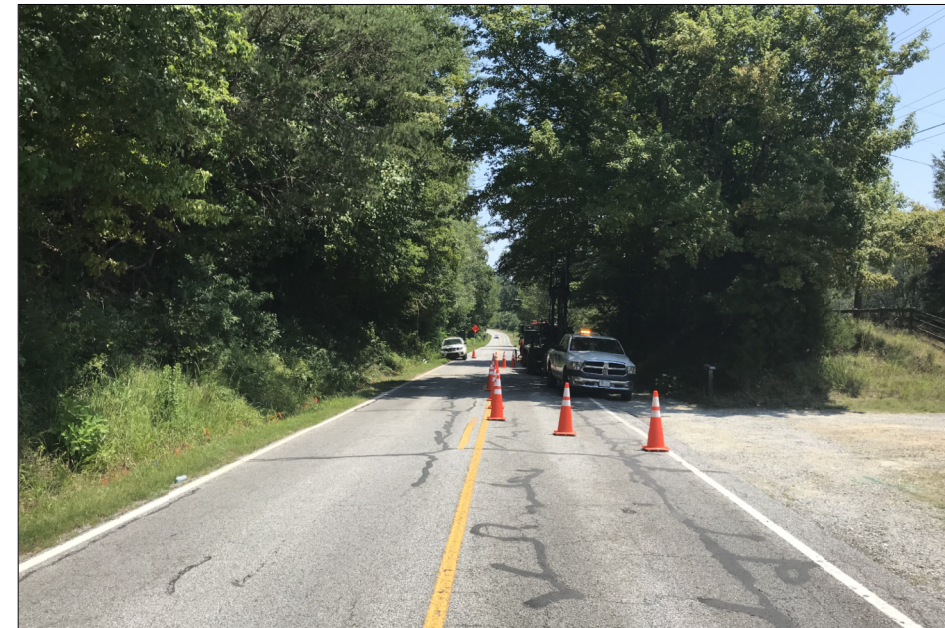
VIEW UPSTATION FROM END BENT 1 TOWARD END BENT 2
