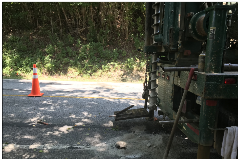
VIEW ALONG END BENT 2 FROM EB2-B TOWARD EB2-A
