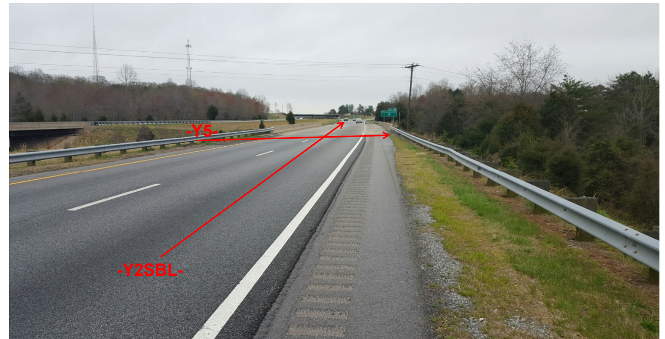
View Looking Southeast along -Y2SBL- from End Bent No. 1
