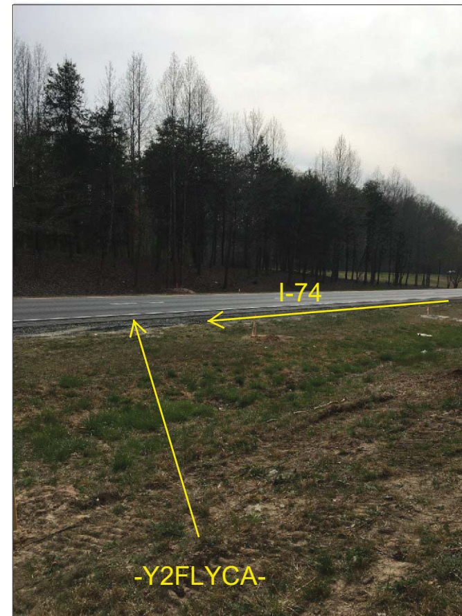
PHOTO 3: VIEW AT END BENT 2 LOOKING DOWNSTATION ALONG -Y2FLYCA- TOWARD EB-1
