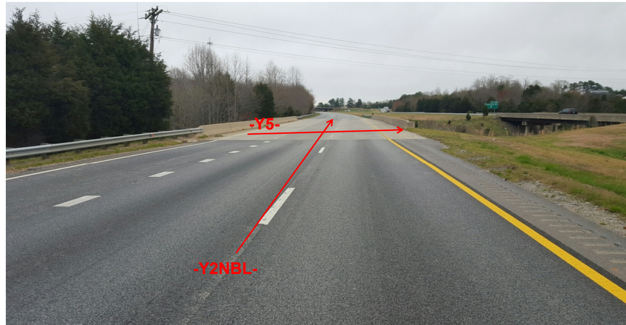
View Looking Southeast along -Y2NBL- from End Bent No. 1
