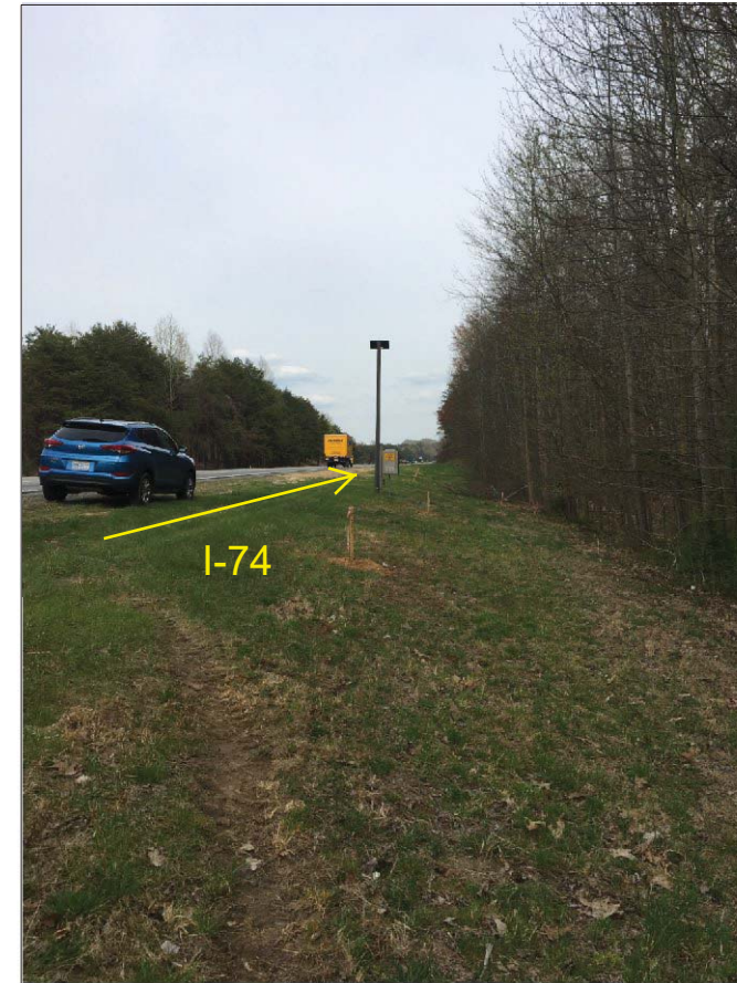
PHOTO 2: VIEW AT END BENT 1 LOOKING EAST ALONG -Y2- (EXISTING I-74)
