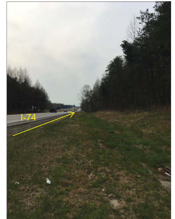
PHOTO 4: VIEW AT END BENT 2 LOOKING WEST ALONG -Y2- (EXISTING I-74)
