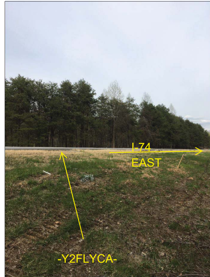
PHOTO 1: VIEW AT END BENT 1 LOOKING UPSTATION ALONG -Y2FLYCA- TOWARD EB-2
