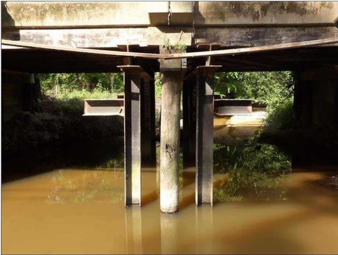
Pier 1 and crutch bents side view
