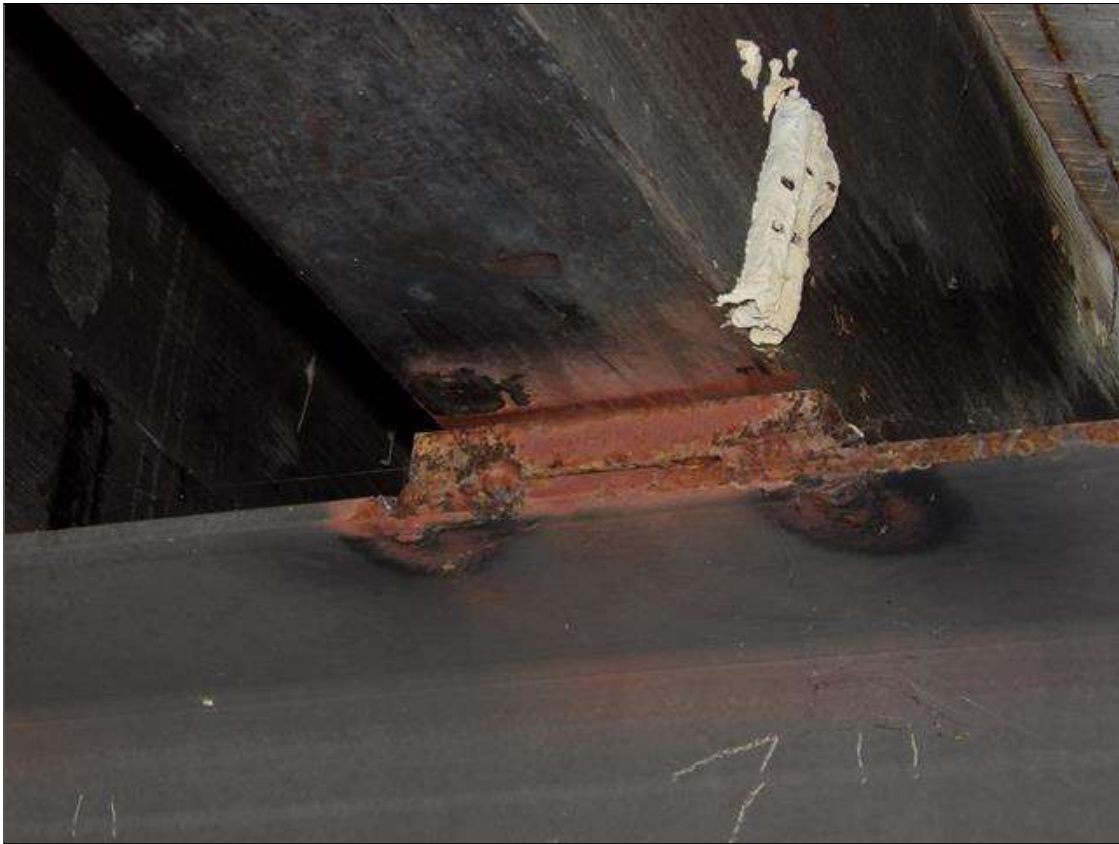
Typical bearing/shim plates under beams at crutch bent
