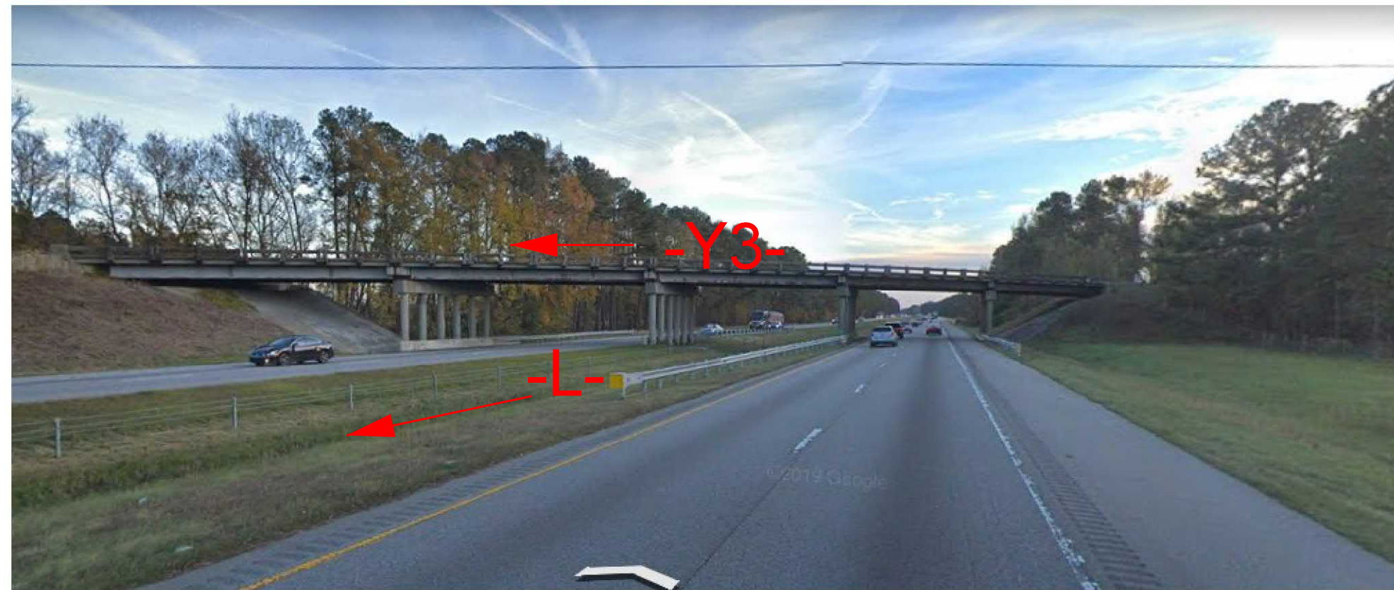
LOOKING SOUTH ON I-95 TOWARD PROPOSED BRIDGE NORTH OF EXISTING BRIDGE, EB2 (LEFT) EB1 (RIGHT)
