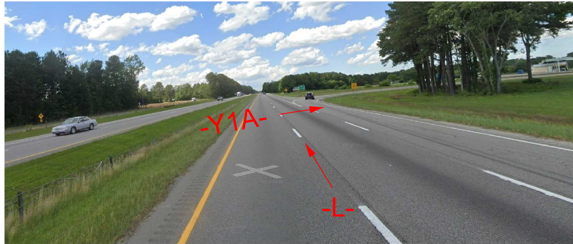
LOOKING NORTH ALONG -L- AT PROPOSED BRIDGE LOCATION
