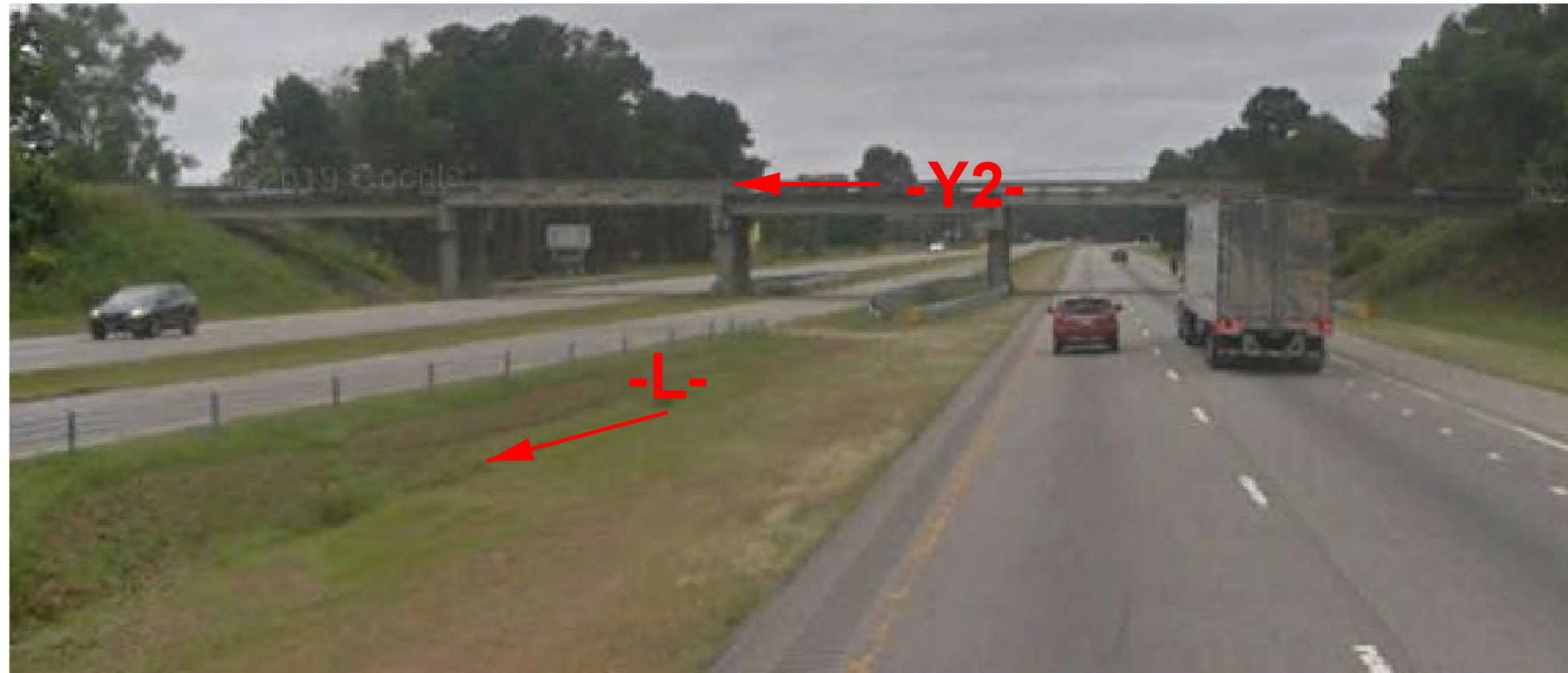
NORTH OF BRIDGE ON -L- LOOKING SOUTH FROM EB2 (LEFT) TOWARD EB1 (RIGHT)
