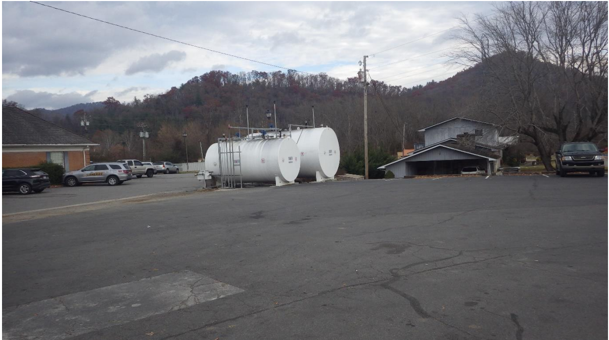
ASTs with concrete internal lining.
