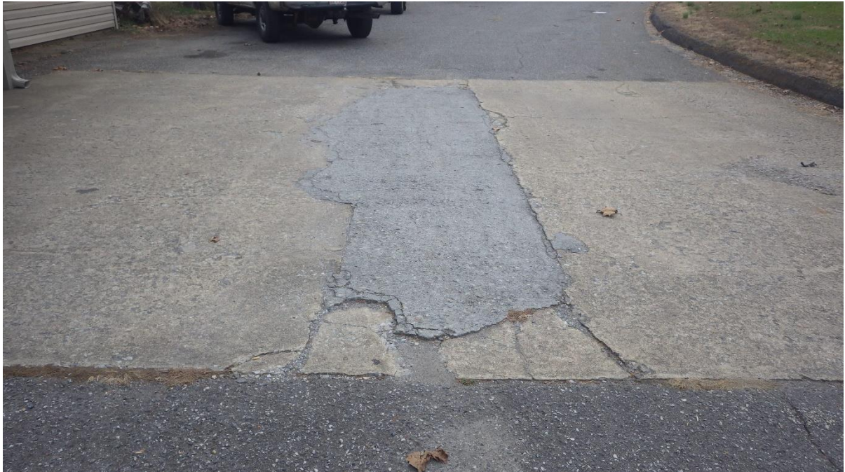
Former Pump island
