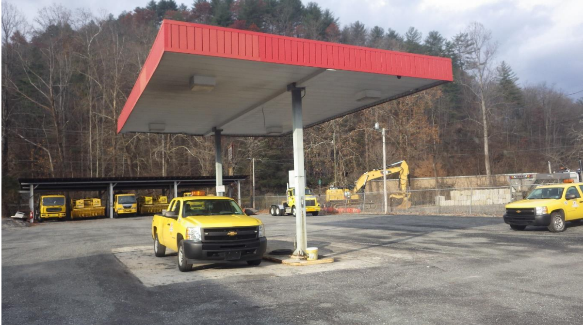
Former dispensers area
