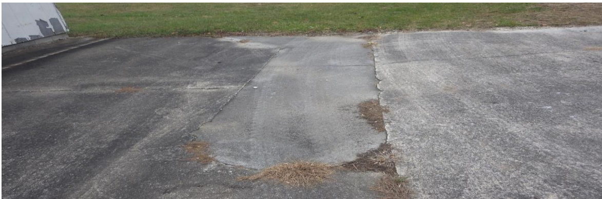
Pump island removed
