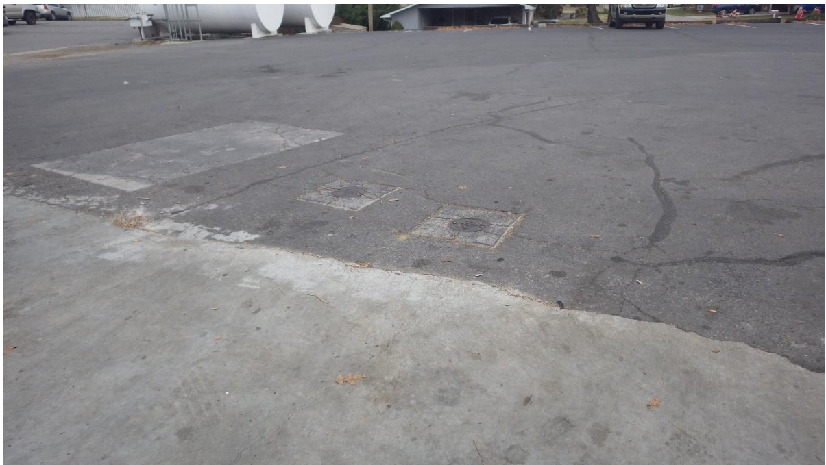
Monitoring wells in pairs.
