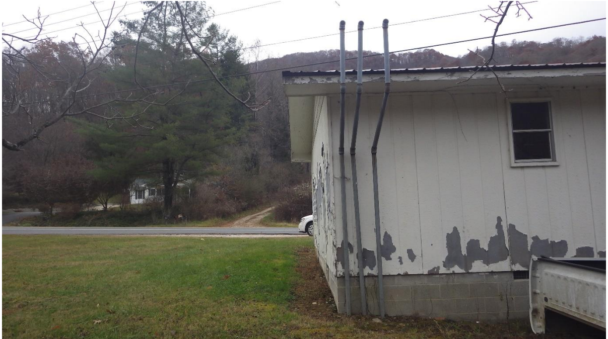
Three vent pipes on the back of the building
